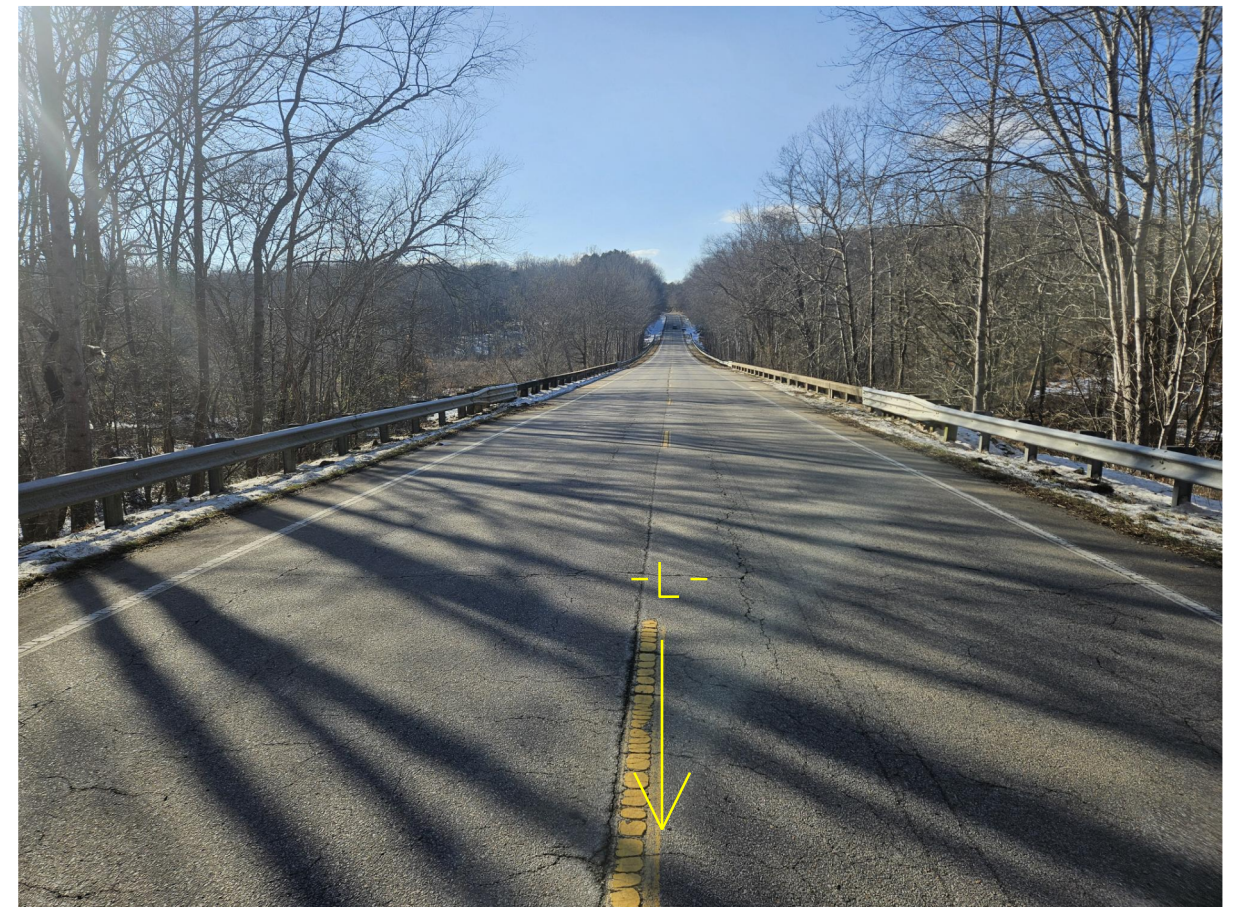
PHOTO #2: VIEW ALONG BRIDGE 163, FACING WEST, DOWNSTATION.
