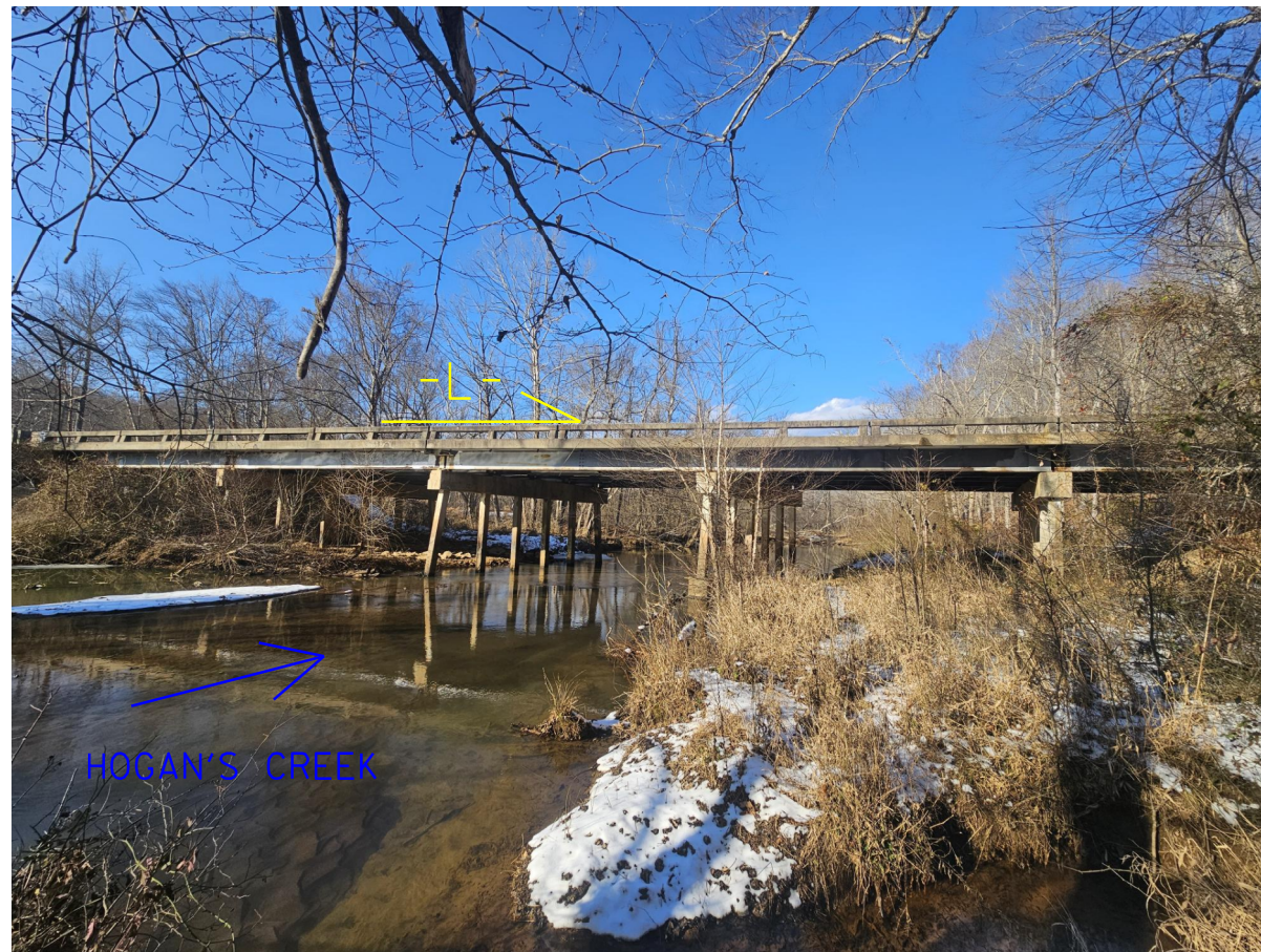
PHOTO #1: VIEW OF BRIDGE 163 PROFILE FACING NORTH.
