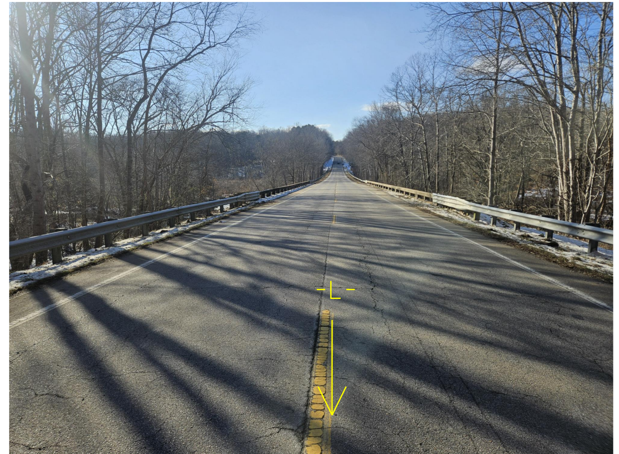
PHOTO #2: VIEW ALONG BRIDGE 163, FACING WEST, DOWNSTATION.
