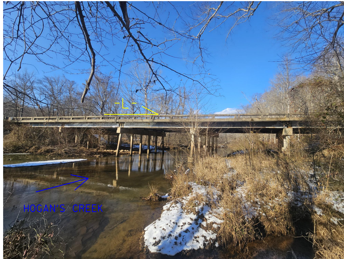
PHOTO #1: VIEW OF BRIDGE 163 PROFILE FACING NORTH.
