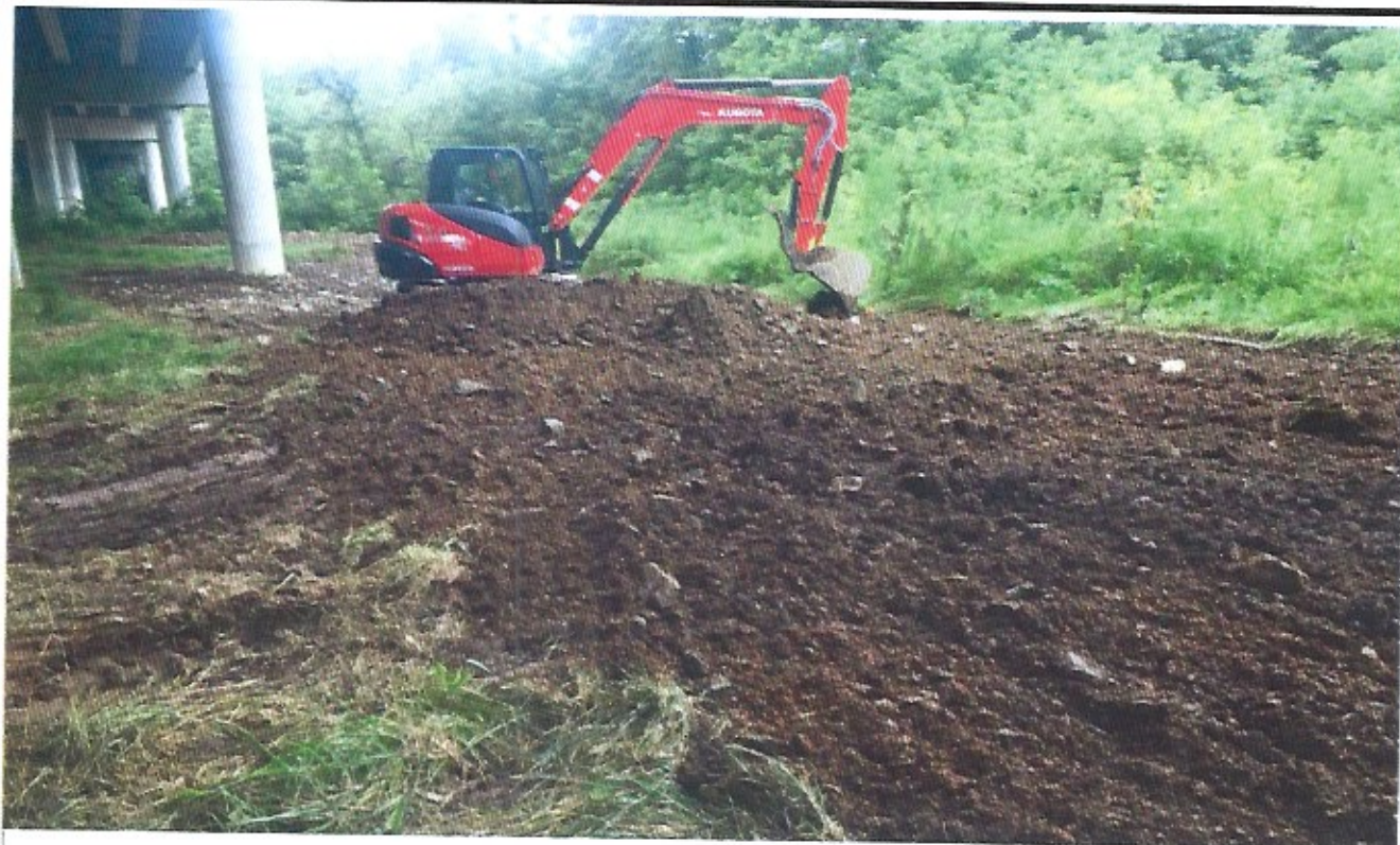
Excavation of contaminated soil
