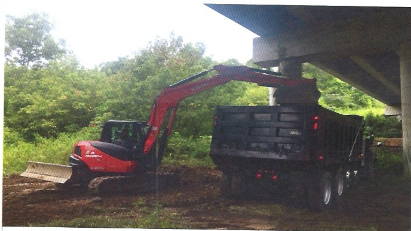
Loading of contaminated soil
