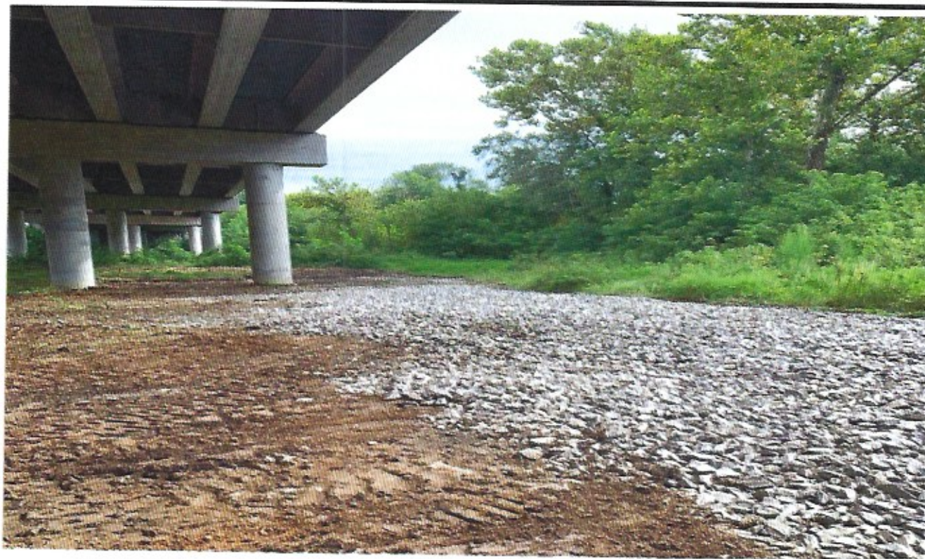
Placing stone over excavation
