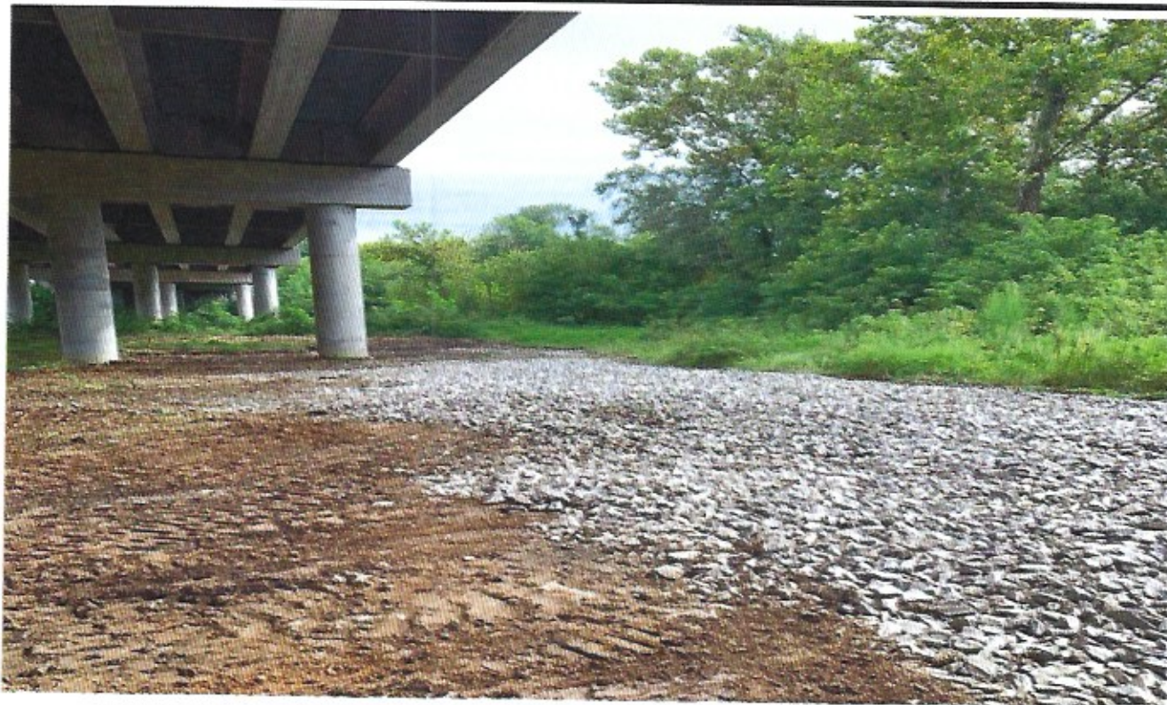
Placing stone over excavation
