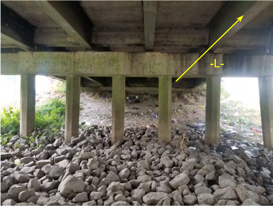
NEAR BENT 1 FACING WEST TO END BENT 1
