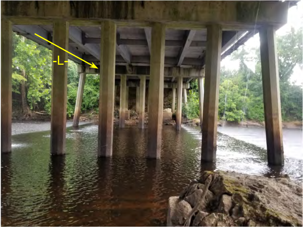
NEAR BENT 1 FACING EAST TO END BENT 2
