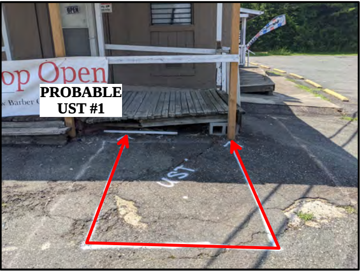
View of One Probable UST (Facing Approximately West)
