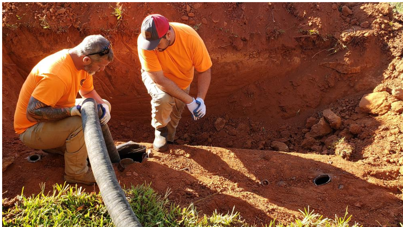
Photograph 5: Removal of Residual Liquids Using a Vacuum Truck
