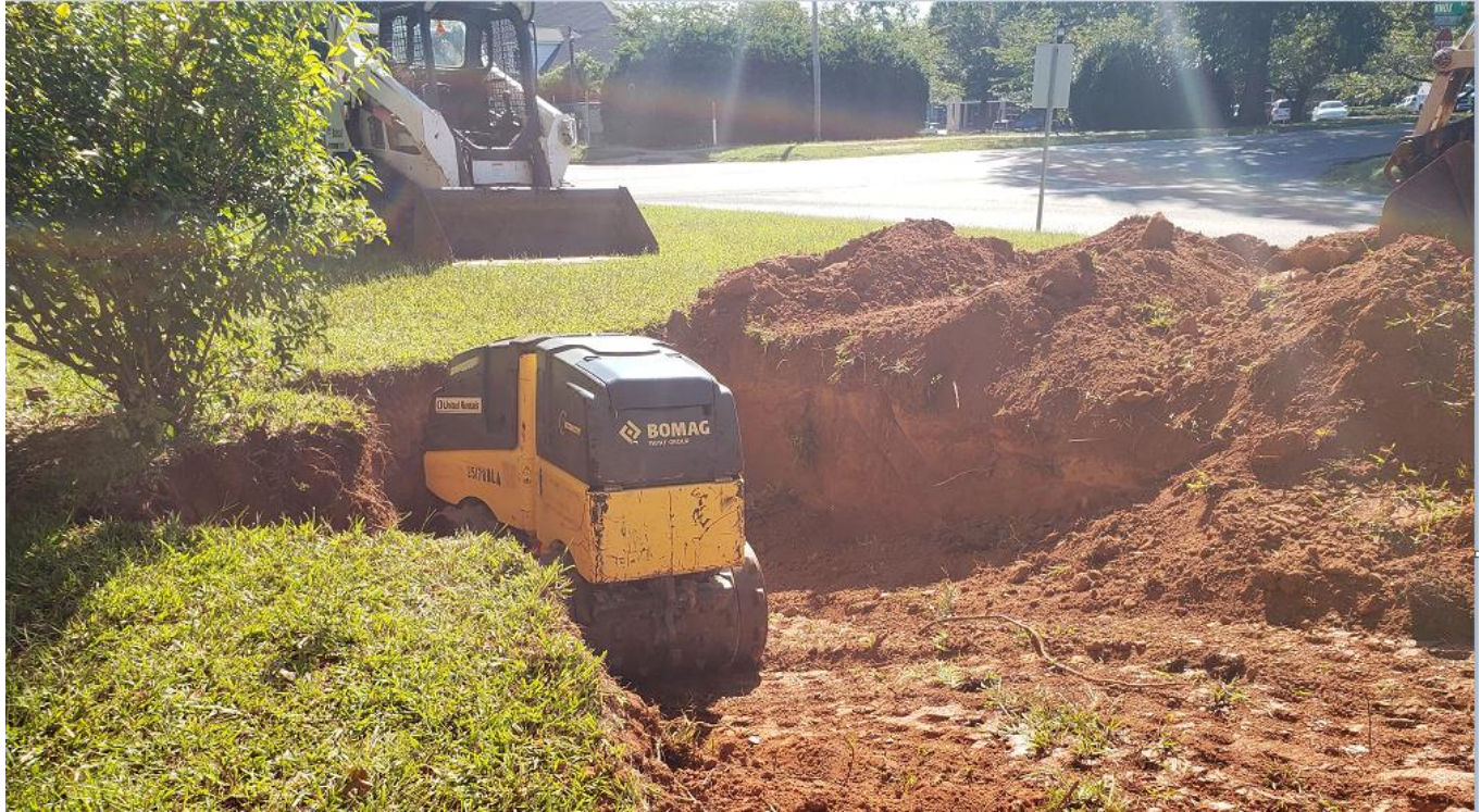
Photograph 9: Compaction of UST Excavation
