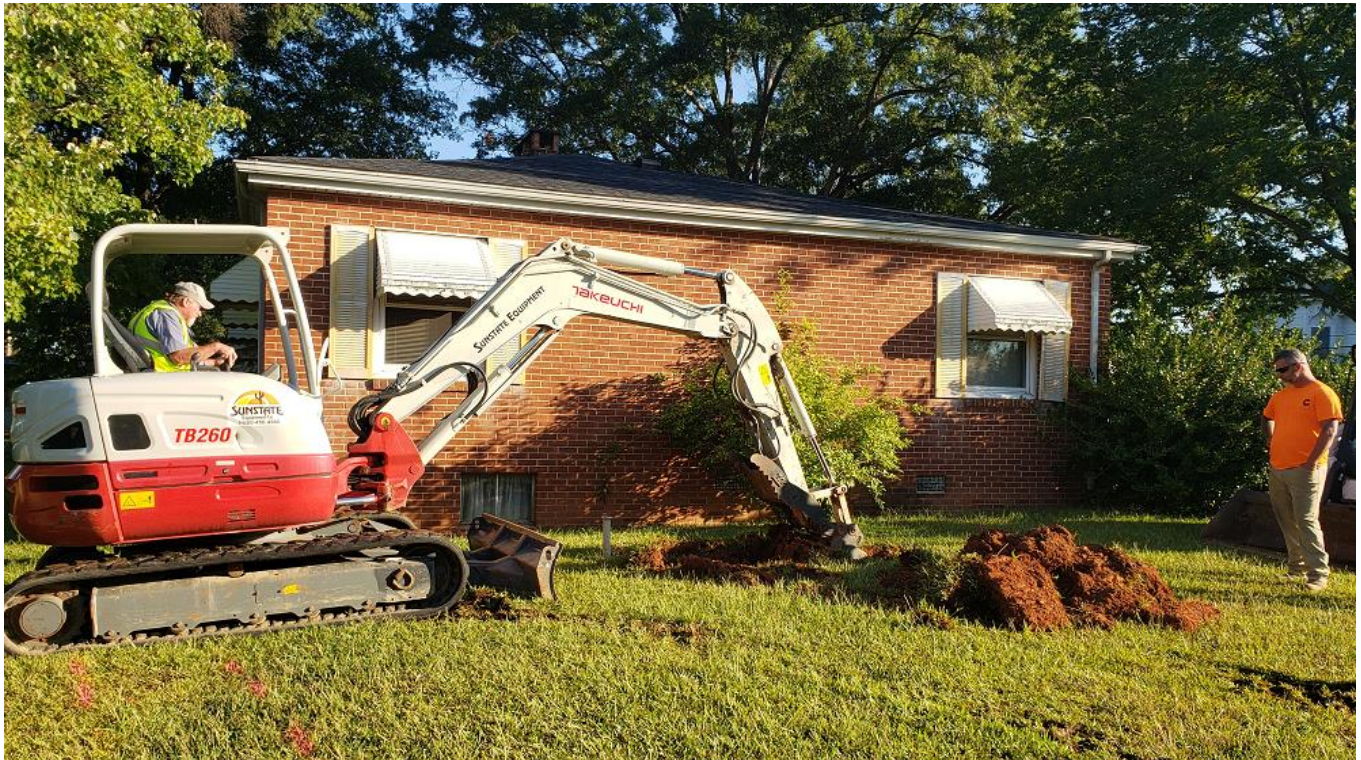
Photograph 3: Uncovering UST with Tracked Excavator
