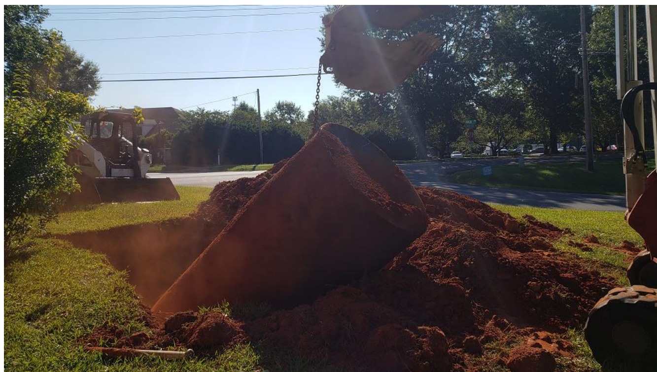
Photograph 6: Removal of UST from Excavation
