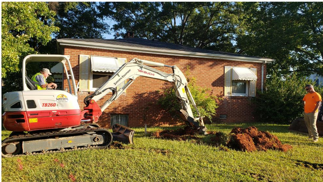
Photograph 3: Uncovering UST with Tracked Excavator
