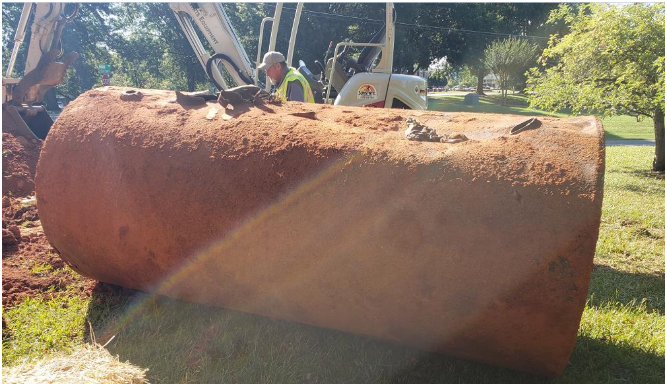
Photograph 7: UST Removed and Ready for Transportation Off-Site
