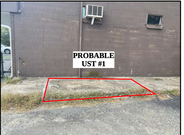
View of One Probable UST (Facing Approximately South)
