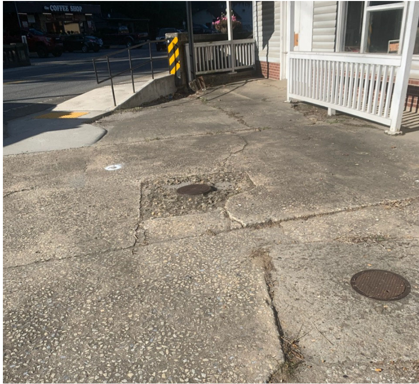
Photograph 1: View of potential fill ports near UST #1 and UST #2.
