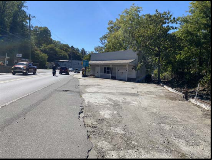
View of Survey Area (Facing Approximately West)
