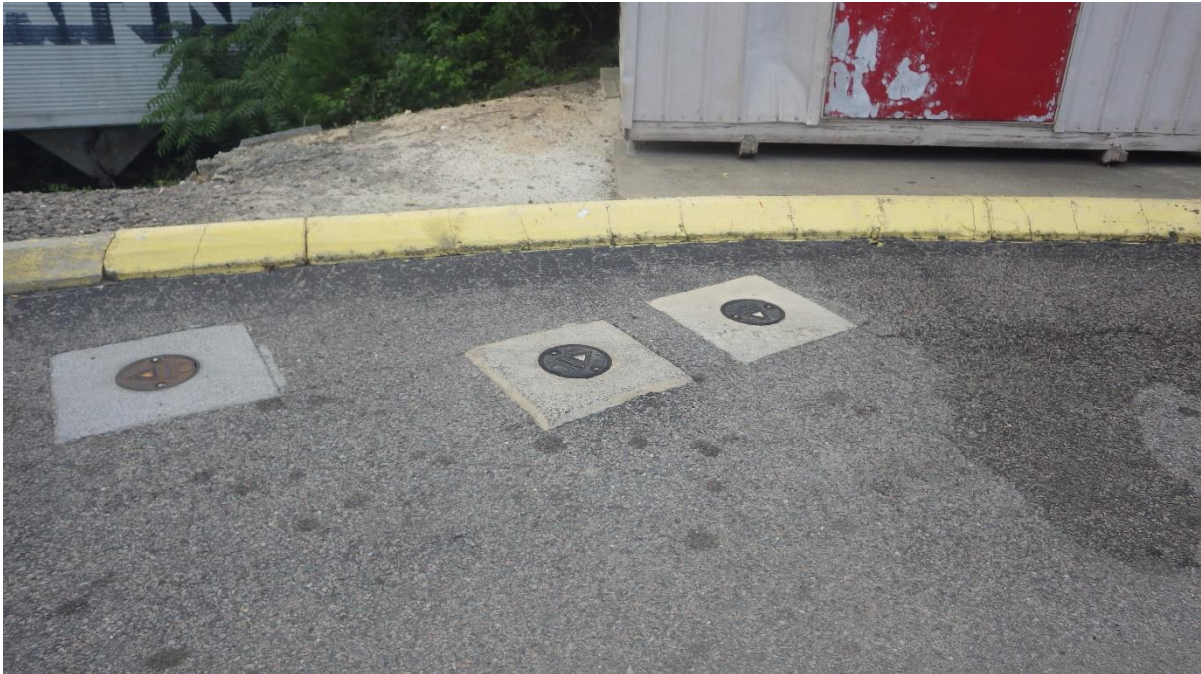
Clustered monitoring wells (Type III and Type II)
