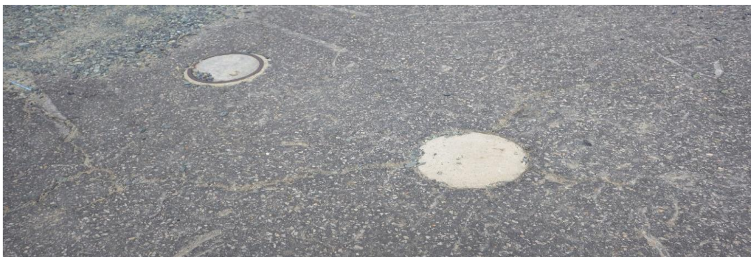
Abandoned monitoring well and testing hole.
