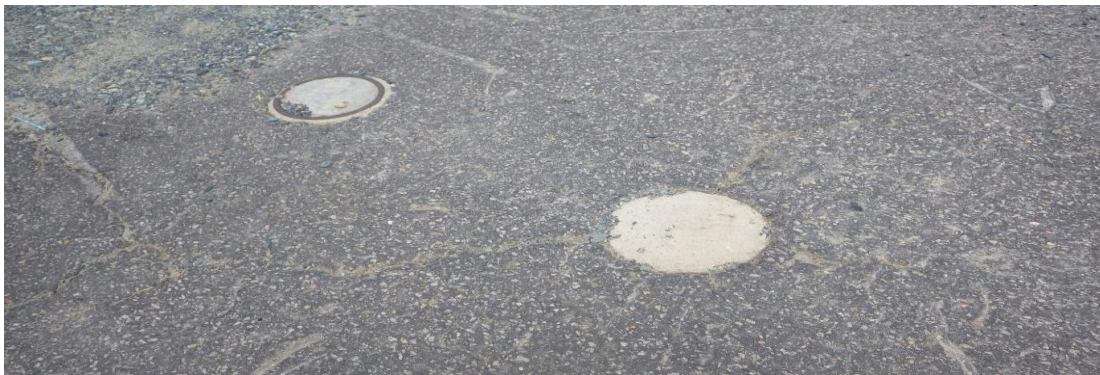
Abandoned monitoring well and testing hole.
