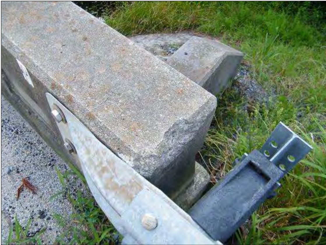
RIGHT RAIL SPALLED AT END BENT 1.
