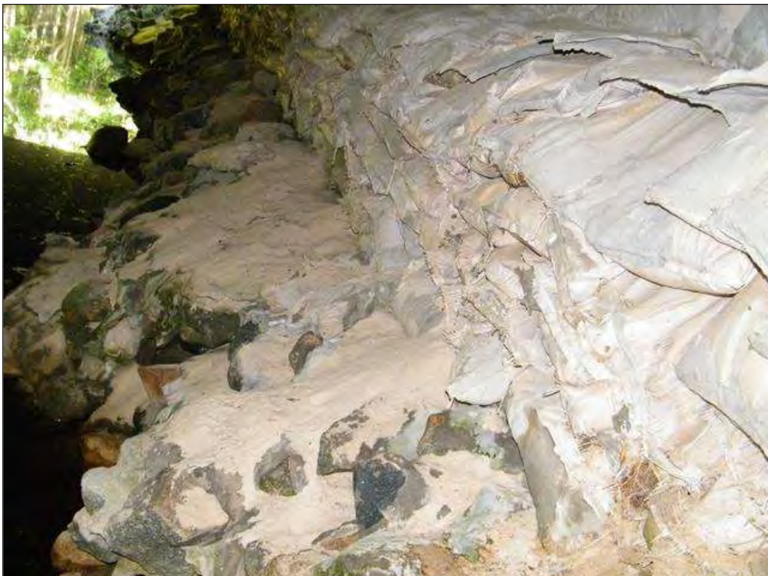
SAND BAGS AND GROUT AT END BENT 1.
