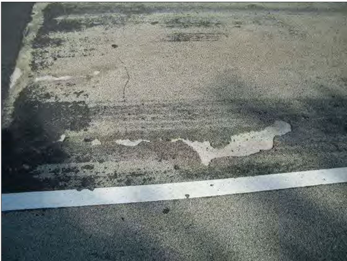
WEARING SURFACE MISSING IN AREAS IN SPAN 1, NORTHBOUND LANE.
