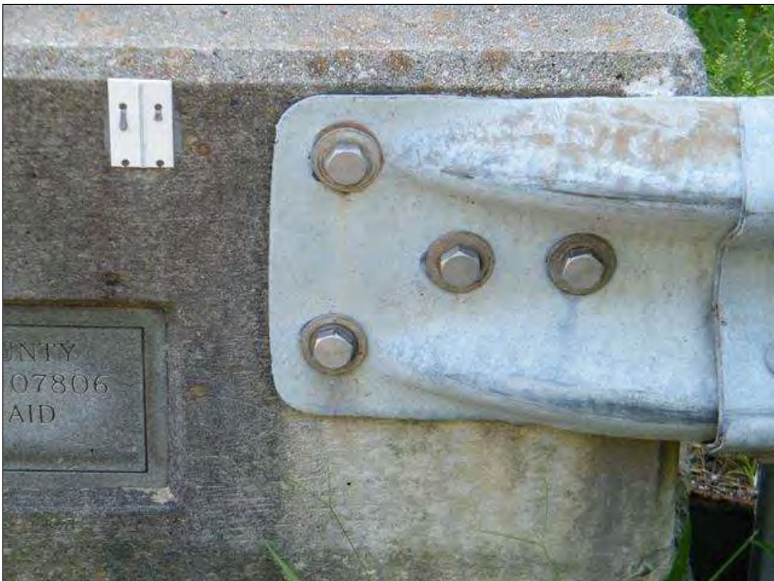
GUARDRAIL ATTACHMENT
