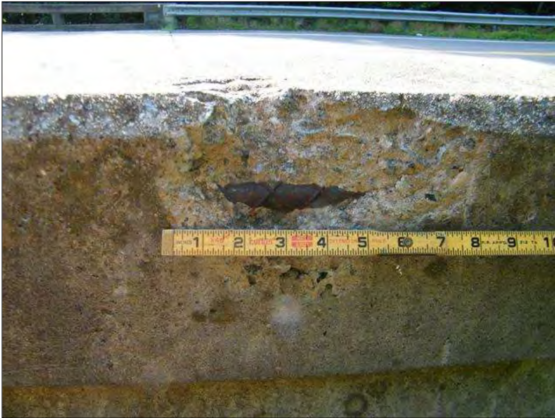
CRACKED, SPALLED, AND DELAMINATED AREA WITH RESTEEL EXPOSED IN EXTERIOR OF LEFT RAIL AT END BENT 1.
