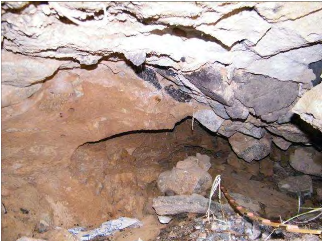
INTERIOR VIEW OF VOID ON LEFT SIDE AT END BENT 2. AREA IS GREATER THAN 6' WIDE AND 1' TALL. PRIORITY MAINTENANCE ISSUED.
