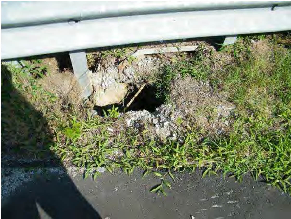
TOP VIEW OF VOID ON LEFT SIDE AT END BENT 2. AREA IS GREATER THAN 6' WIDE, 1' TALL, AND IS LOCATED 18" FROM PAVEMENT.
