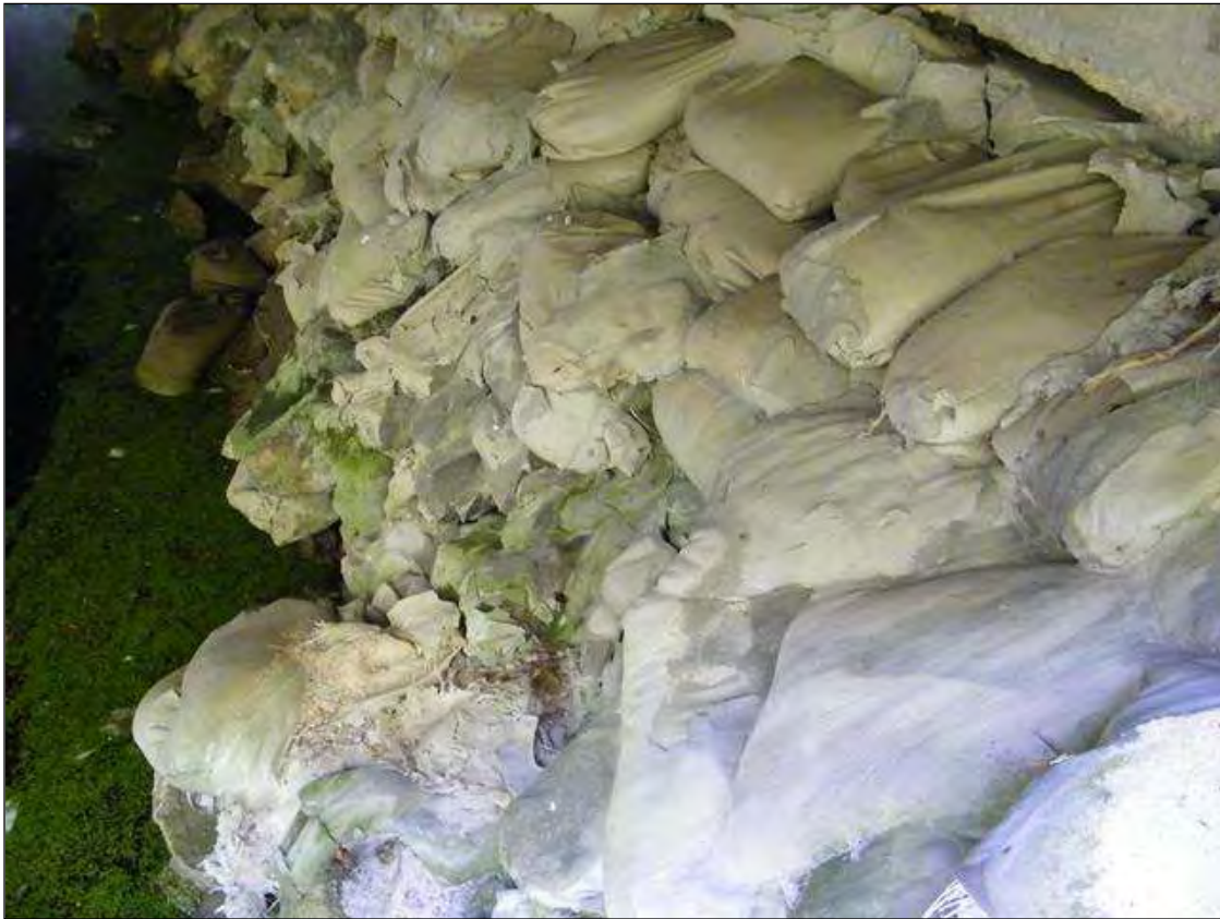
GROUT AND SAND BAGS AT ENDBENTS.
