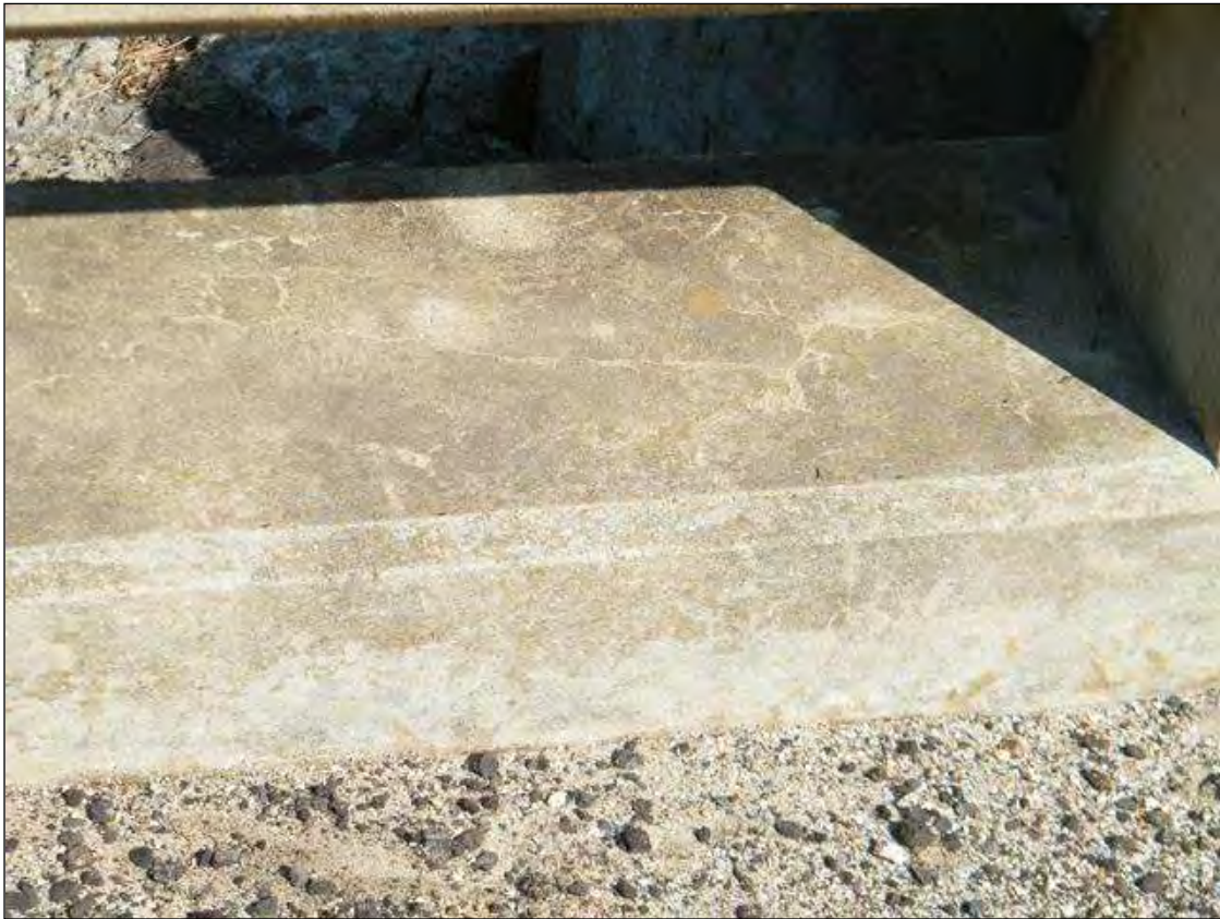
MAP CRACKING WITH EFFLO IN CURBS.
