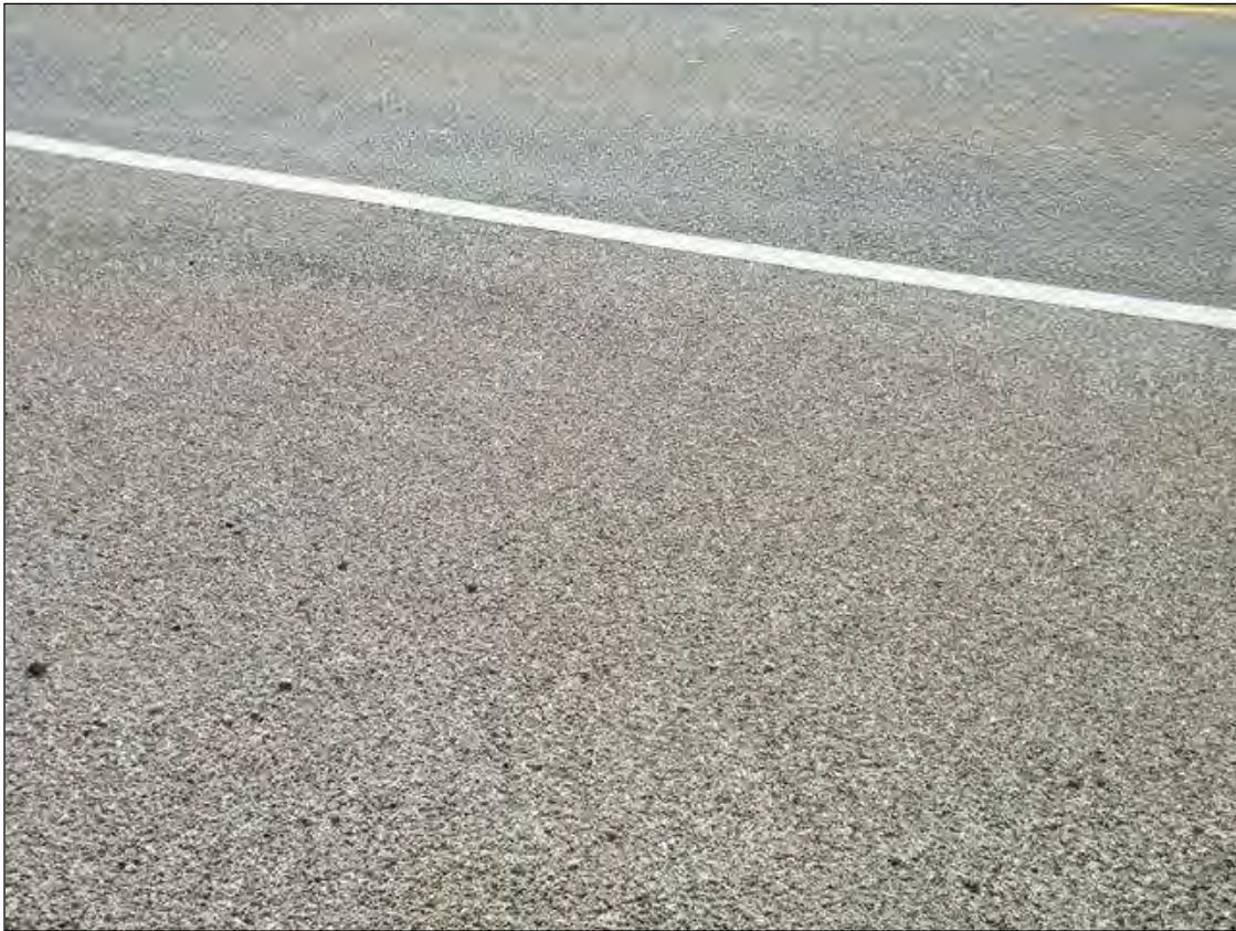
0.010' EPOXY WEARING SURFACE ADDED.
