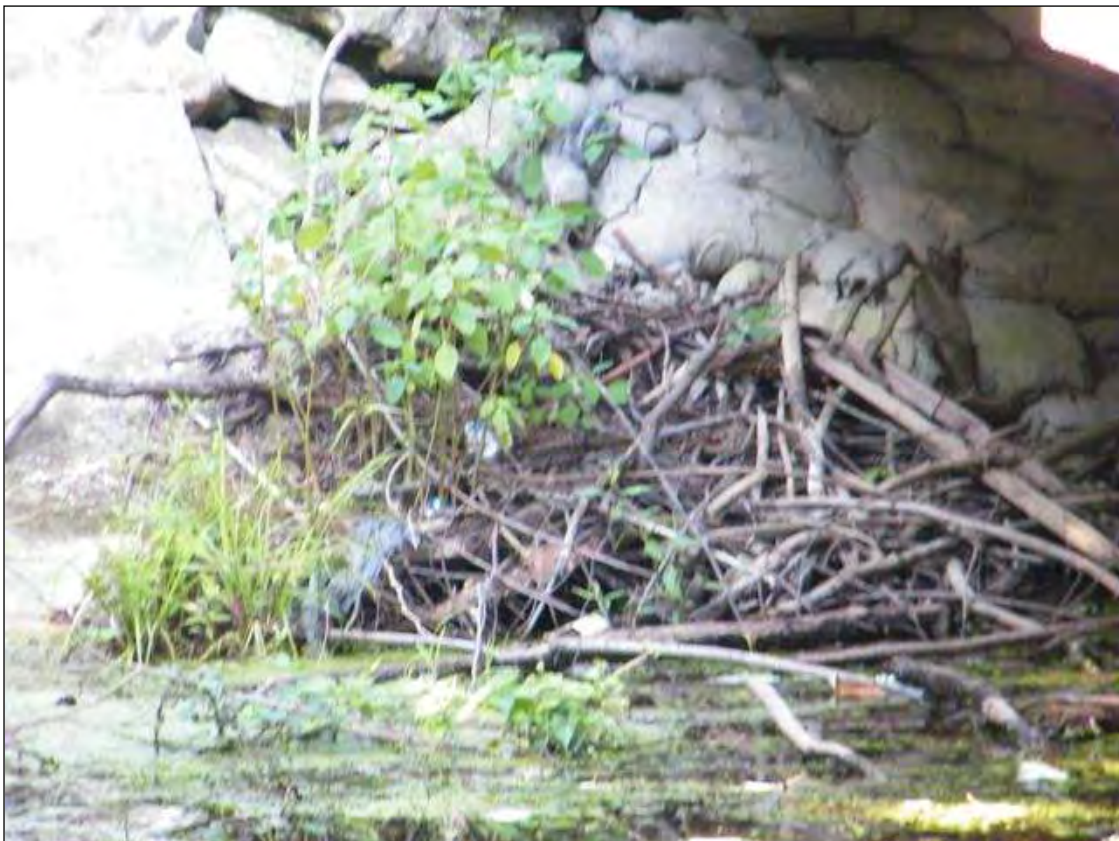
DRIFT AT END BENT 1 ON RIGHT SIDE.
