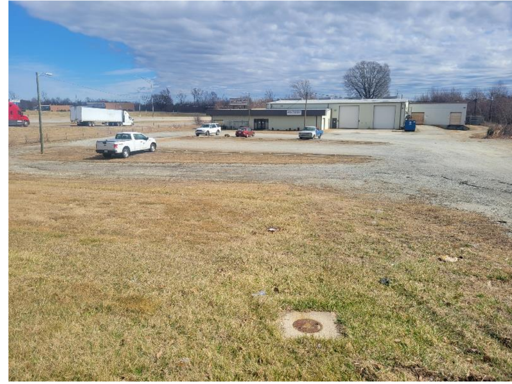
B. Photograph from west side of parcel, facing east with MW-14 in foreground.
