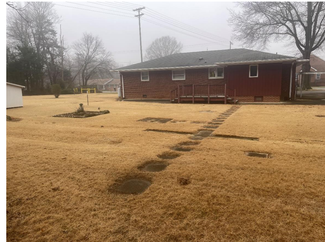
B. Photograph of east side of site and rear of house, facing west. The former heating oil UST is reportedly located outside the kitchen widow beneath the deck.
