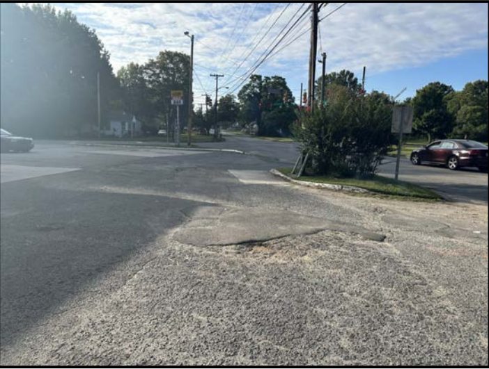
View of Survey Area (Facing Approximately South)
