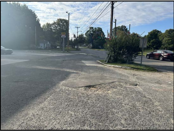
View of Survey Area (Facing Approximately South)
