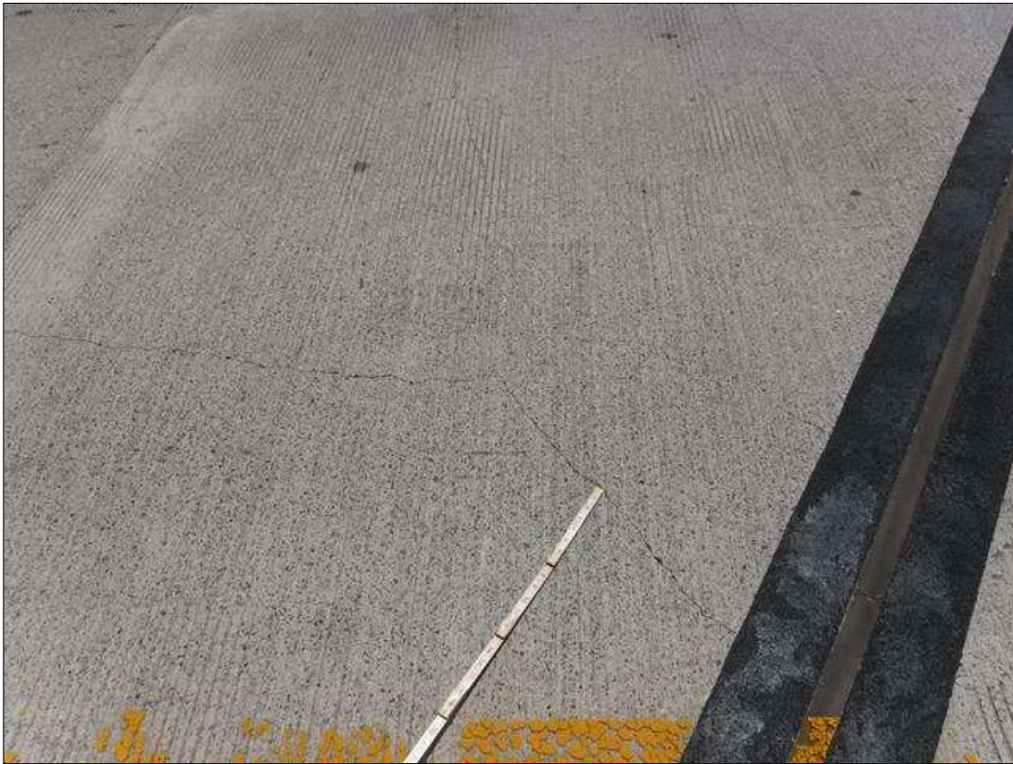
Span 3 Wearing Surface: UP TO 1/16" DIAGONAL, LONGITUDINAL AND TRANSVERSE CRACKS IN VARIOUS LOCATIONS, CRACKS IN INSIDE EASTBOUND LANE AT BENT 3 JOINT SHOWN
