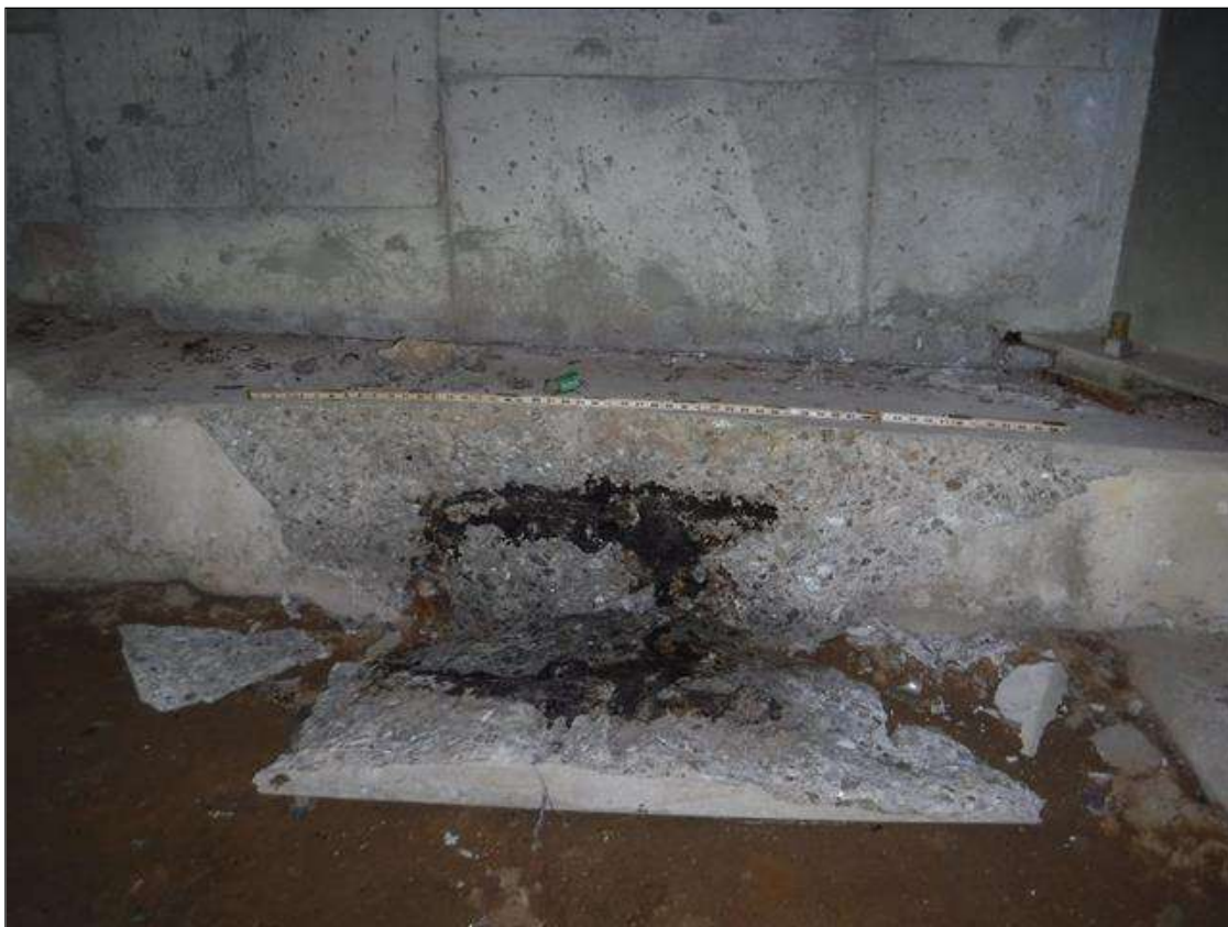
End Bent 2 Cap 1: PAR: 60" X 15" X 3" SPALL WITH EXPOSED REBAR IN TOP AND FACE OF CAP BENEATH BAY
