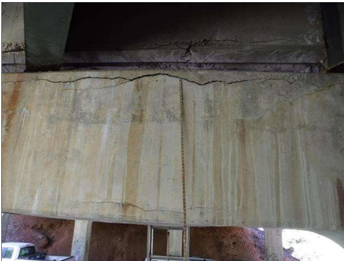
Bent 1 Cap 1: PAR: UP TO 8' X 30" X 3" DEEP SPALLS WITH EXPOSED REBAR, 13' X 6" AREAS OF DELAMINATION AND UP TO 1/2" DIAGONAL AND HORIZONTAL CRACKS IN BOTTOM AND BOTH FACES OF CAP BENEATH BAY 2, CONDITION IN SPAN 1 FACE SHOWN
