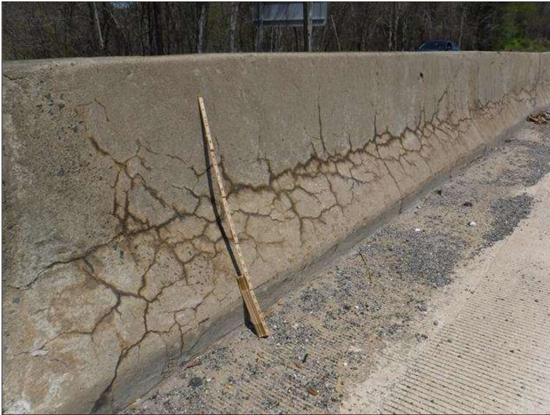
Span 3 Median Bridge Rail: UP TO 1/16" HORIZONTAL AND MAP CRACKING THROUGHOUT BOTH FACES OF RAIL, CRACKS IN RIGHT FACE NEAR MIDSPAN SHOWN
