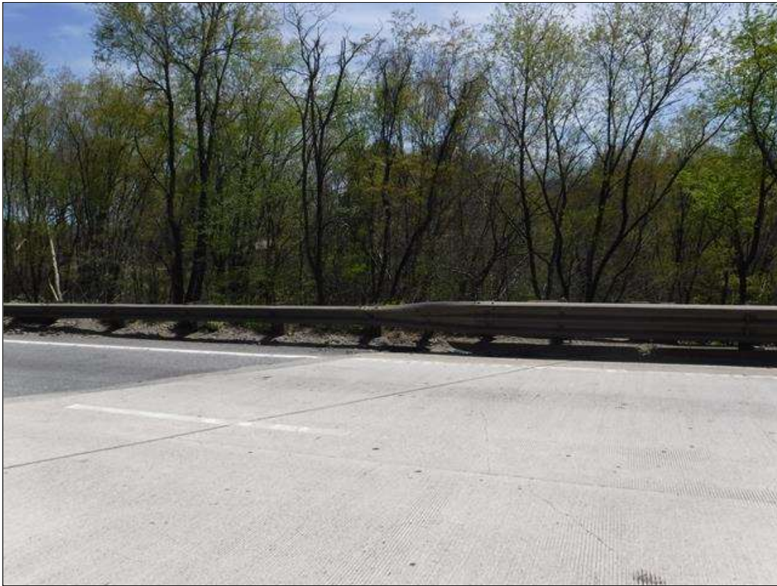
GUARDRAIL TO BARRIER RAIL TRANSITION AT SOUTHEAST CORNER, NORTHEAST AND SOUTHWEST CORNERS SIMILAR
