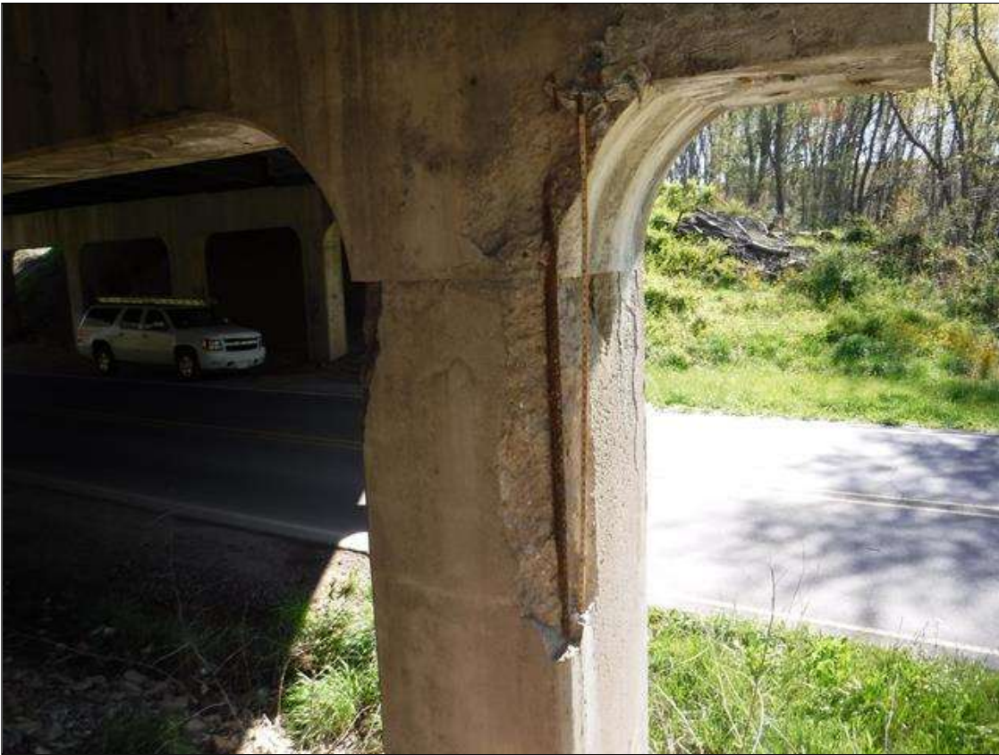
Bent 1 Pile 5: PAR: (3) SPALLS WITH EXPOSED REBAR UP TO 60" X 10" X 10" IN NORTHWEST CORNER, SOUTHWEST CORNER AND RIGHT FACE OF COLUMN EXTENDING FROM BOTTOM OF CAP
