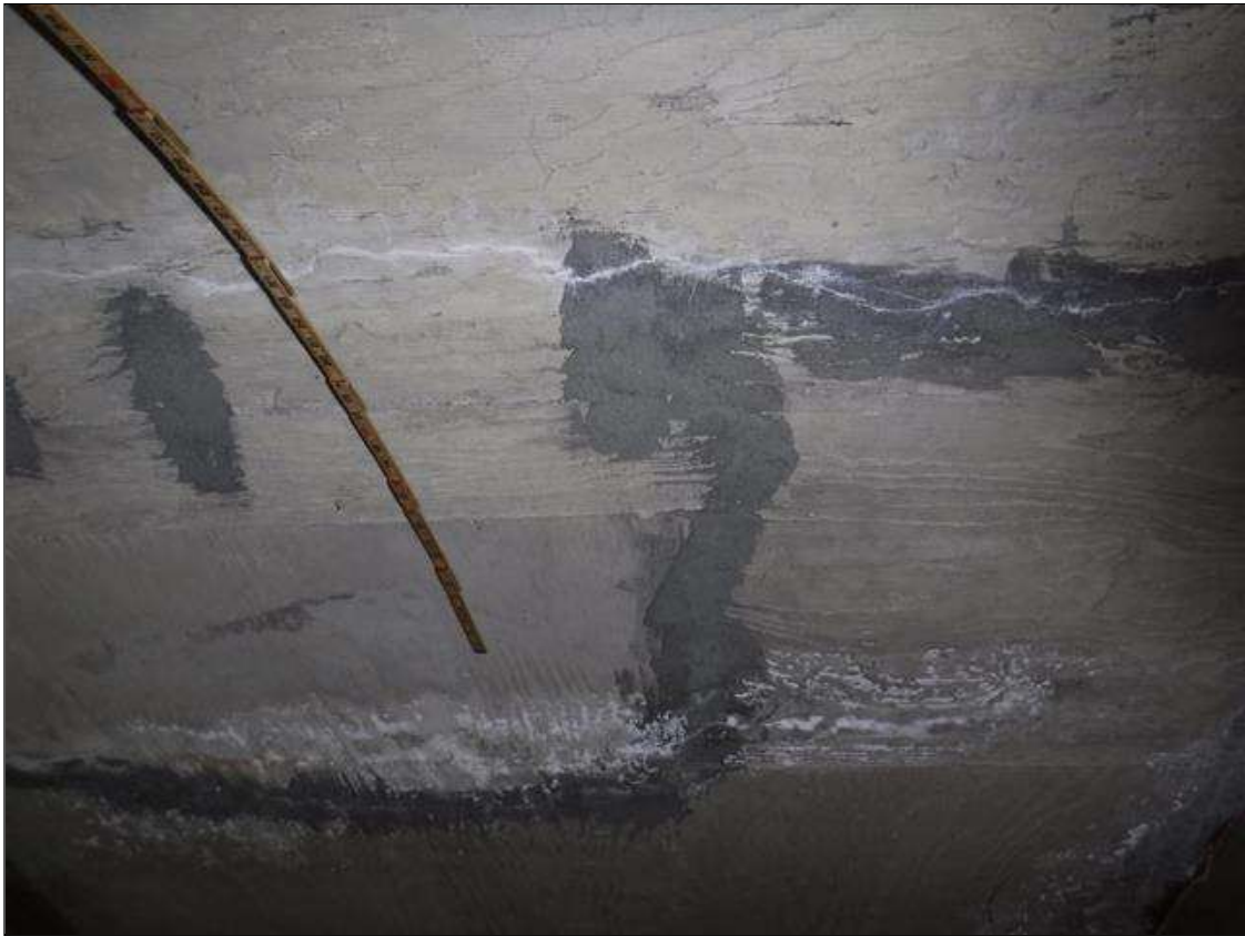
Span 1 Deck: UP TO 0.016" TRANSVERSE CRACKS WITH EFFLORESCENCE AND FAILED SEALED CRACKS IN BOTTOM OF DECK IN BAY 1, CONDITION APPROXIMATELY 6' FROM END BENT 1 SHOWN
