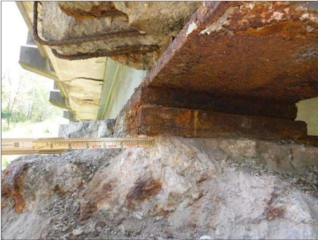
Span 2 Beam 10 Near Bearing: LESS THAN 1% LOSS OF BEARING AREA BENEATH BEAM 10 BEARING
