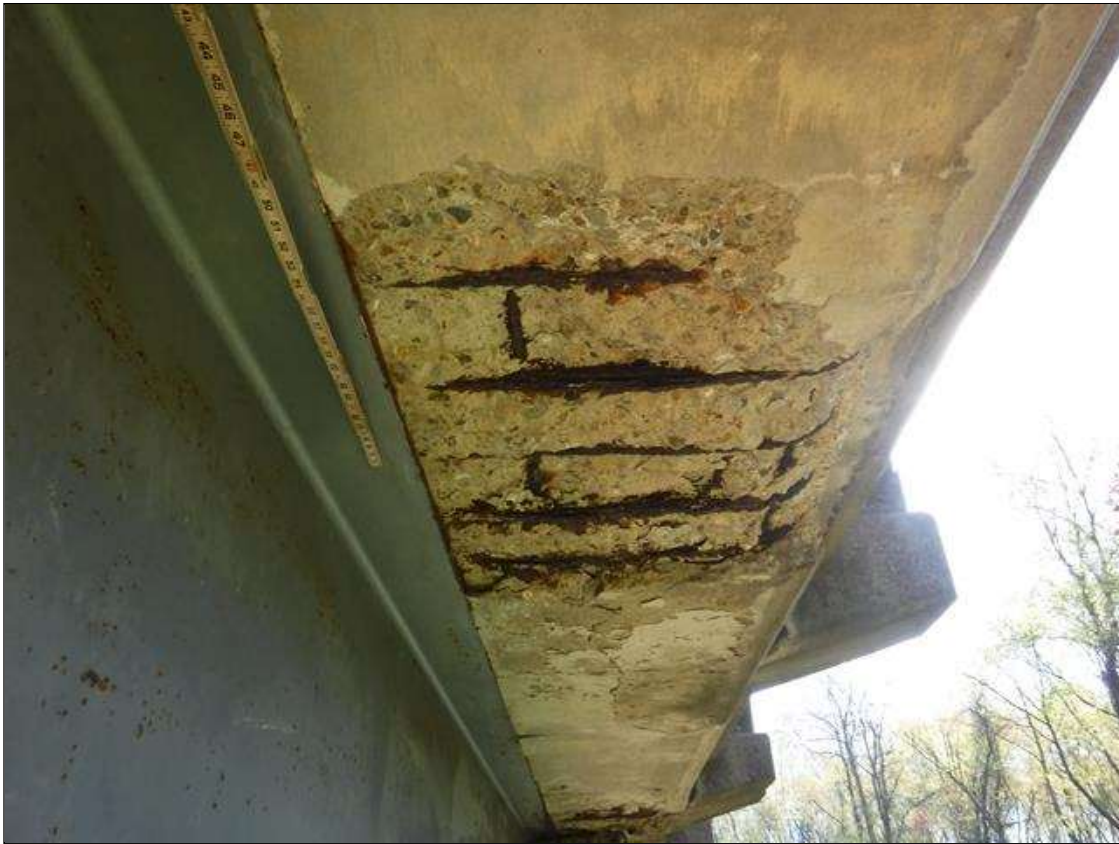
Span 1 Deck: PAR: (6) SPALLS WITH EXPOSED LONGITUDINAL AND TRANSVERSE REBAR UP TO 48" X 24" X 3" DEEP AND AREAS OF DELAMINATION UP TO 60" X 24" ALONG RIGHT OVERHANG, CONDITION APPROXIMATELY 15' FROM BENT 1 SHOWN
