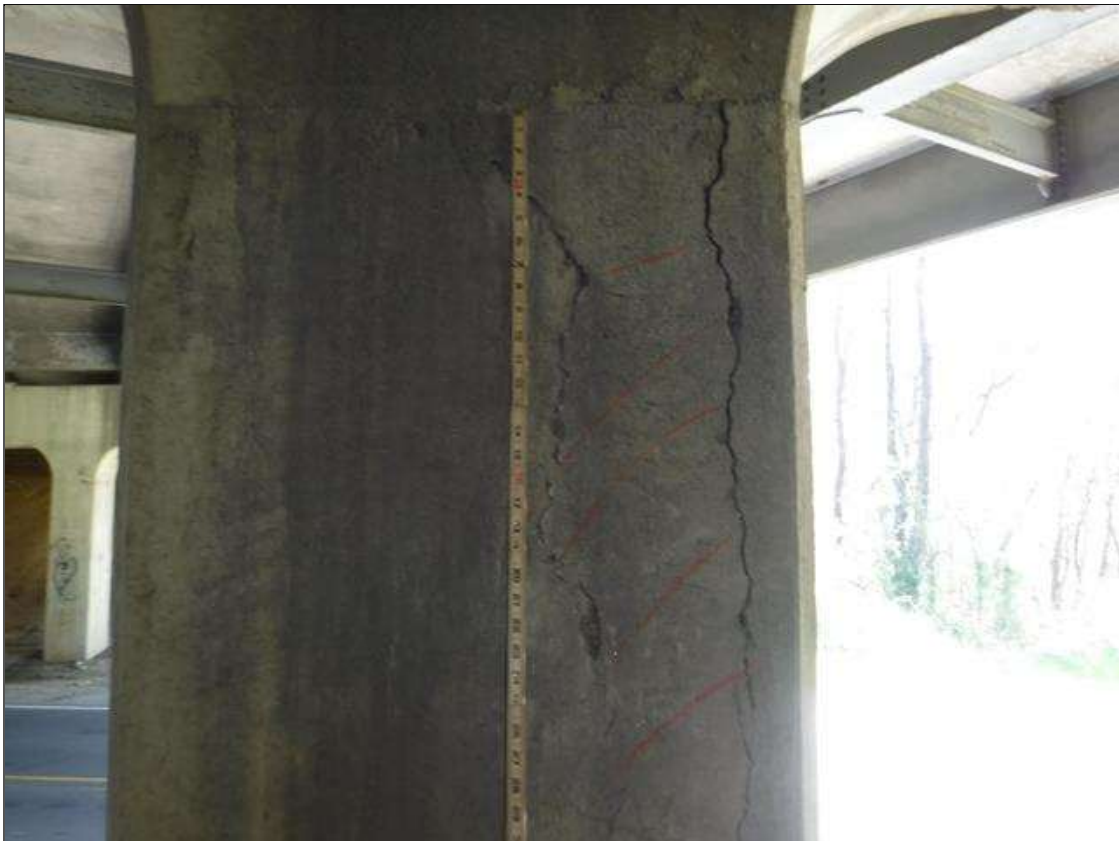
Bent 1 Pile 4: 52" X 8" AREA OF DELAMINATION WITH UP TO 1/4" VERTICAL CRACKS IN SPAN 1 FACE OF COLUMN EXTENDING FROM BOTTOM OF CAP
