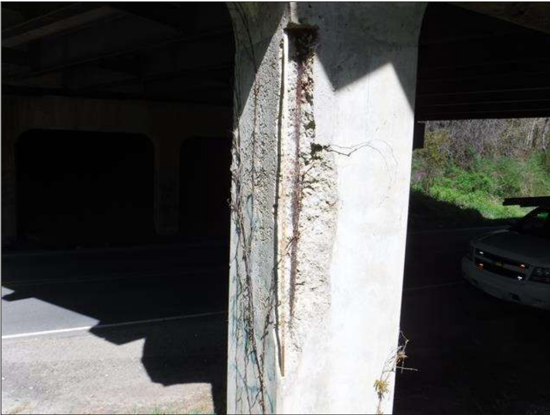
Bent 2 Pile 5: PAR: 66" X 13" X 6" SPALL WITH EXPOSED REBAR IN SOUTHEAST CORNER OF COLUMN EXTENDING FROM BOTTOM OF CAP
