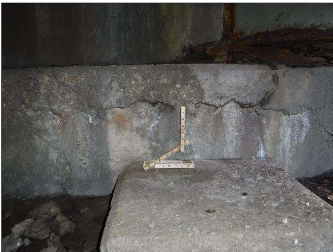
End Bent 1 Cap 1: UP TO 1/4" TRANSVERSE AND VERTICAL CRACKS WITH AND WITHOUT EFFLORESCENCE IN FACE OF CAP BENEATH BAY 1
