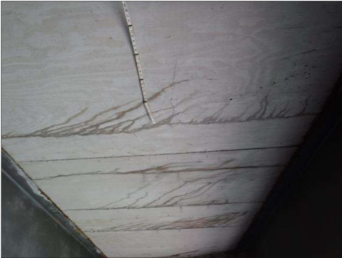
Span 1 Deck: 20' X 78" FAILED PATCH WITH UP TO 0.02" LONGITUDINAL AND TRANSVERSE CRACKS WITH EFFLORESCENCE IN BOTTOM OF DECK IN BAY 8, EXTENDING FROM BENT 1, CONDITION APPROXIMATELY 15' FROM BENT 1 SHOWN
