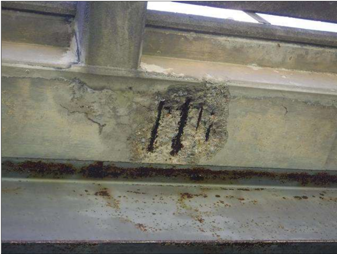
Span 2 Deck: PAR: 26" X 24" X 2" DEEP SPALL WITH EXPOSED REBAR IN BOTTOM OF LEFT OVERHANG, APPROXIMATELY 6' FROM BENT 1
