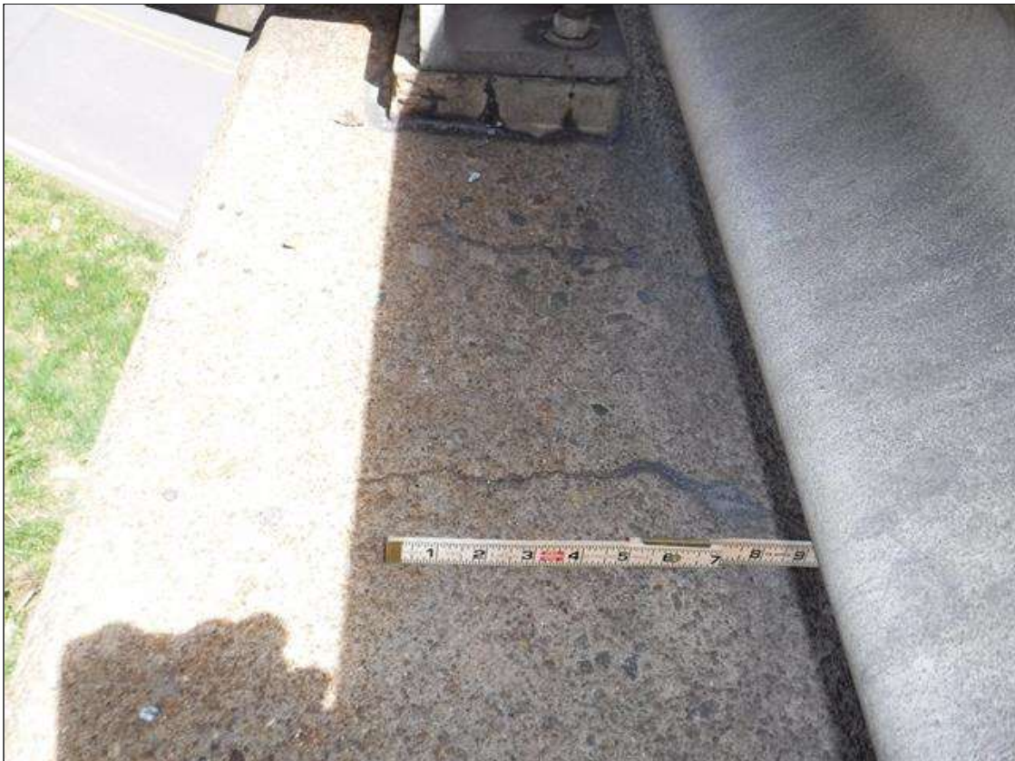
UP TO 0.05" TRANSVERSE AND VERTICAL CRACKS IN TOP AND FACE OF CURBS IN VARIOUS LOCATIONS, CRACK IN SPAN 1 LEFT CURB APPROXIMATELY 5' FROM BENT 1 JOINT SHOWN
