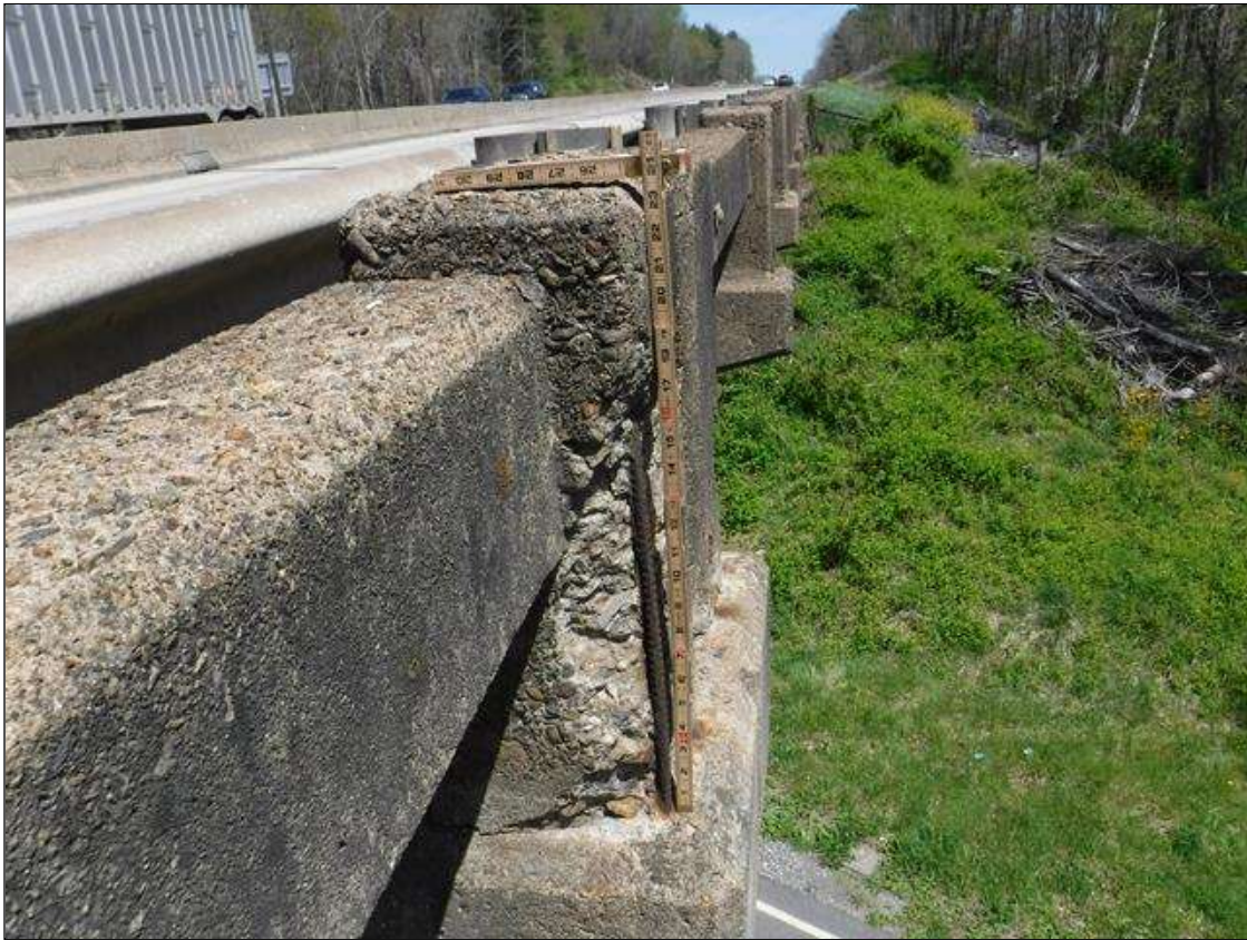
Span 2 Right Bridge Rail: SPALLS WITH EXPOSED REBAR UP TO 17" X 4" X 4" DEEP IN BACK FACE AND BOTTOM OF RAIL AND POSTS IN VARIOUS LOCATIONS, CONDITION NEAR MIDSPAN SHOWN
