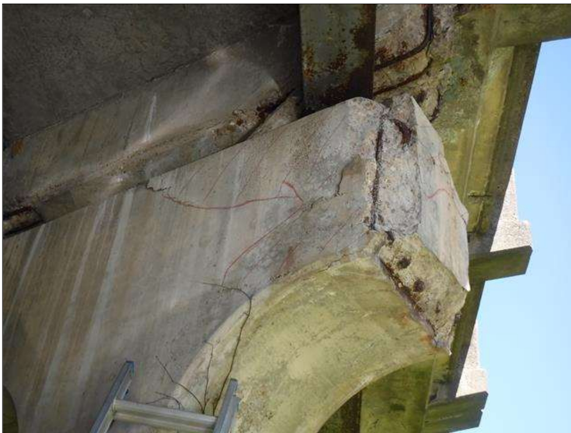
Bent 2 Cap 1: PAR: 103" X 33" X 30" AREA OF DELAMINATION WITH UP TO 1/2" VERTICAL AND HORIZONTAL CRACKS AND 33" X 30" X 5" DEEP SPALL WITH EXPOSED REBAR THROUGHOUT CAP EXTERIOR FROM RIGHT END TO BENEATH BAY 9, CONDITION IN SPAN 3 FACE SHOWN
