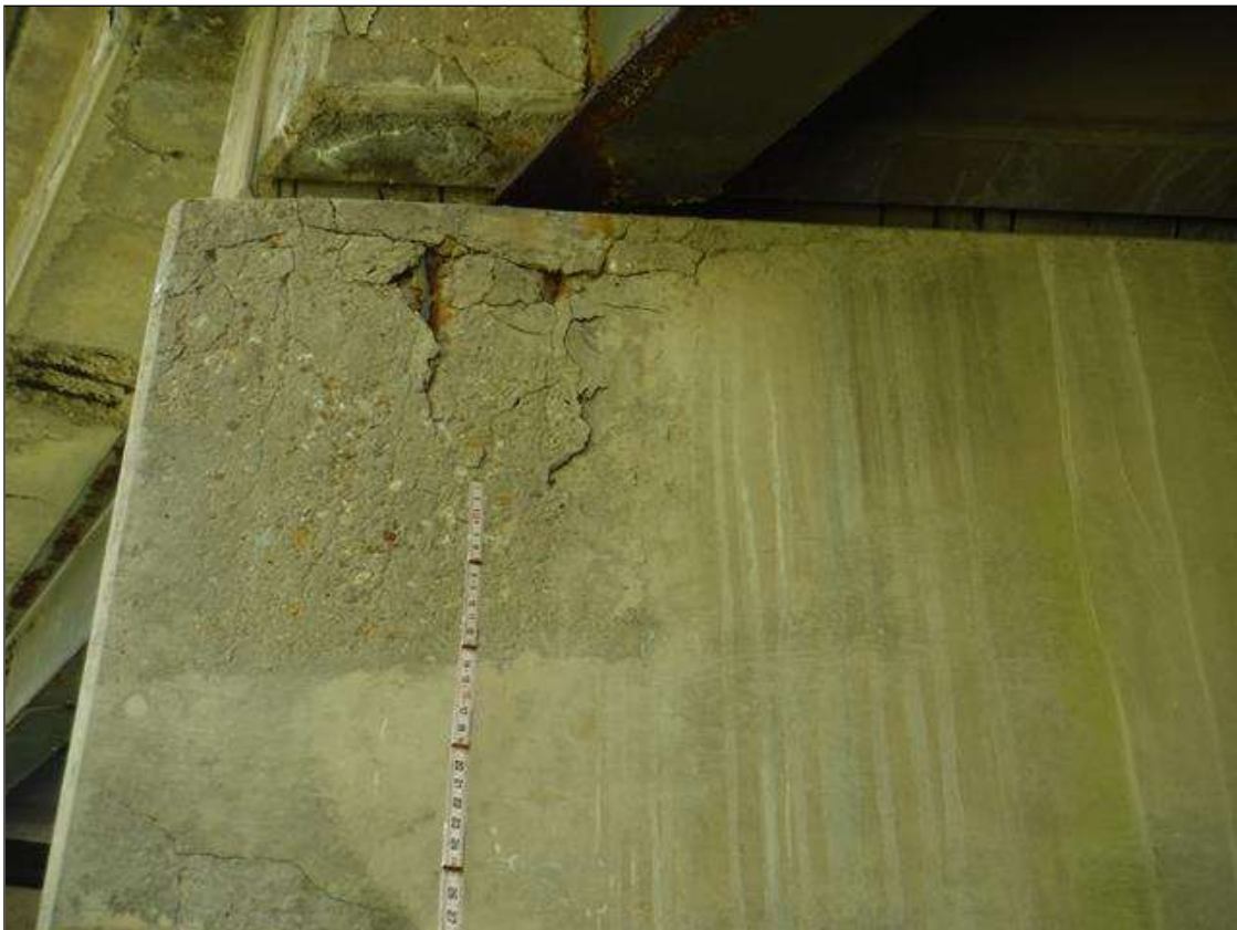
Bent 1 Cap 1: (2) SPALLS WITH EXPOSED REBAR UP TO 7" X 3" X 1" DEEP WITH 32" X 32" AREA OF DELAMINATION AND UP TO 1/8" MAP CRACKING IN SPAN 1 FACE OF CAP AT LEFT END
