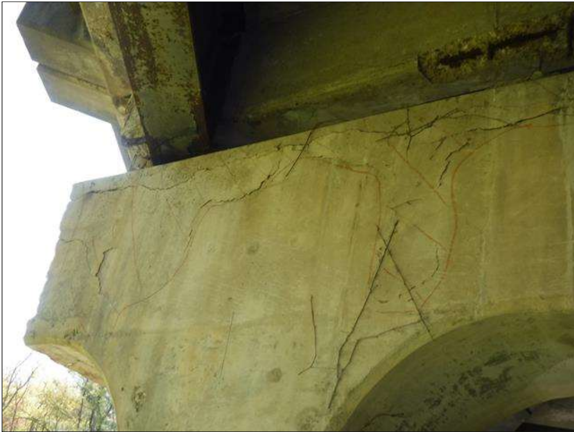
Bent 2 Cap 1: PAR: 103" X 33" X 30" AREA OF DELAMINATION WITH UP TO 1/2" VERTICAL AND HORIZONTAL CRACKS AND 33" X 30" X 5" DEEP SPALL WITH EXPOSED REBAR THROUGHOUT CAP EXTERIOR FROM RIGHT END TO BENEATH BAY 9, CONDITION IN SPAN 2 SHOWN
