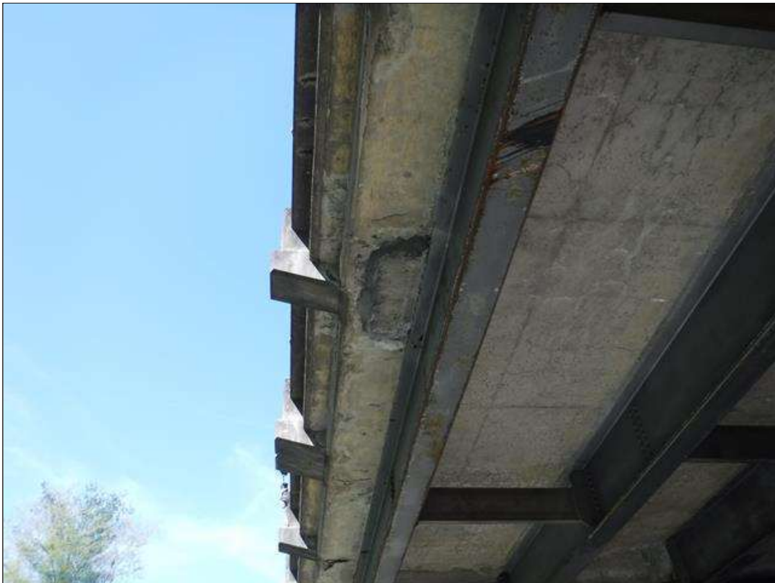
Span 2 Deck: PAR: FAILED REPAIR AND (2) AREAS OF DELAMINATION UP TO 36" X 22" IN BOTTOM OF RIGHT OVERHANG ABOVE ROADWAY
