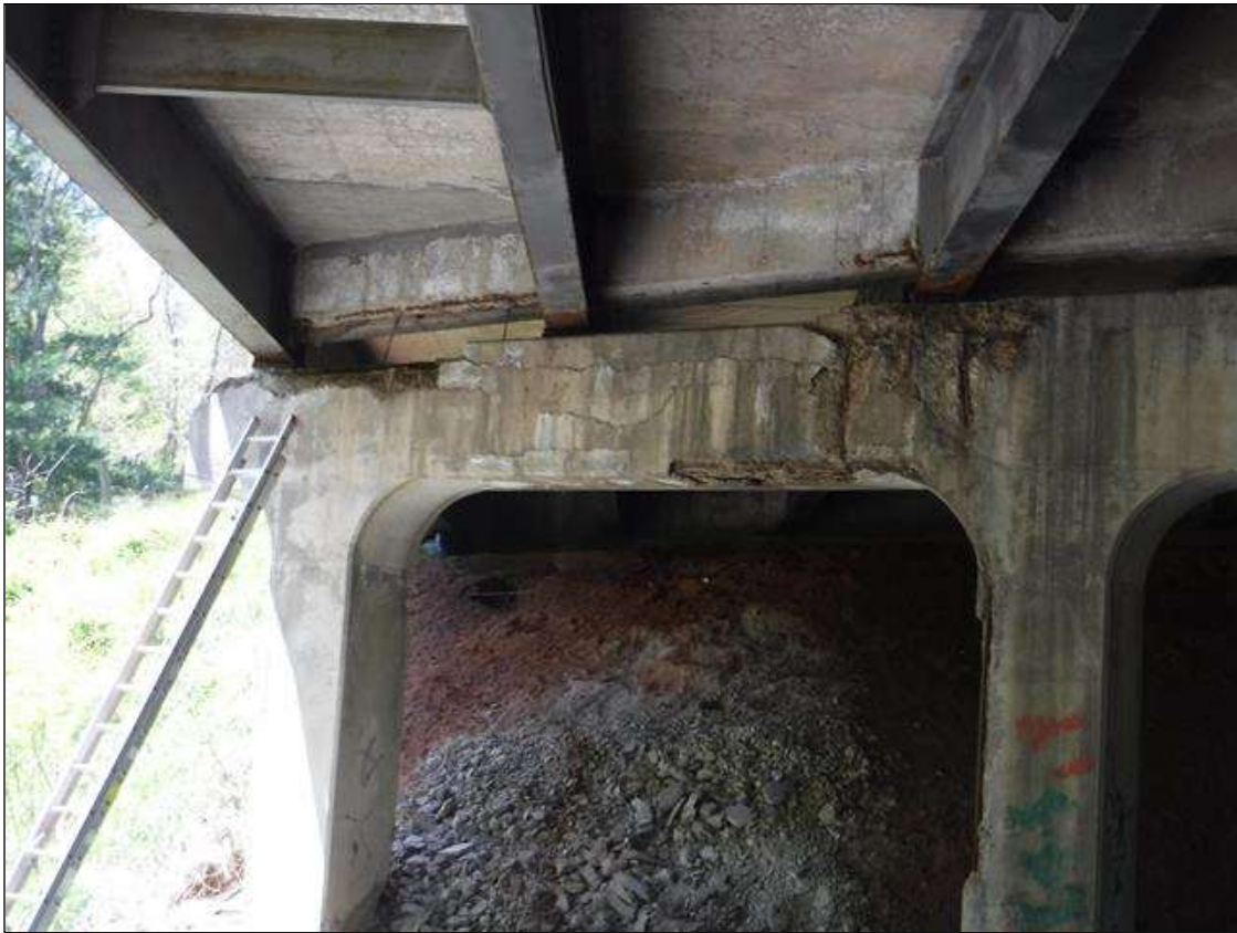
Bent 1 Cap 1: PAR: UP TO 64" X 42" X 3" DEEP SPALLS WITH EXPOSED REBAR, 16' X 24" AREAS OF DELAMINATION AND UP TO 1 1/2" LONGITUDINAL, TRANSVERSE, DIAGONAL AND HORIZONTAL CRACKS IN TOP, BOTTOM, RIGHT END AND BOTH FACES OF CAP FROM BENEATH BEAM 8 TO RIGHT END, CONDITION IN SPAN 2 FACE SHOWN
