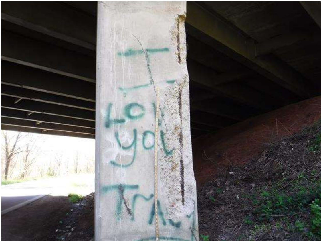
Bent 1 Pile 1: PAR: 65" X 12" X 3" SPALL WITH EXPOSED REBAR IN NORTHWEST CORNER OF COLUMN, BEGINNING APPROXIMATELY 2' FROM GROUND LINE
