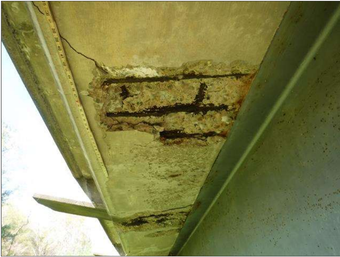
Span 1 Deck: PAR: (6) SPALLS WITH EXPOSED LONGITUDINAL AND TRANSVERSE REBAR UP TO 48" X 24" X 3" DEEP AND AREAS OF DELAMINATION UP TO 60" X 24" ALONG RIGHT OVERHANG, CONDITION APPROXIMATELY 13' FROM END BENT 1 SHOWN
