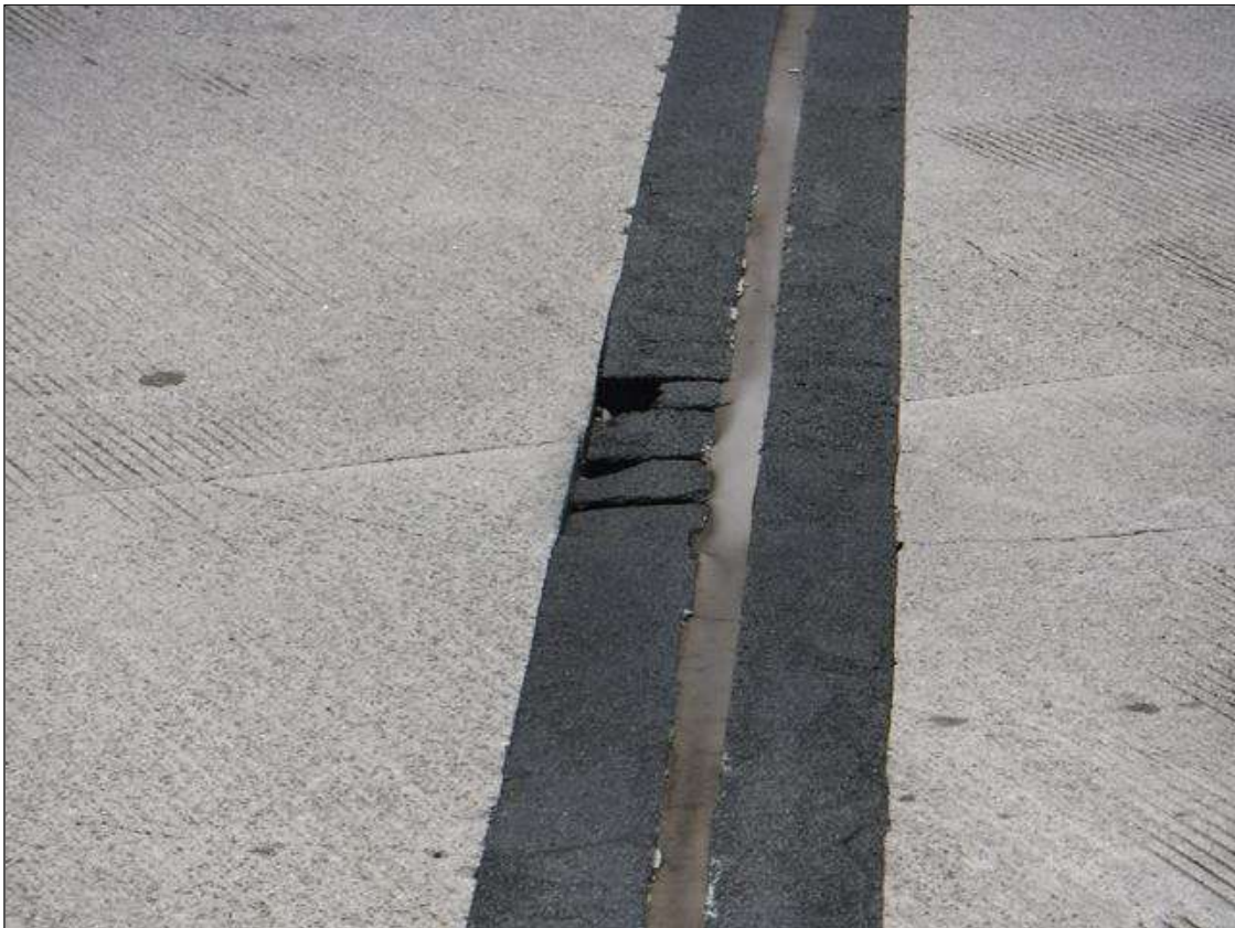
Expansion Joint 3: 14" X 6" AREA OF CRACKED AND BROKEN DECK HEADER ALONG BENT 2 JOINT ALONG CENTERLINE OF EASTBOUND LANES
