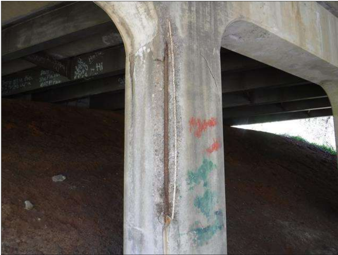
Bent 1 Pile 4: PAR: 96" X 8" X 7" SPALL WITH EXPOSED REBAR IN SOUTHEAST CORNER OF COLUMN EXTENDING FROM BOTTOM OF CAP
