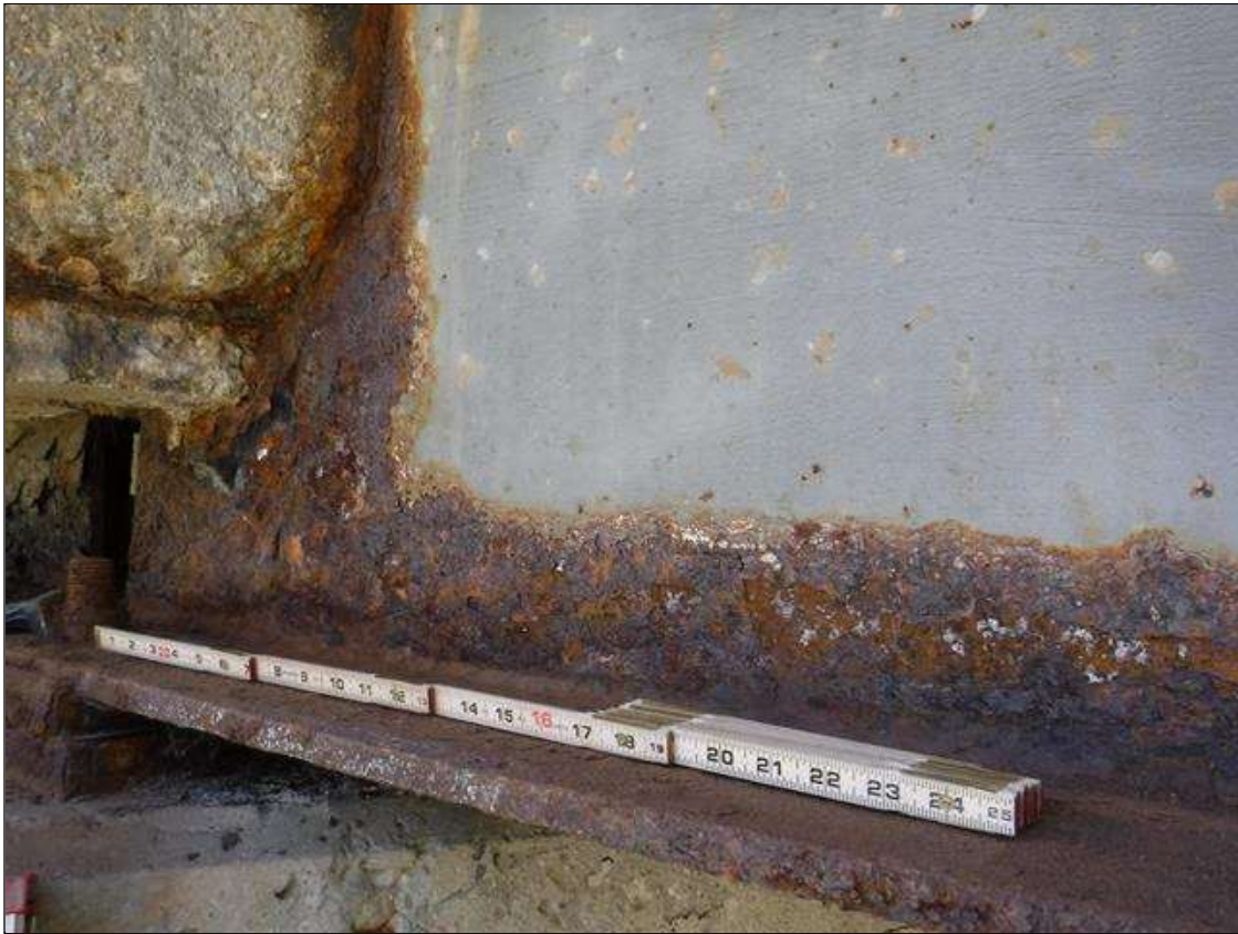
Span 2 Beam 1: CORROSION WITH NO MEASURABLE LOSS OF SECTION ALONG WEB AND BOTTOM FLANGE UP TO 16' LONG X 14" HIGH IN WEB, AND 16' LONG X 11 1/2" WIDE IN FLANGE EXTENDING FROM END OF BEAM AT BENT 2, CONDITION ON LEFT SIDE SHOWN
