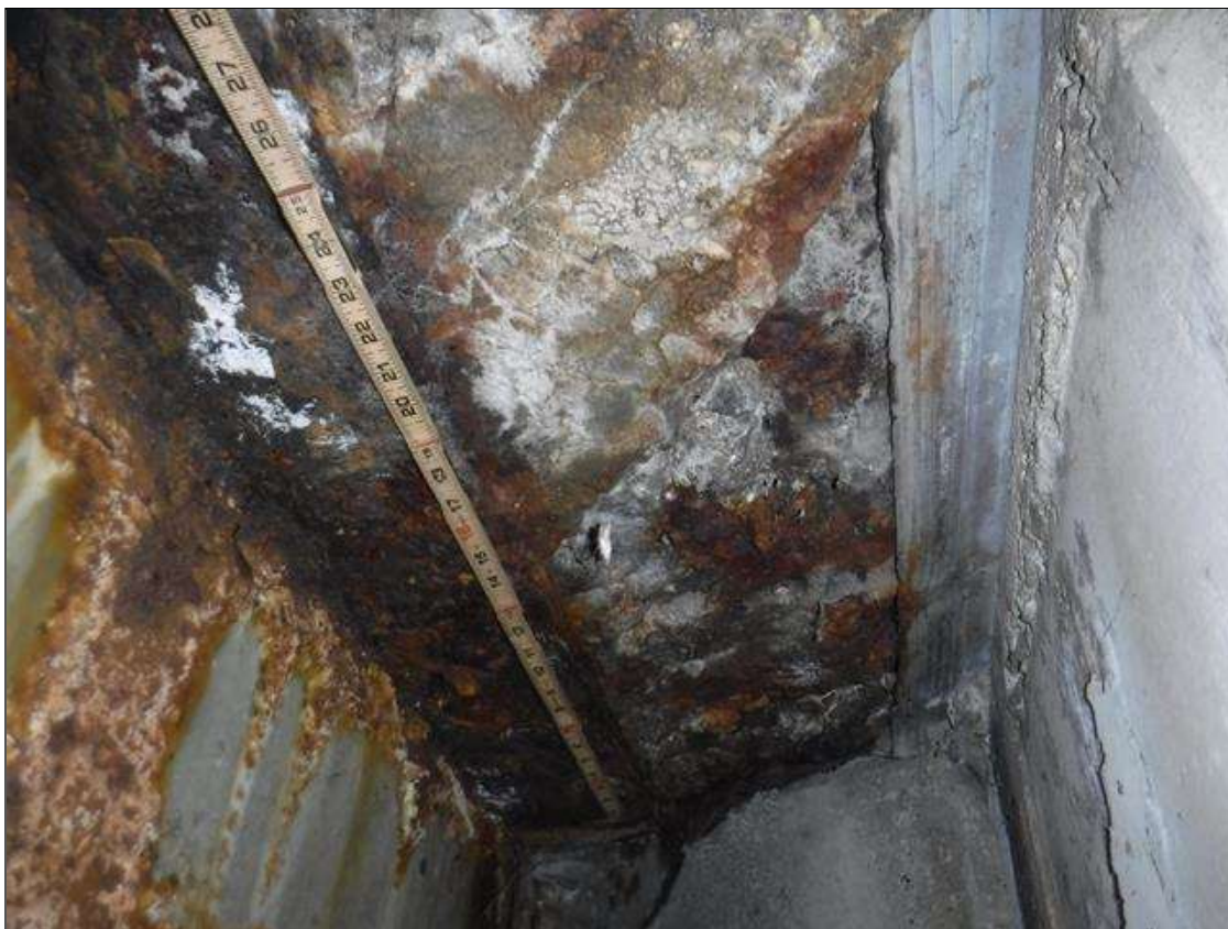
Span 1 Deck: 26" X 11" X 2" DEEP SPALL IN BOTTOM OF DECK TO LEFT OF BEAM 1 AT END BENT 1
