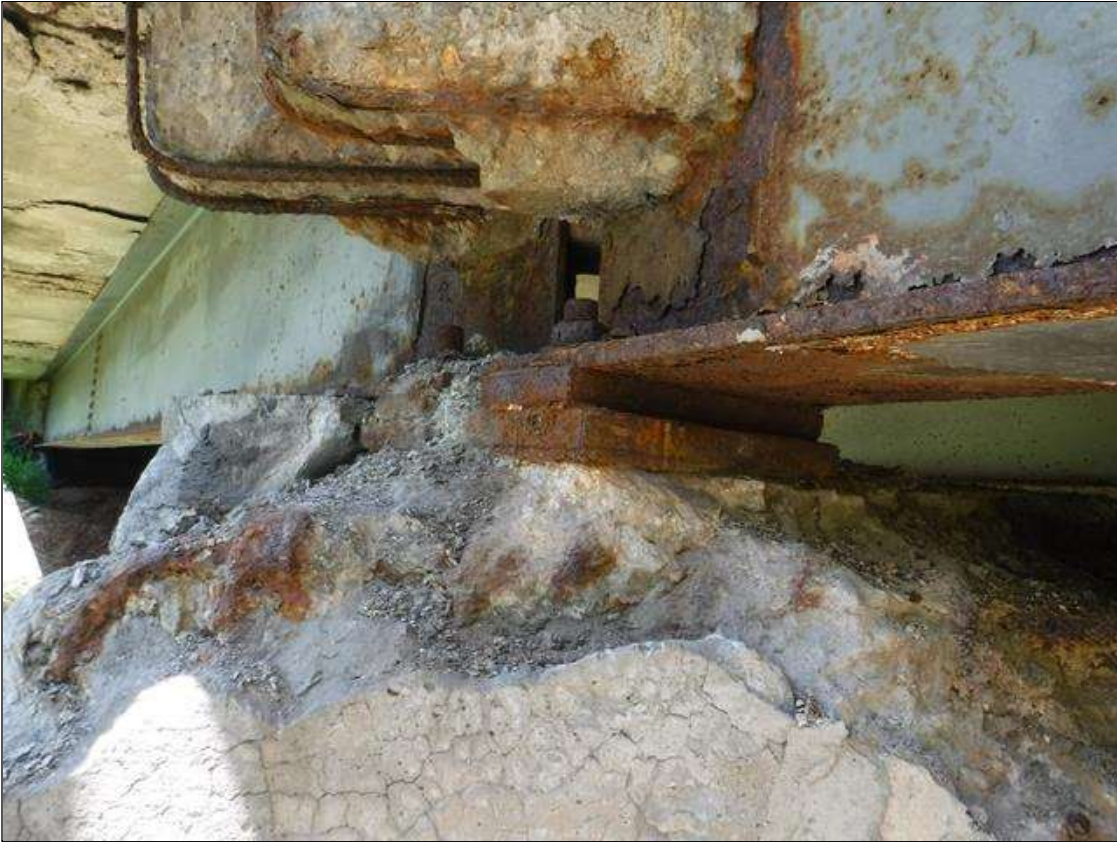
Bent 1 Cap 1: PAR: UP TO 64" X 42" X 3" DEEP SPALLS WITH EXPOSED REBAR, 16' X 24" AREAS OF DELAMINATION AND UP TO 1 1/2" LONGITUDINAL, TRANSVERSE, DIAGONAL AND HORIZONTAL CRACKS IN TOP, BOTTOM, RIGHT END AND BOTH FACES OF CAP FROM BENEATH BEAM 8 TO RIGHT END, CONDITION IN SPAN 2 FACE BENEATH BEAM 10 SHOWN
