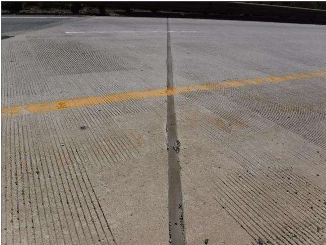
END BENT 2 JOINT IN EASTBOUND LANES, END BENT 1 JOINT SIMILAR
