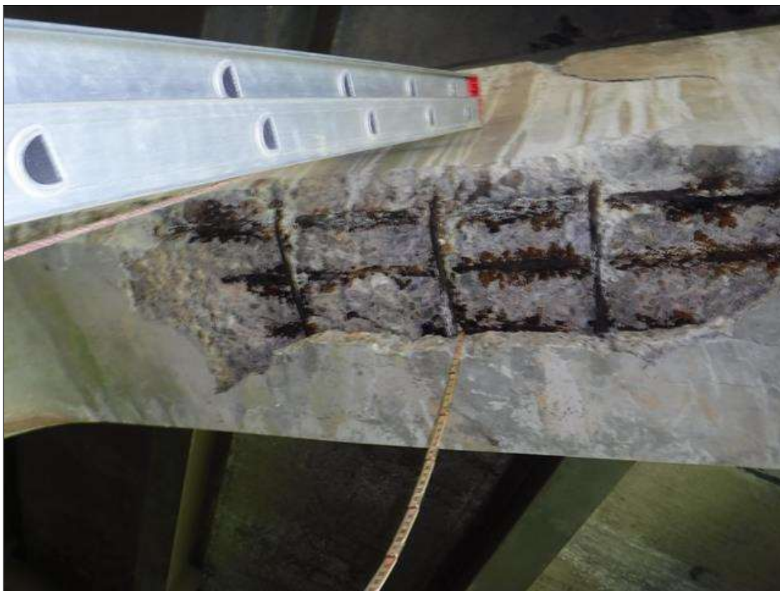
Bent 1 Cap 1: PAR: UP TO 8' X 30" X 3" DEEP SPALLS WITH EXPOSED REBAR, 13' X 6" AREAS OF DELAMINATION AND UP TO 1/2" DIAGONAL AND HORIZONTAL CRACKS IN BOTTOM AND BOTH FACES OF CAP BENEATH BAY 2, CONDITION IN BOTTOM SHOWN
