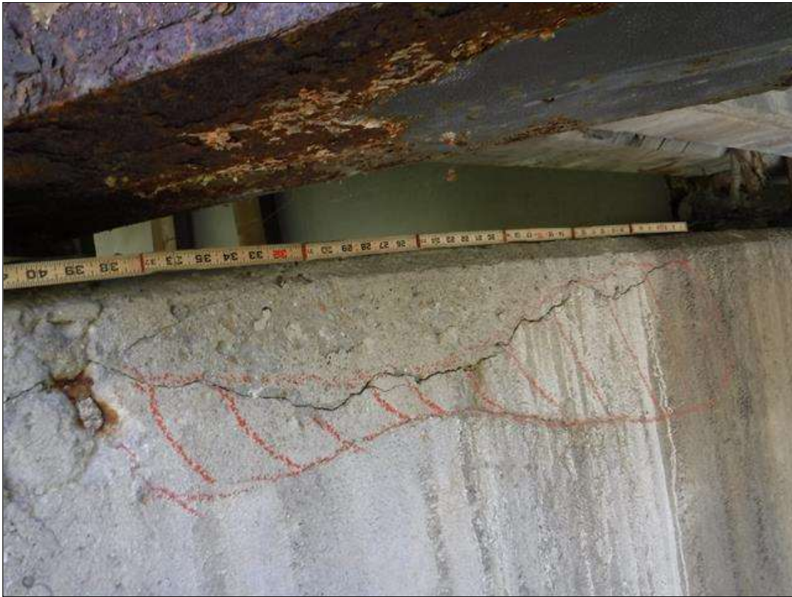
Bent 2 Cap 1: 44" X 8" AREA OF DELAMINATION WITH UP TO 1/16" HORIZONTAL CRACKS IN SPAN 2 FACE OF CAP BENEATH BEAM 1
