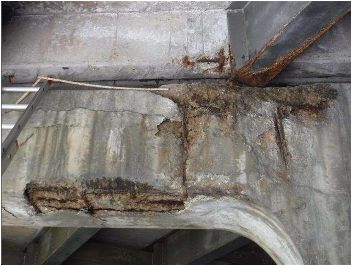
Bent 1 Cap 1: PAR: UP TO 64" X 42" X 3" DEEP SPALLS WITH EXPOSED REBAR, 16' X 24" AREAS OF DELAMINATION AND UP TO 1 1/2" LONGITUDINAL, TRANSVERSE, DIAGONAL AND HORIZONTAL CRACKS IN TOP, BOTTOM, RIGHT END AND BOTH FACES OF CAP FROM BENEATH BEAM 8 TO RIGHT END, CONDITION IN SPAN 2 FACE BENEATH BEAM 8 SHOWN
