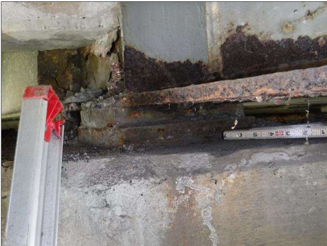
BEAM 3 BEARING AT BENT 2 IN SPAN 2, OTHERS SIMILAR AT BENTS
