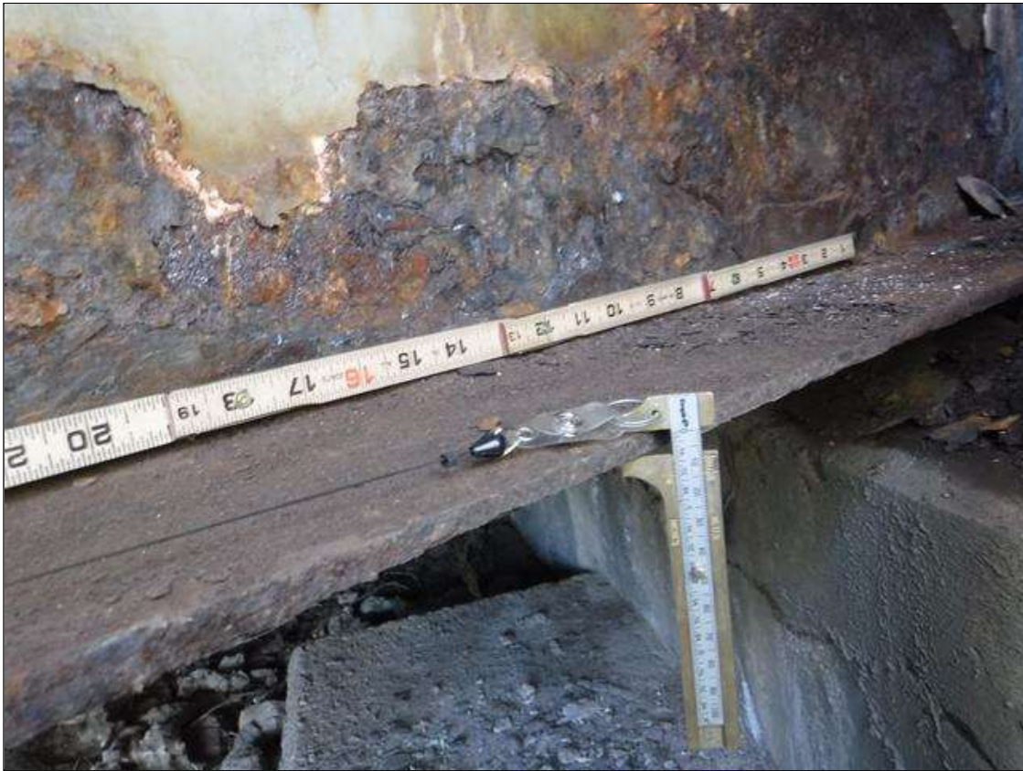
Span 1 Beam 1: PAR: CORROSION ALONG WEB AND BOTH FLANGES UP TO 45" LONG X 14" HIGH DOWN TO 1/4" RESIDUAL WEB, 42" LONG X 6" WIDE WITH NO MEASURABLE LOSS OF SECTION IN TOP FLANGE, AND 46" LONG X 6" WIDE DOWN TO 1/4" RESIDUAL BOTTOM FLANGE EXTENDING FROM END OF BEAM AT END BENT 1, CONDITION ON LEFT SIDE SHOWN
