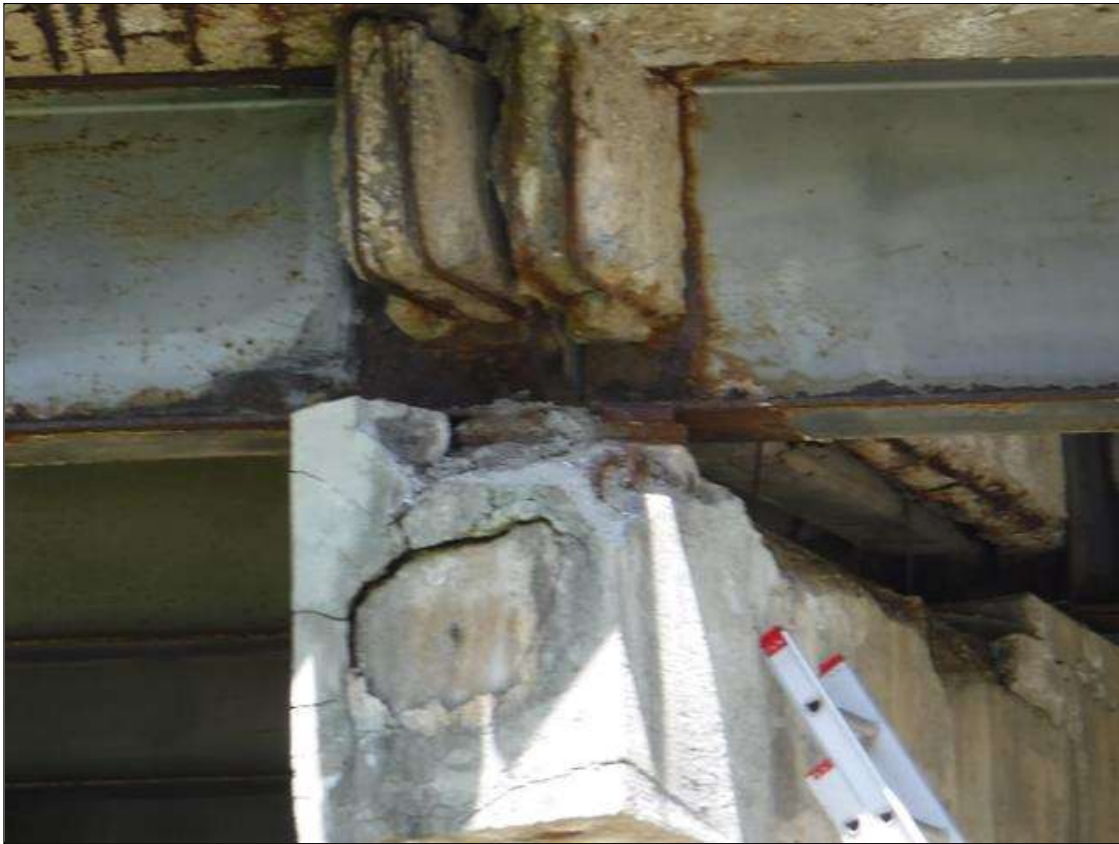
Bent 1 Cap 1: PAR: UP TO 64" X 42" X 3" DEEP SPALLS WITH EXPOSED REBAR, 16' X 24" AREAS OF DELAMINATION AND UP TO 1 1/2" LONGITUDINAL, TRANSVERSE, DIAGONAL AND HORIZONTAL CRACKS IN TOP, BOTTOM, RIGHT END AND BOTH FACES OF CAP FROM BENEATH BEAM 8 TO RIGHT END, CONDITION IN RIGHT FACE SHOWN
