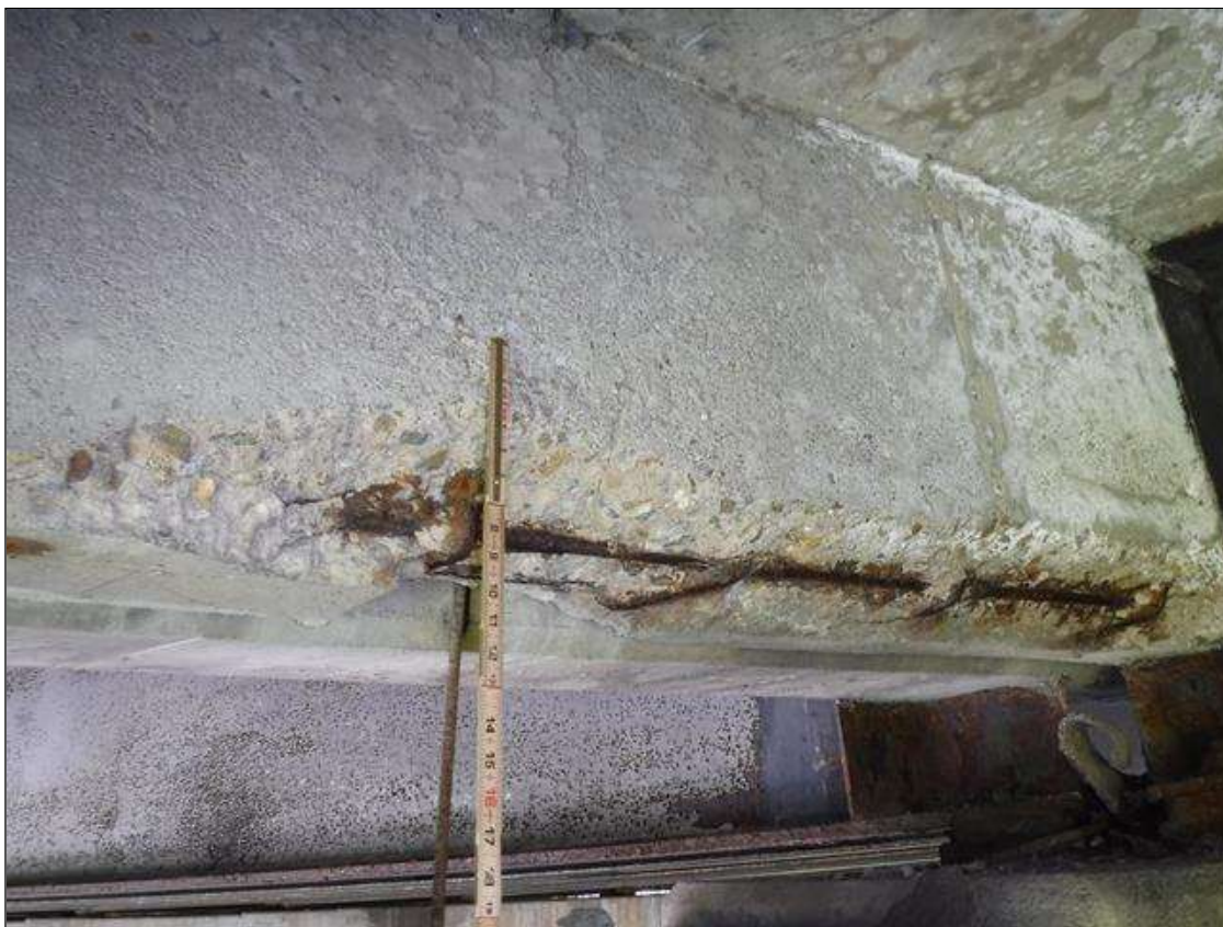
UP TO 60" X 6" X 5" SPALLS WITH EXPOSED REBAR IN BOTTOM AND FACES OF BENT 2 DIAPHRAGMS IN BAYS 2 THRU 9, CONDITION IN SPAN 3 FACE IN BAY 8 SHOWN
