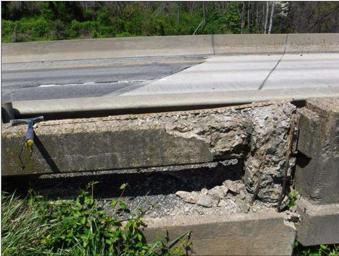
PAR: 42" LONG SPALLED AREA WITH EXPOSED REBAR IN RIGHT APPROACH RAIL AT END BENT 1 JOINT
