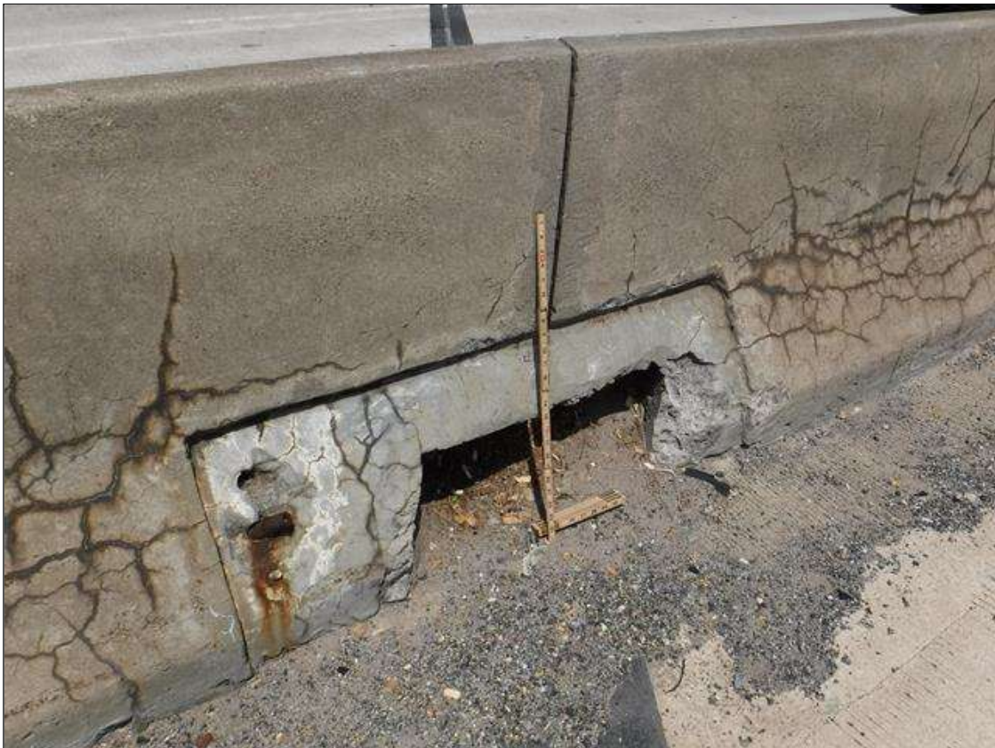
Span 1 Median Bridge Rail: MISSING CONNECTION PLATE ALONG RIGHT FACE OF MEDIAN RAIL AT BENT 1 JOINT
