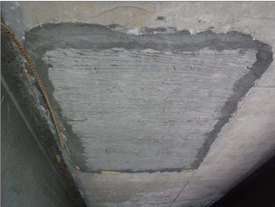
Span 3 Deck: (3) PATCHES UP TO 64" X 48" IN BOTTOM OF DECK IN BAYS 8 AND 9 NEAR END BENT 2, PATCH IN BAY 9 SHOWN
