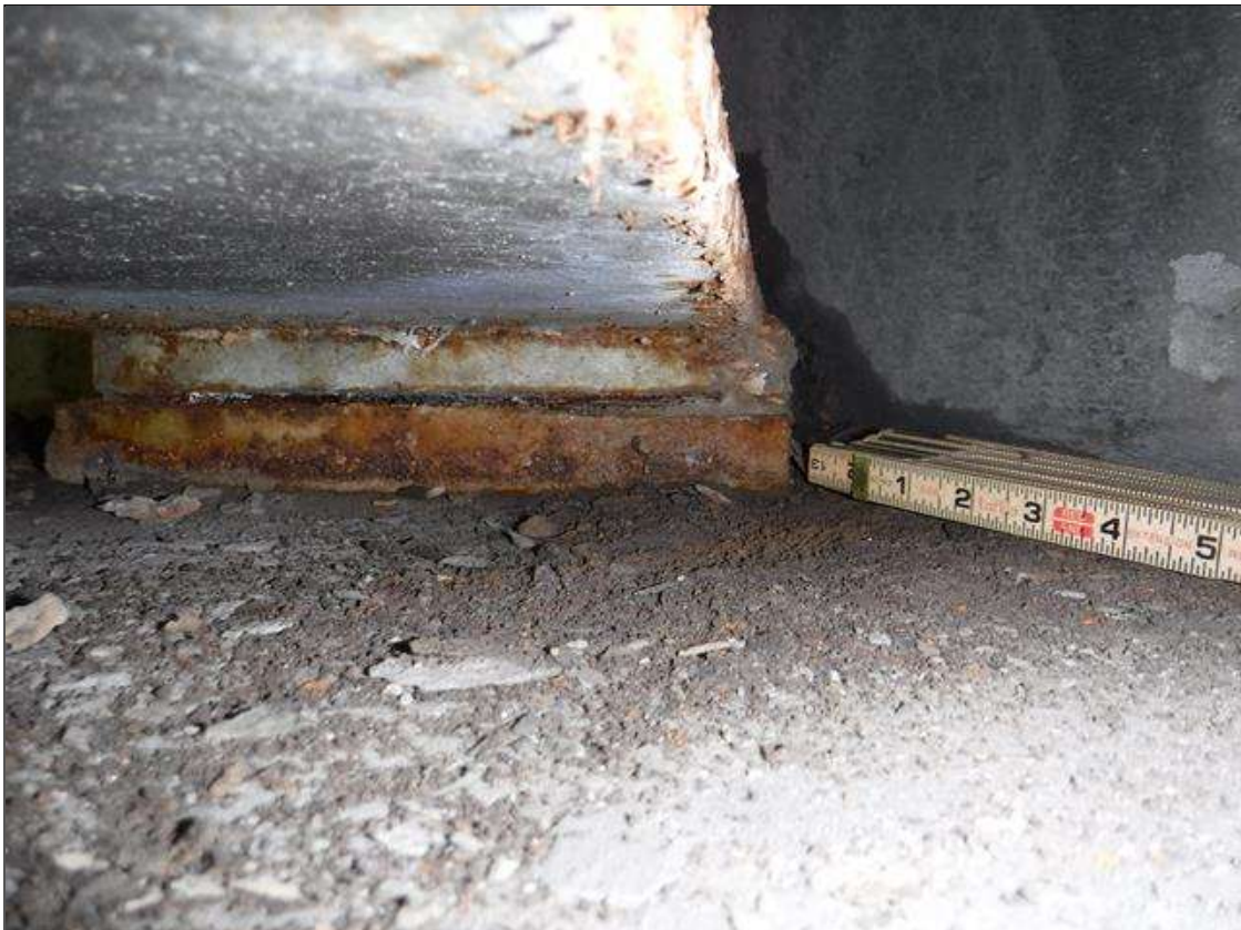
Span 1 Beam 9 Near Bearing: SURFACE CORROSION THROUGHOUT BEAM 9 BEARING
