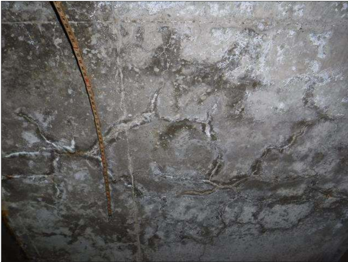
Span 1 Deck: AREAS OF HAIRLINE MAP CRACKING WITH EFFLORESCENCE IN BOTTOM OF DECK IN VARIOUS LOCATIONS, CRACKS IN BAY 2 APPROXIMATELY 17' FROM END BENT 1 SHOWN
