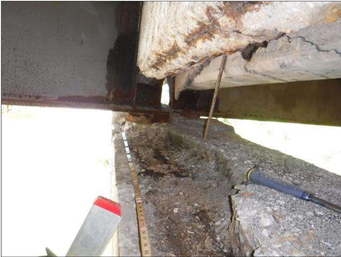
Bent 1 Cap 1: PAR: UP TO 64" X 42" X 3" DEEP SPALLS WITH EXPOSED REBAR, 16' X 24" AREAS OF DELAMINATION AND UP TO 1 1/2" LONGITUDINAL, TRANSVERSE, DIAGONAL AND HORIZONTAL CRACKS IN TOP, BOTTOM, RIGHT END AND BOTH FACES OF CAP FROM BENEATH BEAM 8 TO RIGHT END, CONDITION IN SPAN 2 FACE BENEATH BAY 9 SHOWN
