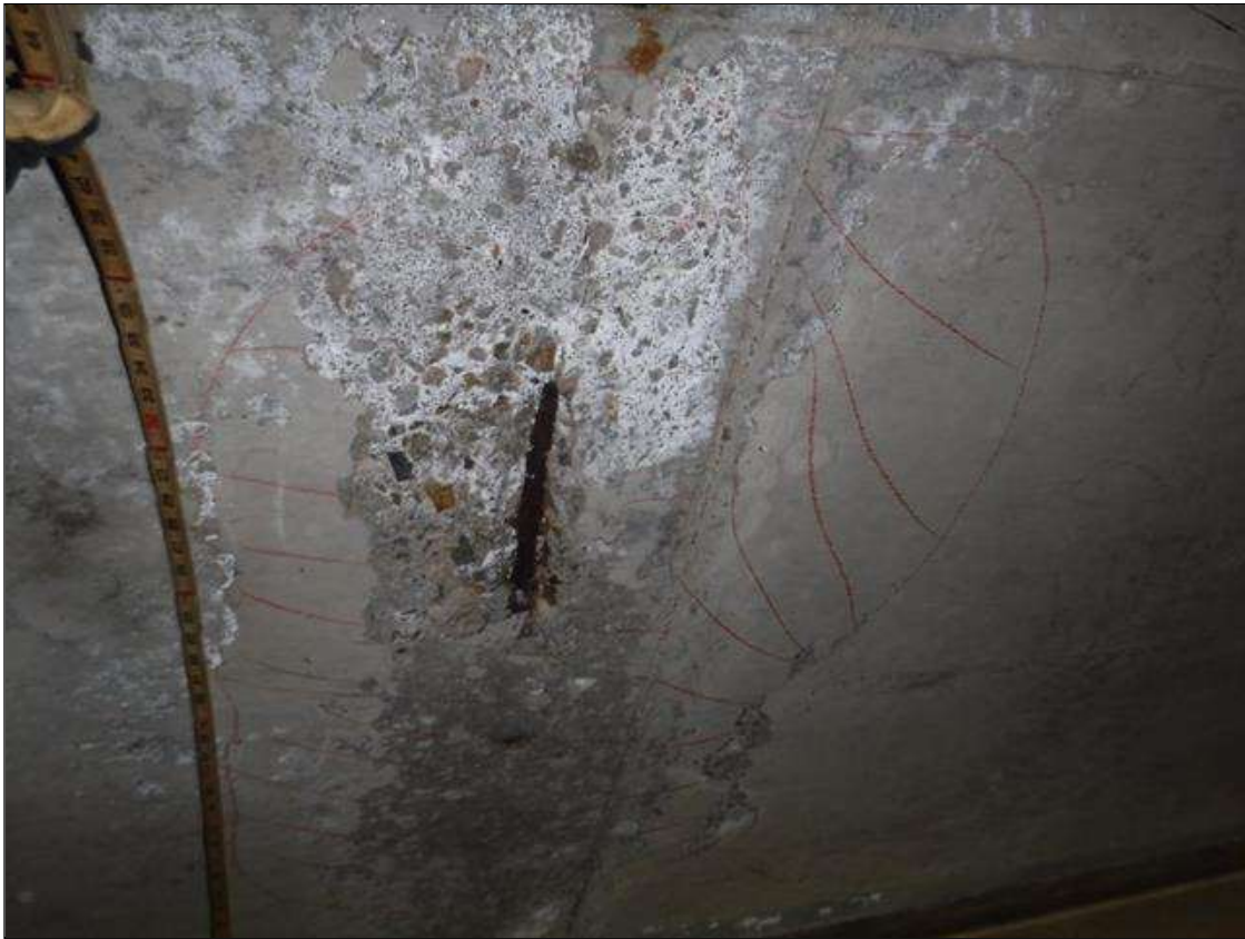
Span 1 Deck: 12" X 6" X 1 1/2" DEEP SPALL WITH EXPOSED REBAR AND 40" X 17" AREA OF DELAMINATION IN BOTTOM OF DECK IN BAY 4, APPROXIMATELY 8' FROM END BENT 1
