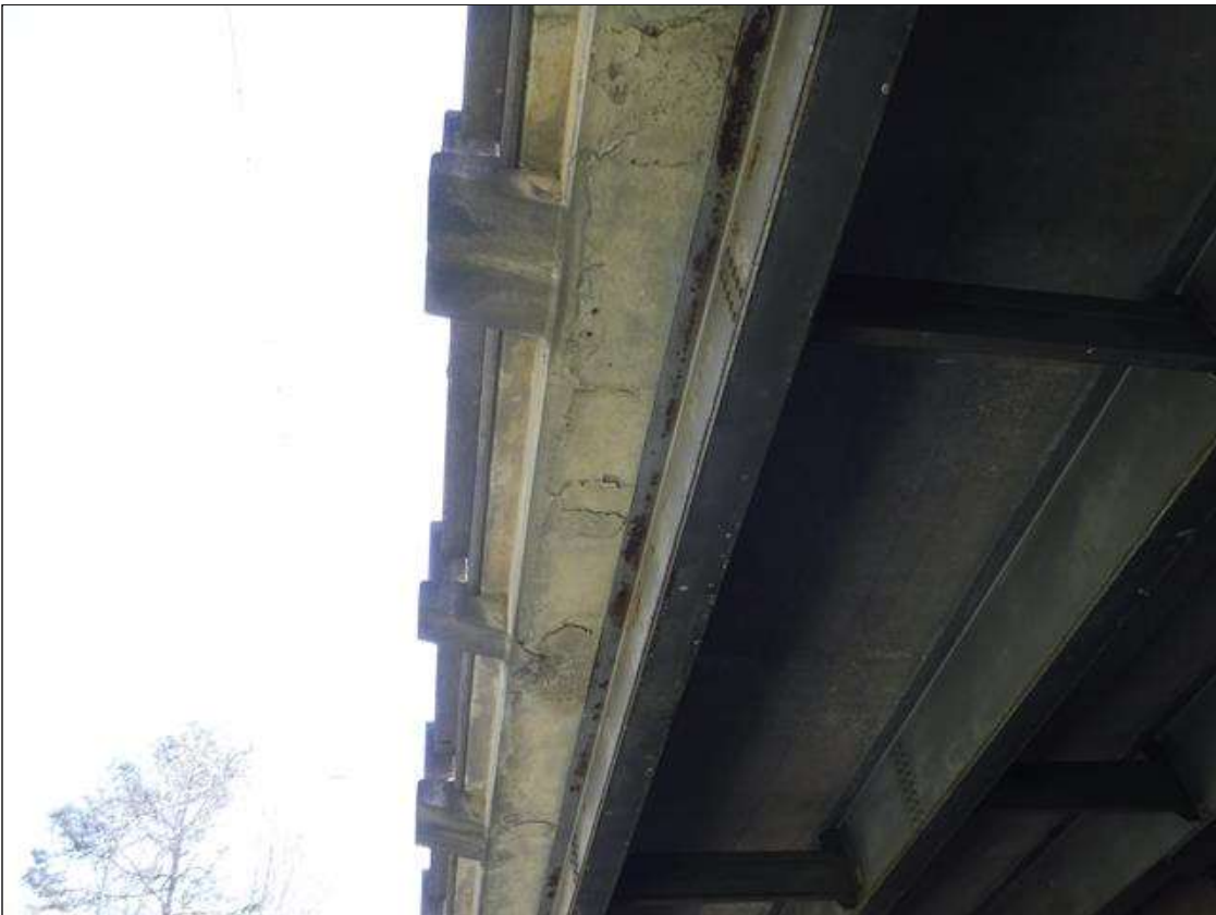
Span 2 Deck: PAR: (4) AREAS OF DELAMINATION UP TO 24" X 24" IN BOTTOM OF LEFT OVERHANG ABOVE ROADWAY
