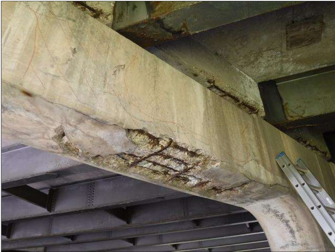
Bent 2 Cap 1: PAR: 125" X 30" X 30" AREA OF DELAMINATION WITH UP TO 1/2" LONGITUDINAL AND HORIZONTAL CRACKS AND 7' X 26" X 4" DEEP SPALL WITH EXPOSED REBAR IN BOTTOM AND BOTH FACES OF CAP TO RIGHT OF COLUMN 4
