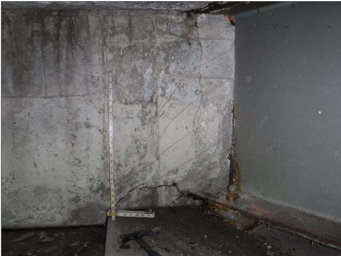
End Bent 1 Abutment/Backwall: FAILED PATCH WITH UP TO 34" X 21" AREA OF DELAMINATION IN FACE OF CURTAIN WALL TO RIGHT OF BEAM 8
