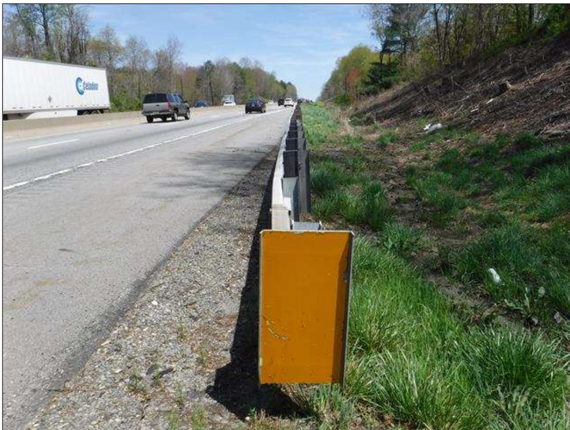
GUARDRAIL END TREATMENT AT SOUTHWEST CORNER, NORTHEAST AND SOUTHEAST CORNERS SIMILAR
