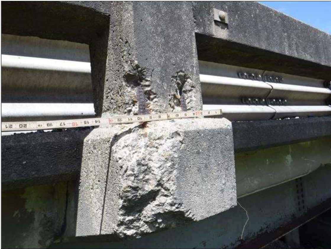
Span 1 Right Bridge Rail: SPALLS WITH EXPOSED REBAR UP TO 18" X 5" X 2" DEEP IN BACK FACE AND BOTTOM OF RAIL AND POSTS IN VARIOUS LOCATIONS, CONDITION APPROXIMATELY 10' FROM END BENT 1 JOINT SHOWN
