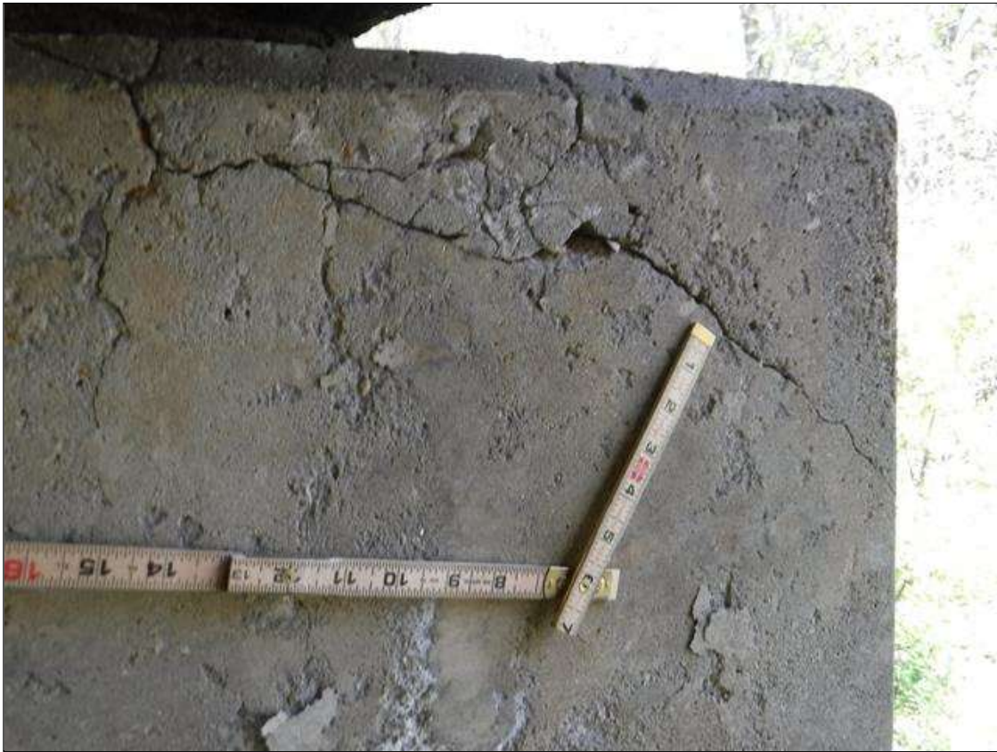
Bent 1 Cap 1: UP TO 1/16" DIAGONAL AND HORIZONTAL CRACKS IN SPAN 2 FACE OF CAP AT LEFT END
