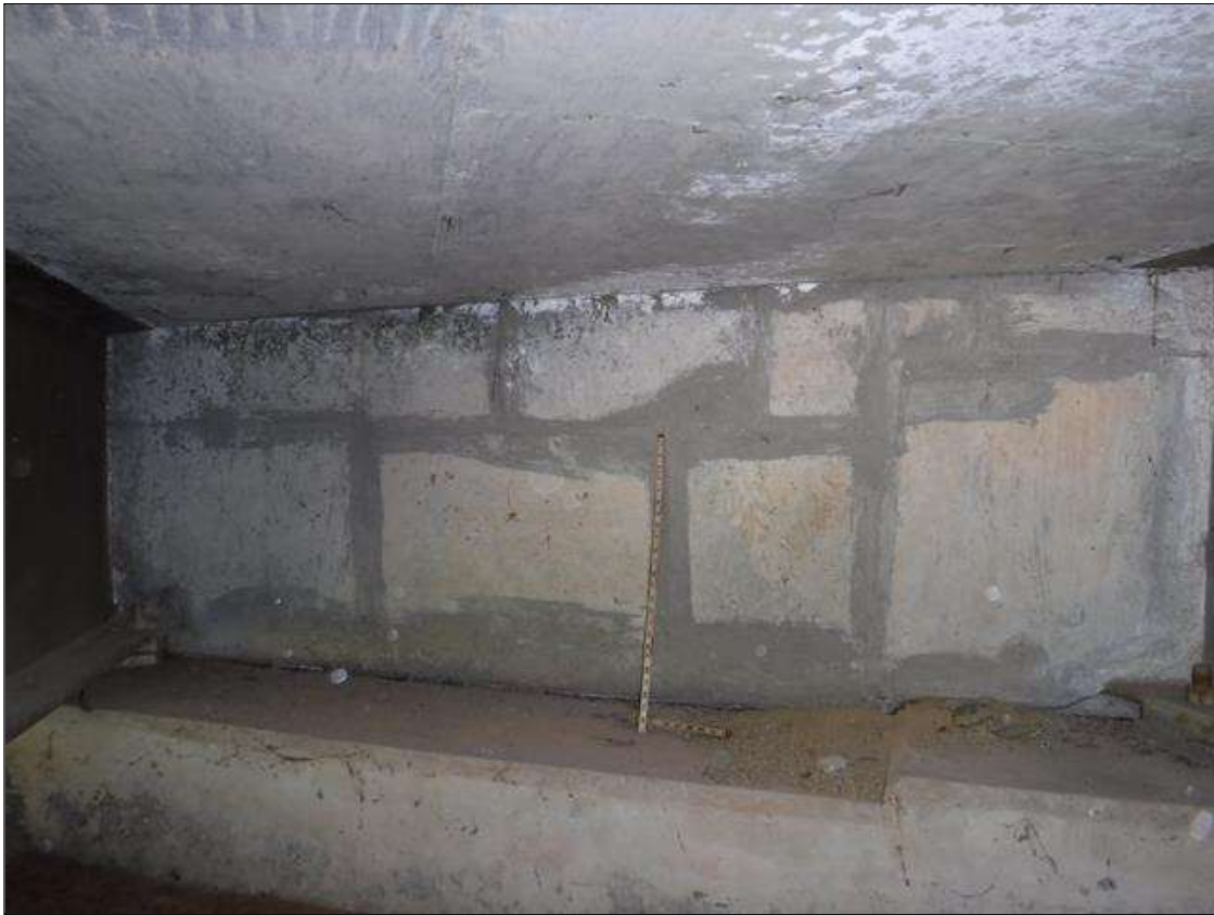
End Bent 1 Abutment/Backwall: UP TO 32" X 16" PATCHES IN FACE OF CURTAIN WALL IN VARIOUS LOCATIONS, CONDITION IN BAY 6 SHOWN
