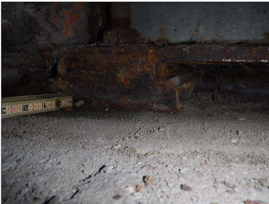
Span 3 Beam 10 Far Bearing: CORROSION THROUGHOUT BEAM 10 BEARING
