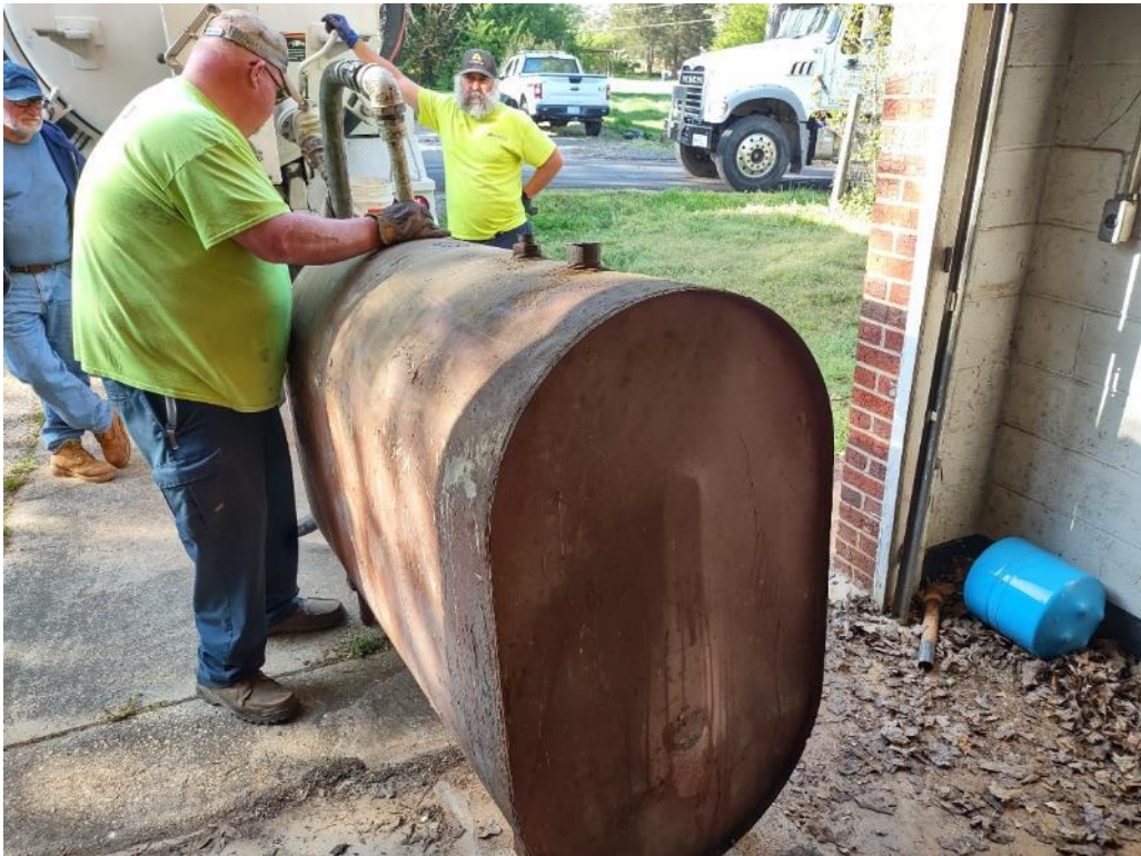
B. Photograph of EVO personnel removing the contents of the AST with the vacuum truck.
