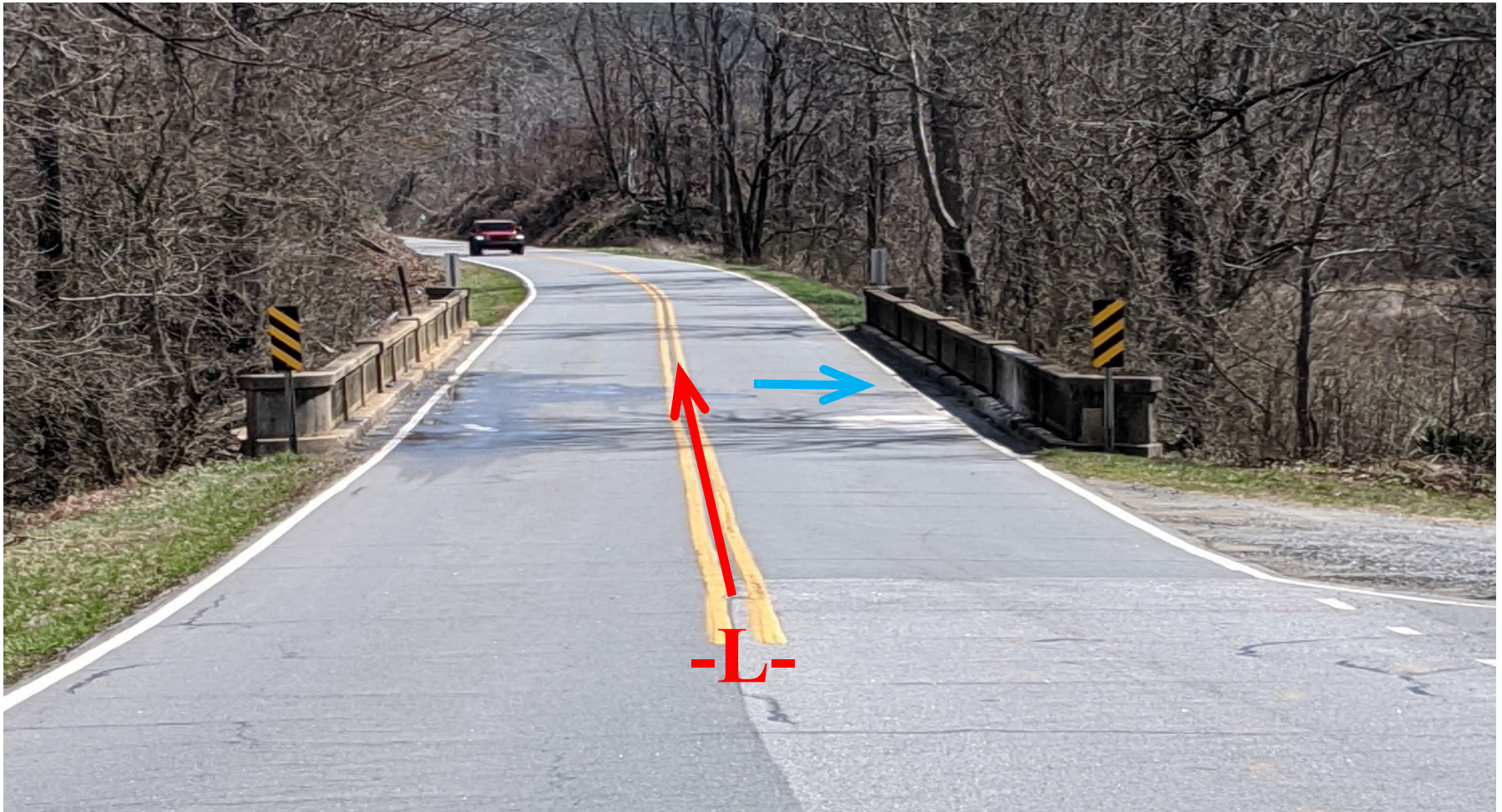
Looking from End Bent 1 toward End Bent 2
