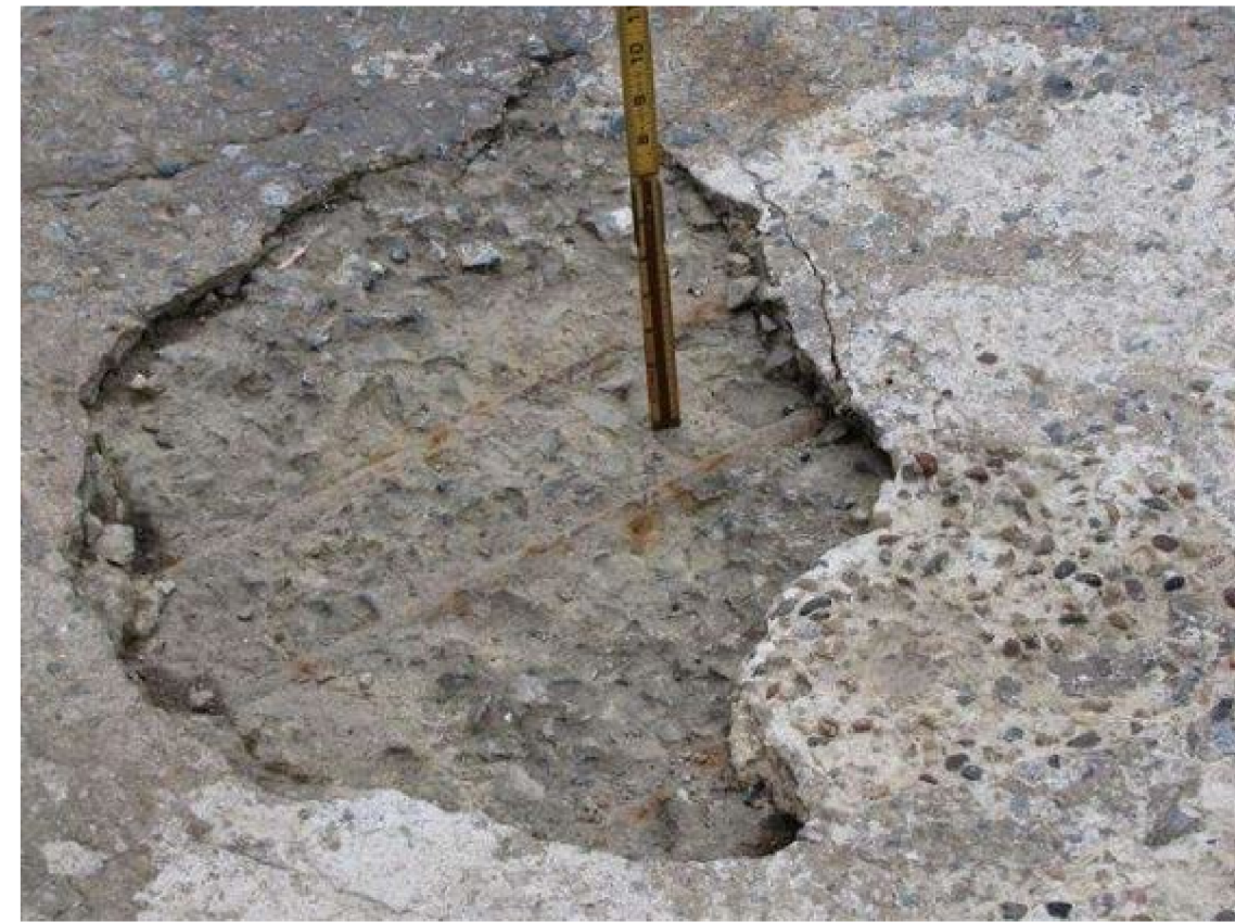
SPAN C CONDITION PHOTO FROM 2016 INSPECTION REPORT
