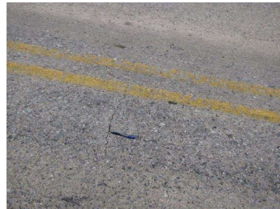
SPAN F CONDITION PHOTO FROM 2016 INSPECTION REPORT
