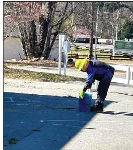
Photo 4. Using asphalt patch to fill in the boring holes at Parcel #001.
