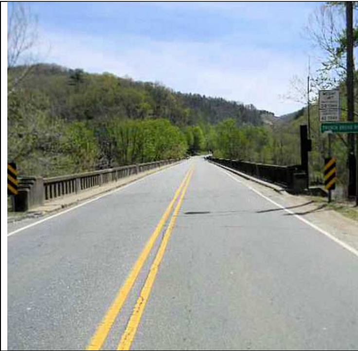
Bridge 67 on US 25/ US 70. View to the east.
