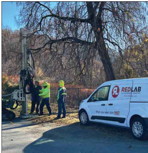
Photo 3. Carolina Soil Investigations drilling boring B-2 & REDLab standing by for samples.
