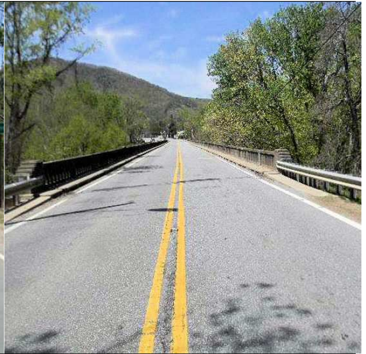
Bridge 67 on US 25/ US 70. View to the west.
