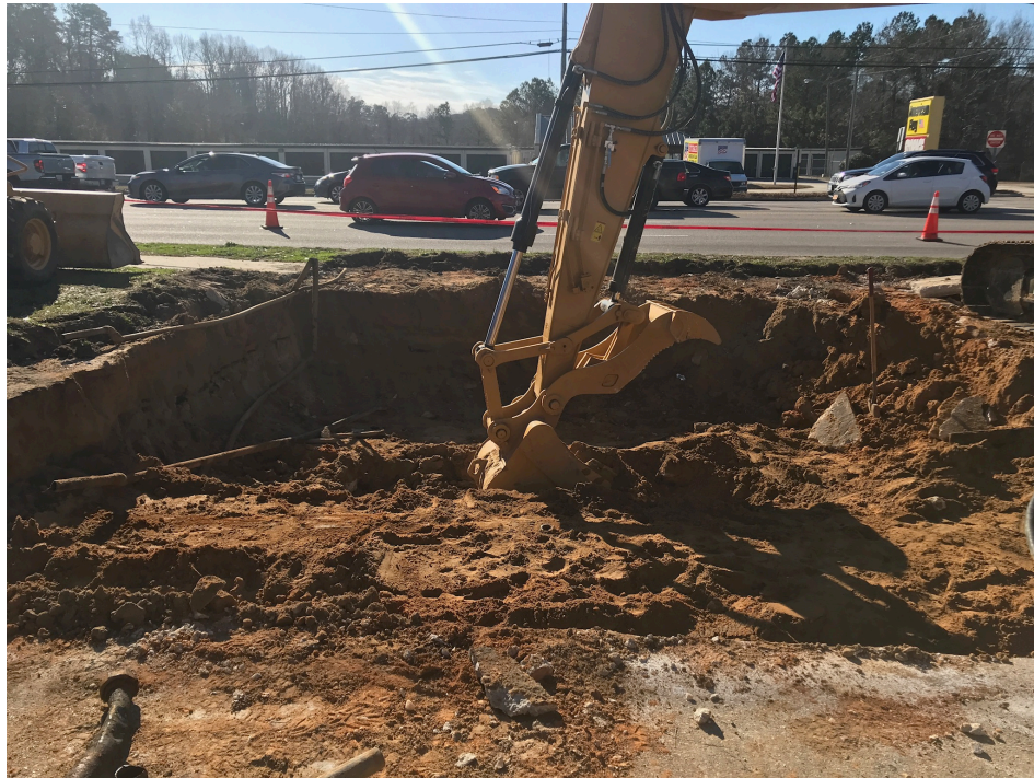
Photo 3: Excavation area prior to tank removal, facing the South.
