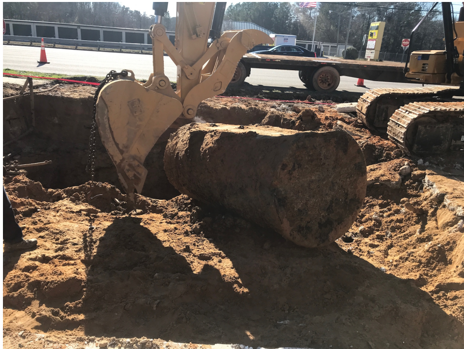
Photo 4: UST-3 removal, 550-gallon kerosene UST
