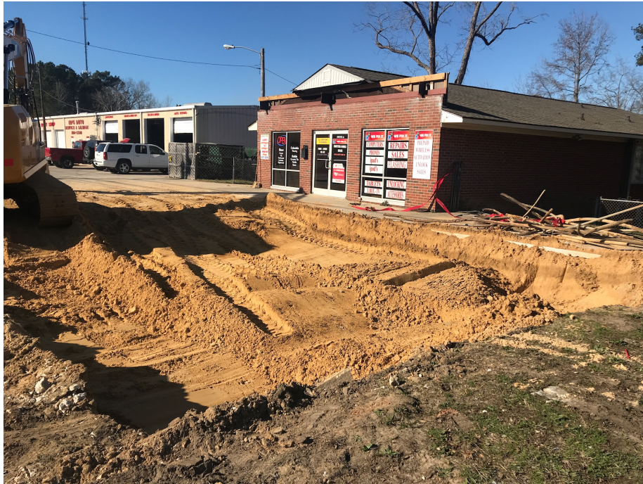
Photo 12: Backfill of excavated area, facing Northwest
