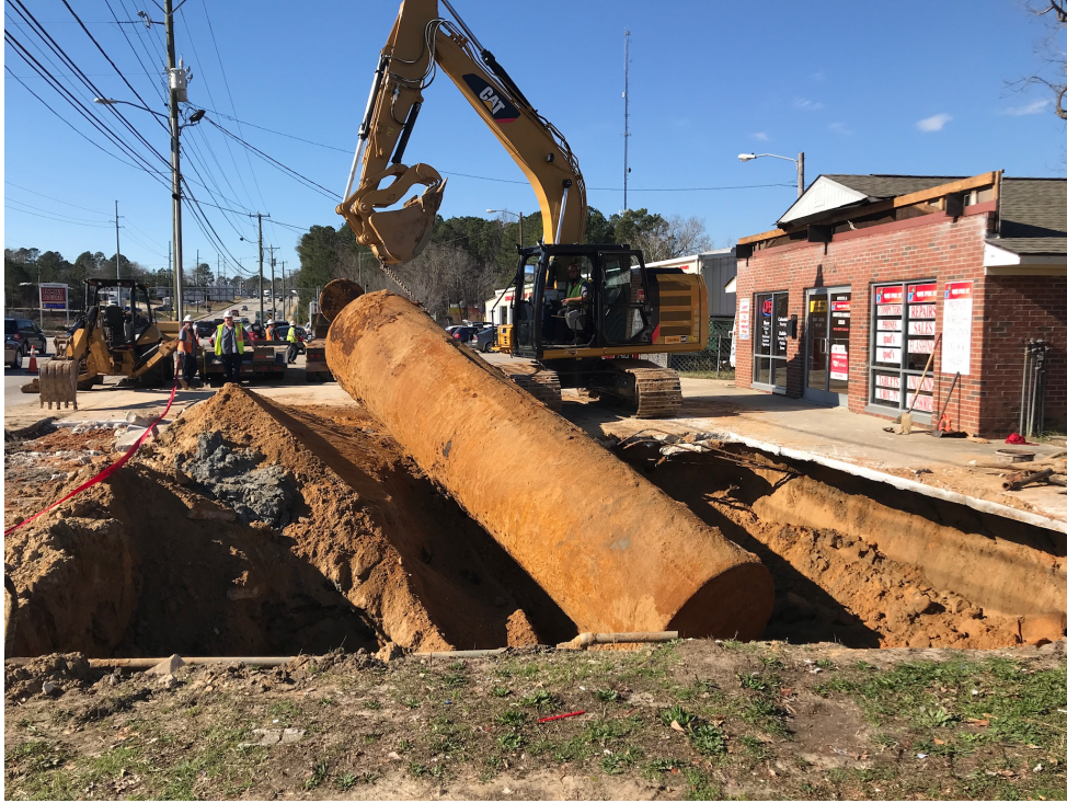
Photo 7: UST-1 removal, 4,000-gallon petroleum UST, facing West
