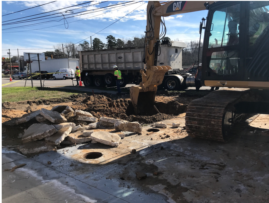
Photo 2: Backhoe excavation of abandoned UST
