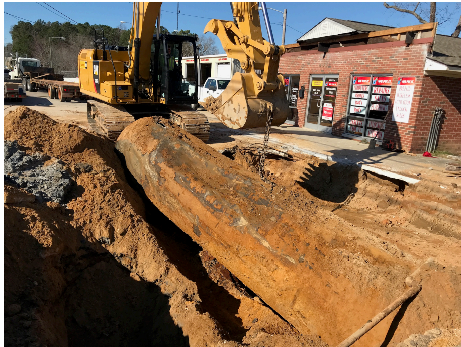
Photo 6: UST-2 removal, 4,000-gallon petroleum UST, facing Northwest
