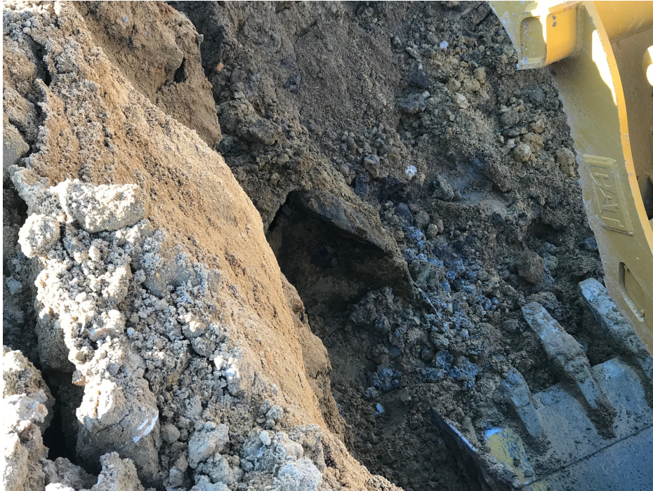
Photo 8: Backhoe excavation of abandoned UST, discovery of UST-4
