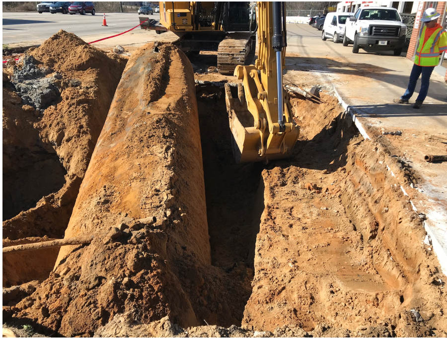
Photo 5: UST-2 removal, 4,000-gallon petroleum UST, facing West
