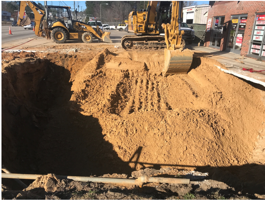
Photo 11: Backfill of excavated area, facing West
