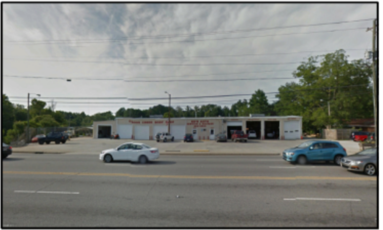
View of Survey Area (Facing Approximately North)
