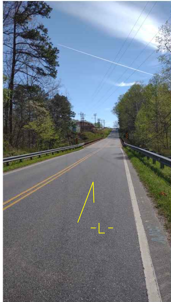
Photo #1: End Bent 1 looking northeast (upstation)
