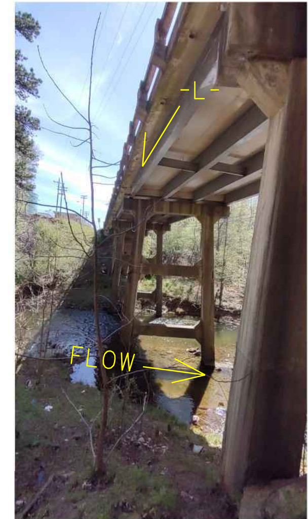
Photo #3: Left side of existing bridge looking northeast (upstation)
