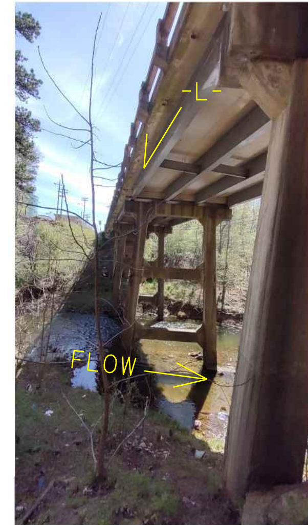
Photo #3: Left side of existing bridge looking northeast (upstation)
