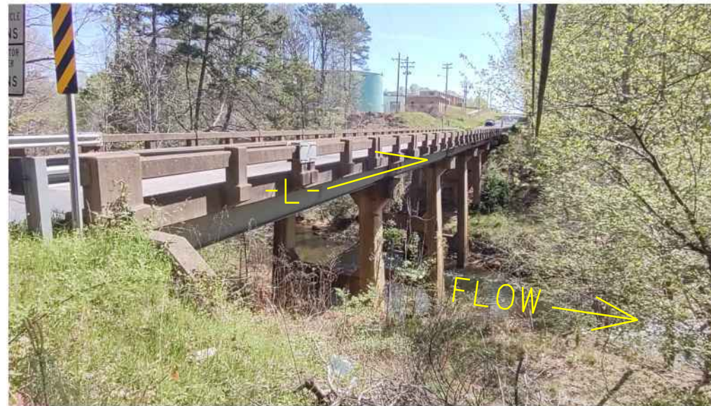
Photo #2: End Bent 1 looking north/northeast (upstation)
