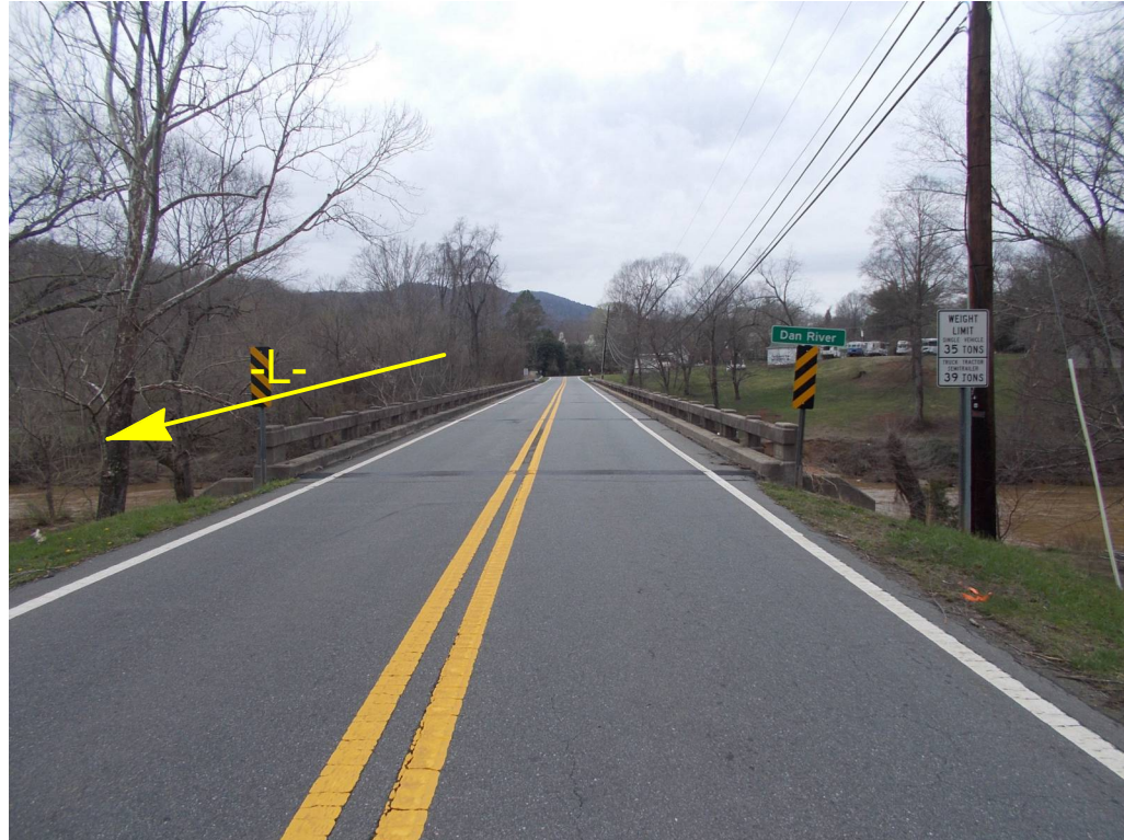
NORTH OF BRIDGE - EAST OF RIVER FACING DOWN STATION LEFT OF -L-
