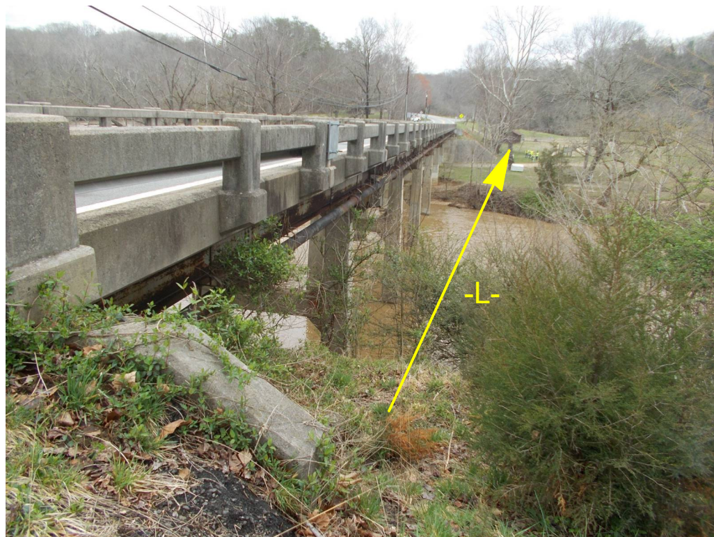
SOUTH OF BRIDGE - WEST OF RIVER FACING UP STATION
