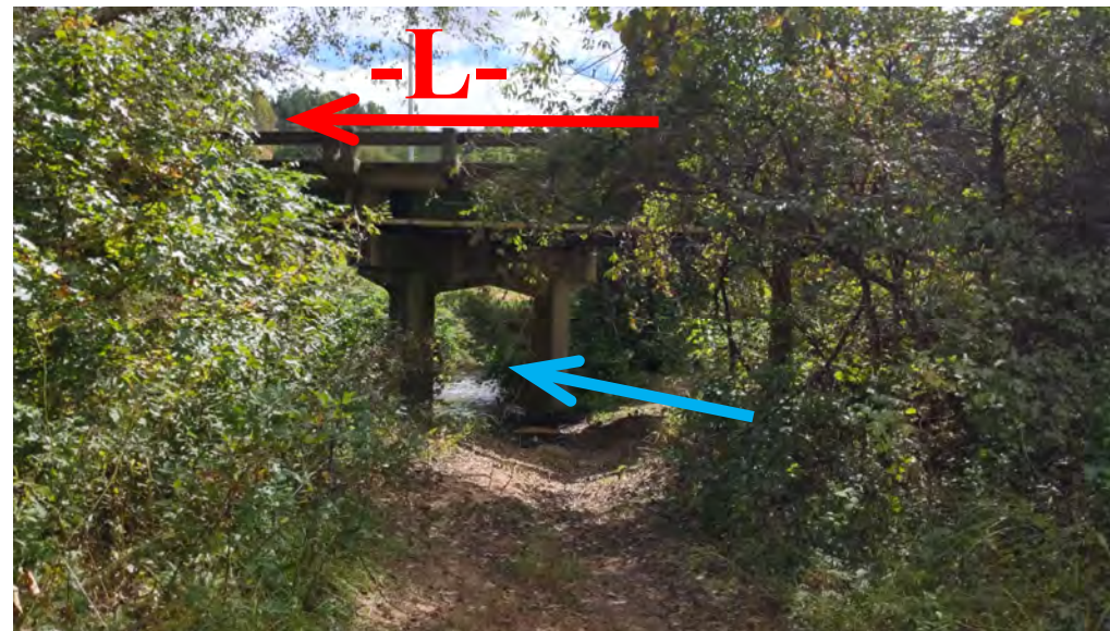
Facing South from North of Existing Bridge
