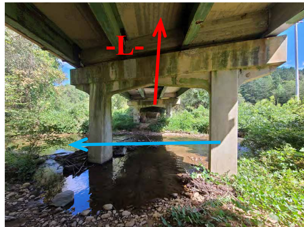
Facing West towards End Bent No. 1
