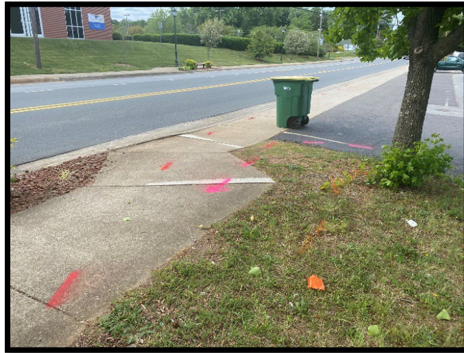
Figure 1 Parcel 39, NC 811 and Pyramid utility mark outs at southwestern portion of property along Shallowford Road
