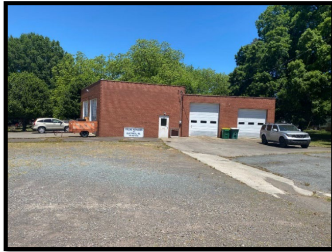
Figure 1 Parcel 37, front view of the building structure, Collins Petroleum and Electrical, Inc.
