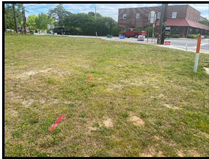
Figure 2 Parcel 39, NC 811 and Pyramid utility mark outs near fiber optic easement, along Shallowford Road.
