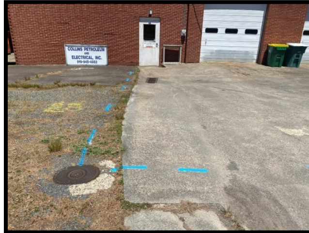
Figure 3 Parcel 37, NC 811 utility mark outs. Northern view of property building structure.
