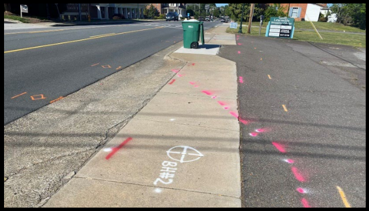
Figure 3 Parcel 17 SB-2 and SB-1 NC811 and Pyramid utility mark outs, within the right-of-way along Shallowford Road.
