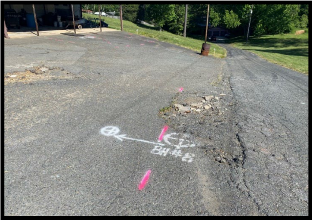
Figure 5 Parcel 31 SB8 Pyramid utility mark out with step-off location.
