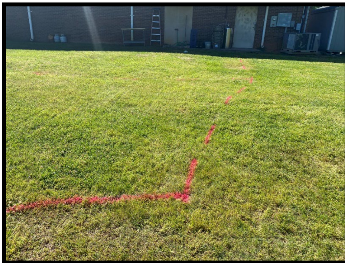
Figure 2 Parcel 34, NC 811 utility mark outs, southern view.
