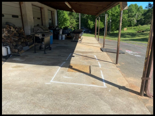
Figure 3 Parcel 31 SB9 with step-off location, and NC 811 and Pyramid utility mark outs adjacent to concrete pad.
