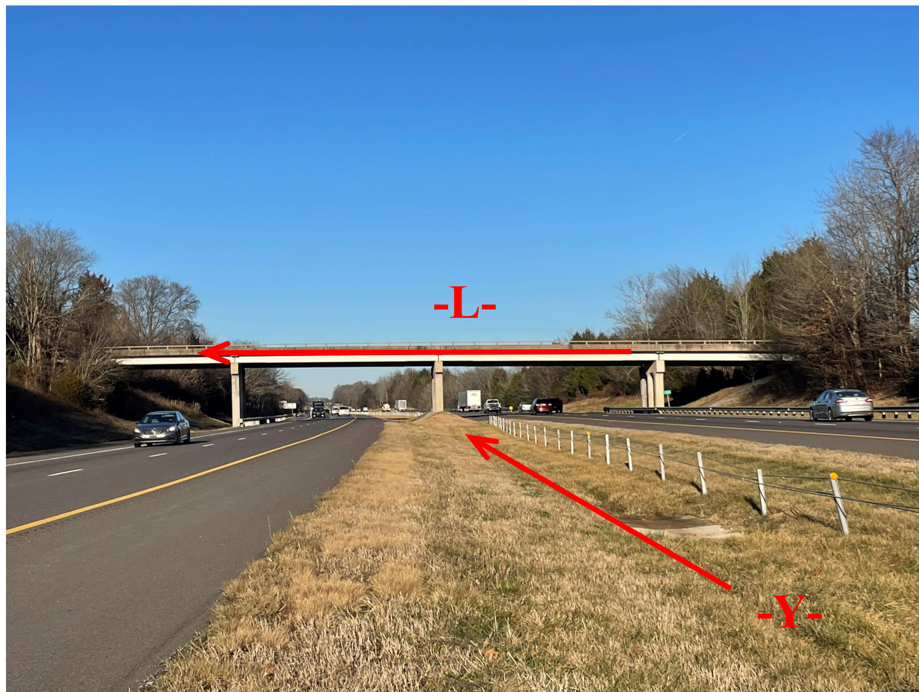
Looking East on I-40 (-Y-) towards Bridge No. 76 on Pinebrook School Road (-L-)
