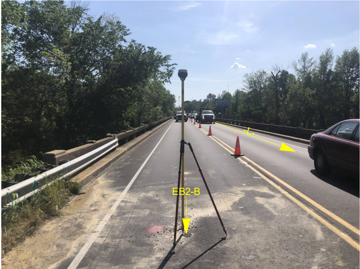
FACING DOWNSTATION ALONG -L- EB2-B IN FOREGROUND
