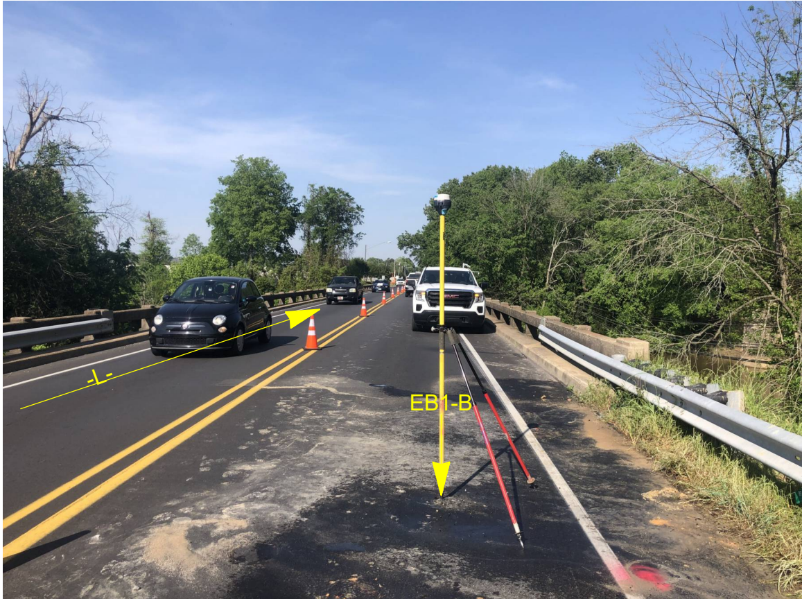
FACING UPSTATION ALONG -L- EB1-B IN FOREGROUND
