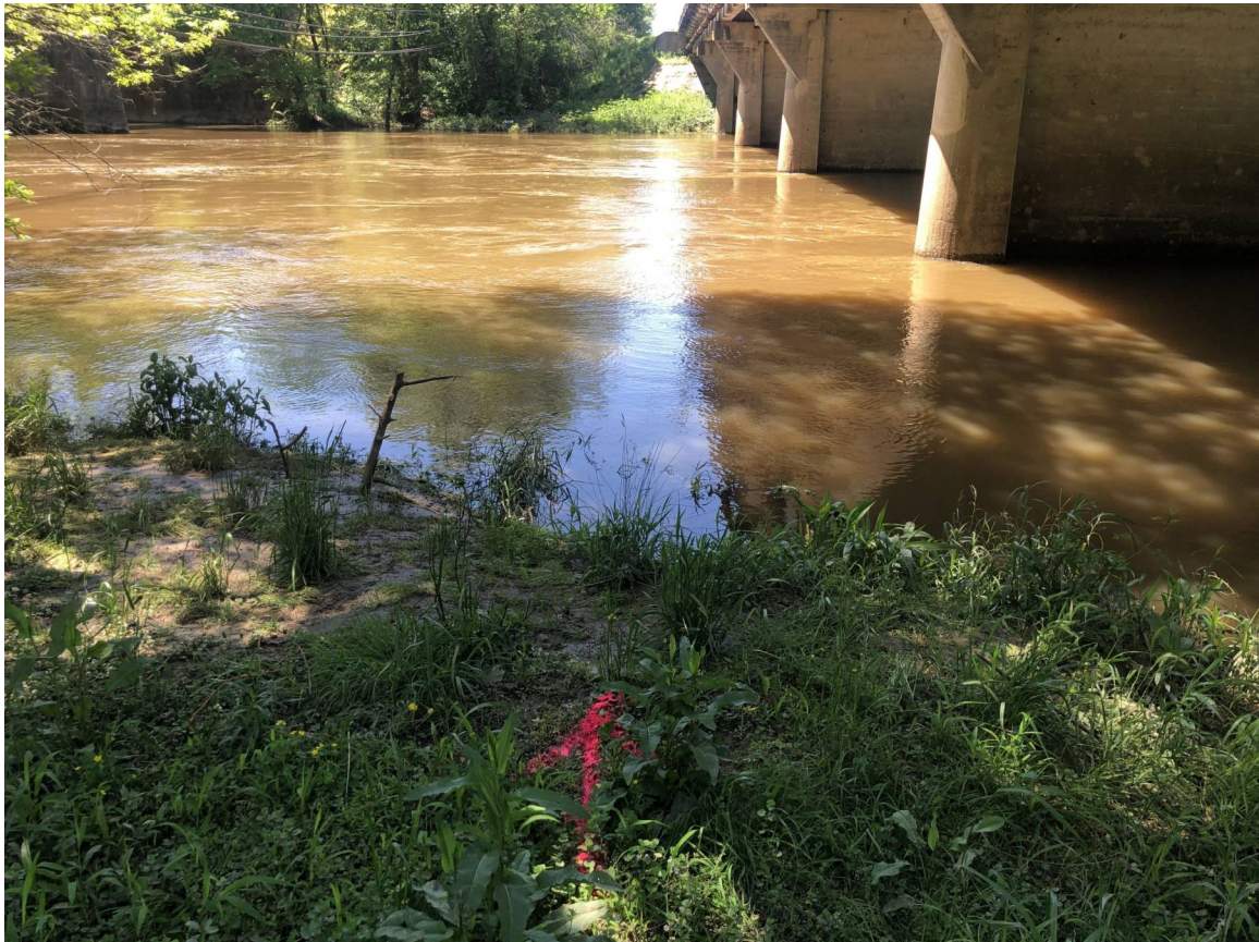
DOWNSTREAM OF BRIDGE 70 NEAR EB2 RIGHT OF -L- FACING SOUTHWEST
