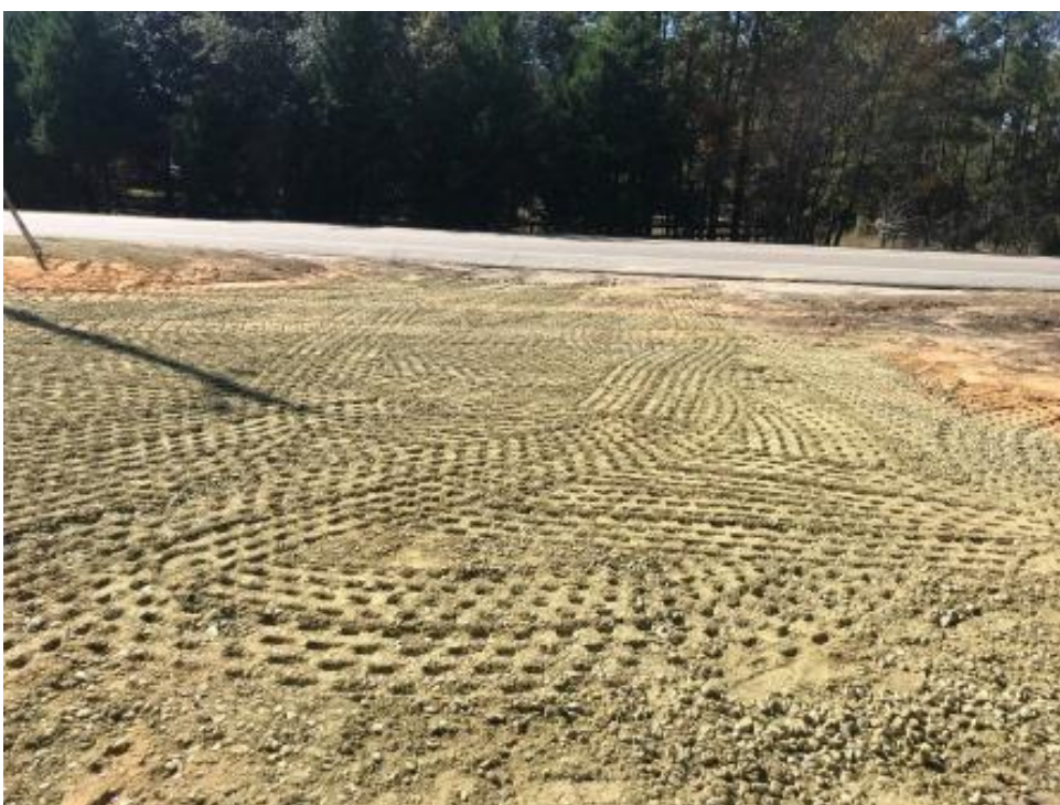
Photograph 16: Photograph of final backfilled excavation.
