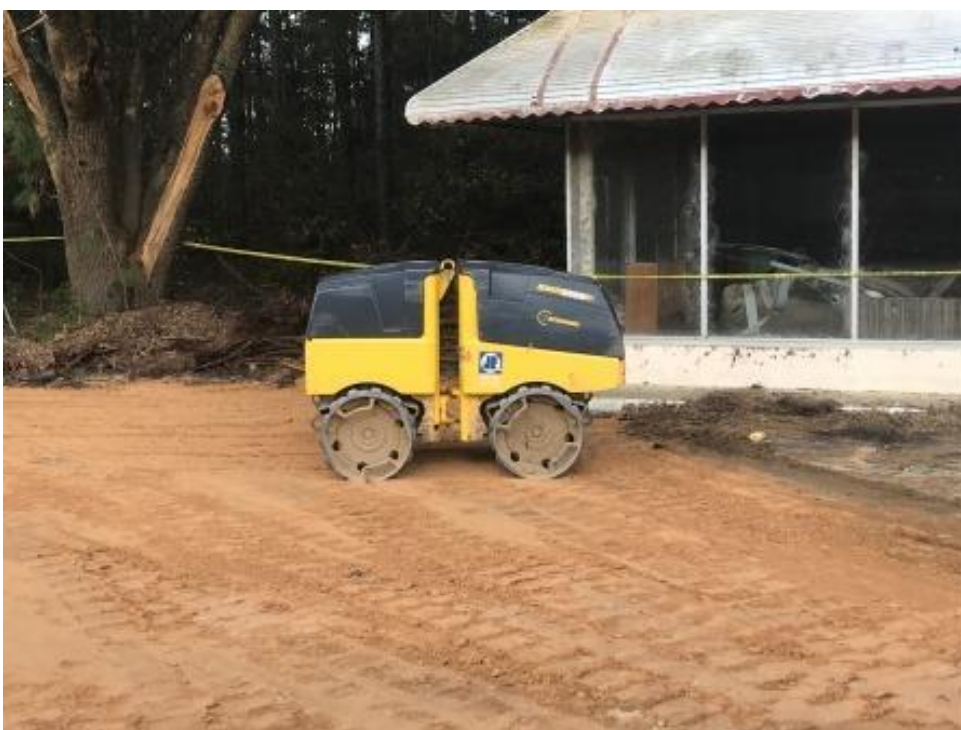
Photograph 14: Photograph of excavation backfilled to the surface.
