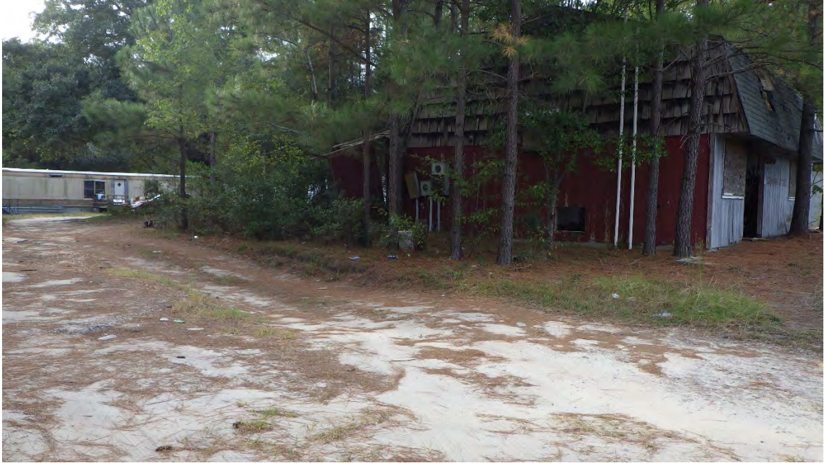
Side of the store building
