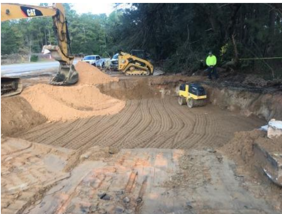
Photograph 12: Evo performing compaction on excavation.
