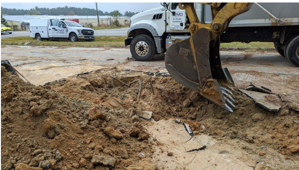
Photograph 5: Removing product lines and dispenser island.
