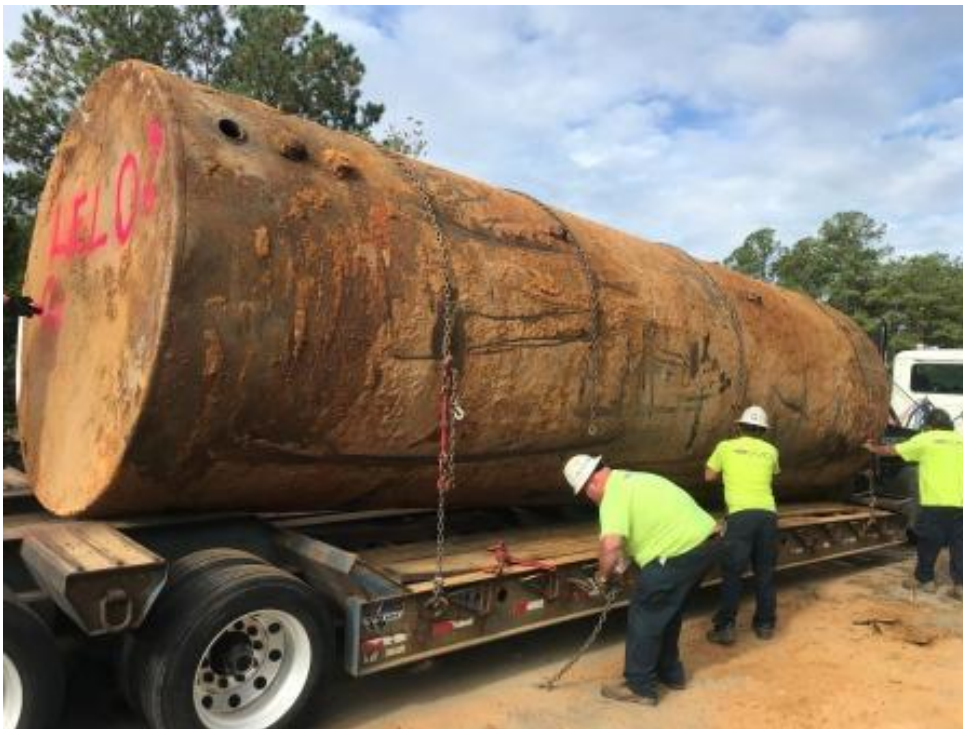
Photograph 6: EVO loading UST#1 on trailer. UST was in good condition, no holes or pitting.
