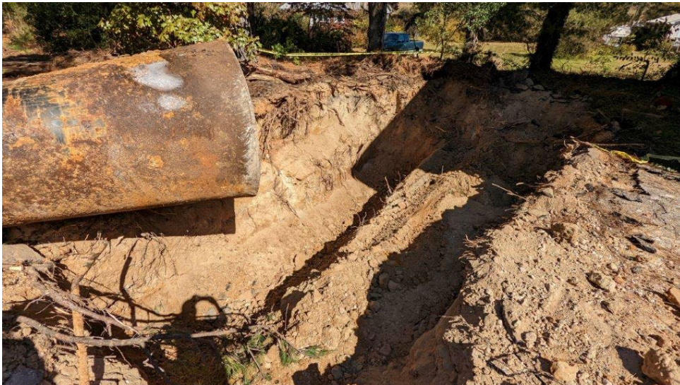
Photograph 2: Removing USTs from the excavation.
