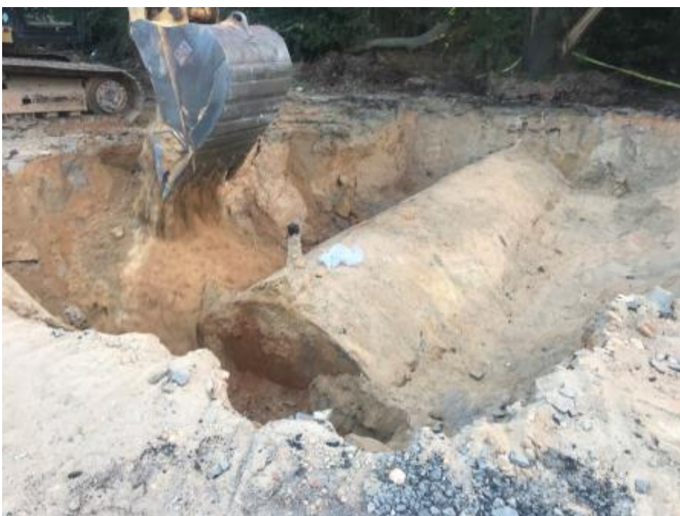
Photograph 2: EVO uncovering UST#1.
