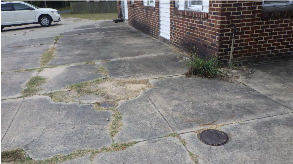
UST fill port with cover
