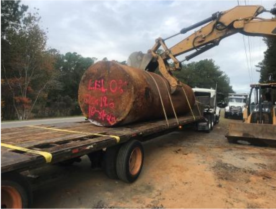
Photograph 7: EVO loading UST#2 on trailer. UST was in good condition, no holes or pitting.
