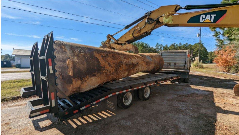
Photograph 3: Loading USTs on trailer.
