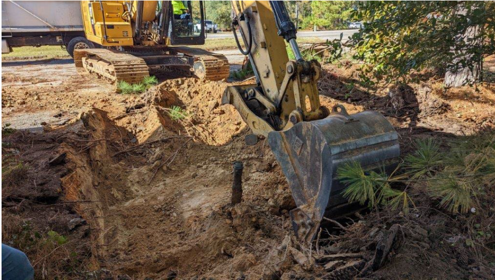
Photograph 1: Exposing top of USTs.
