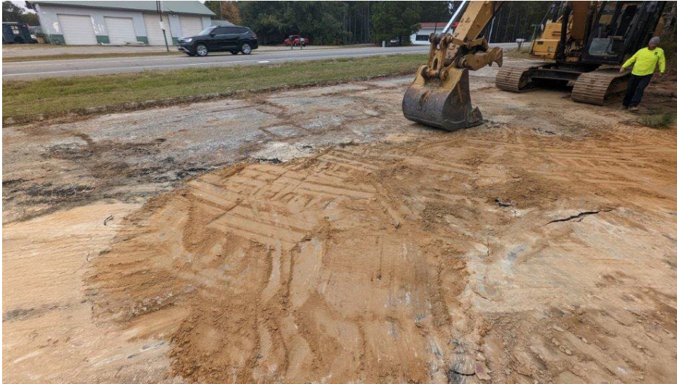
Photograph 7: Former dispenser island area after backfilling excavation.
