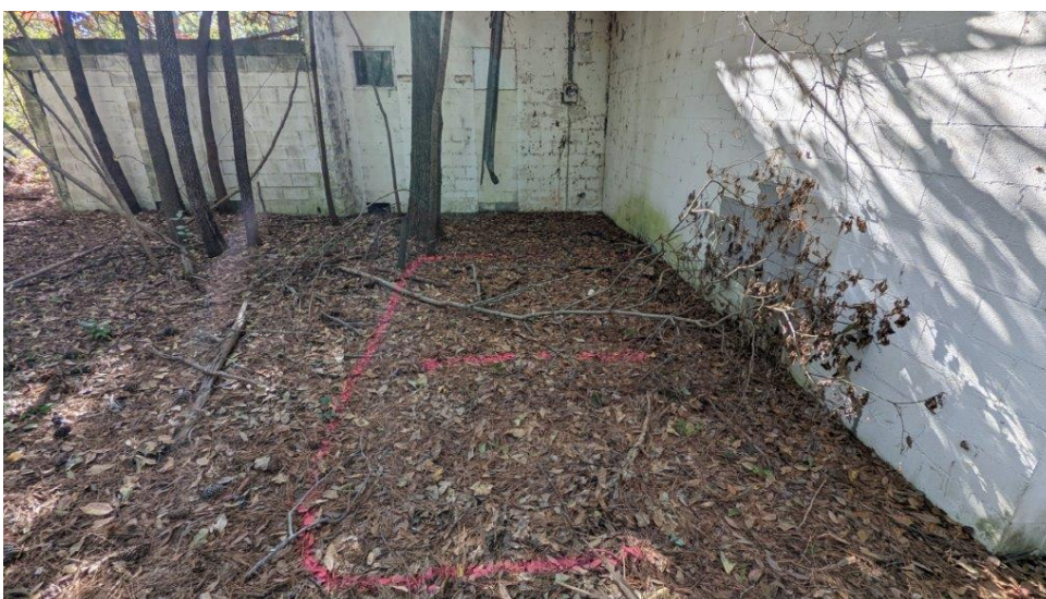
Photograph 4: TWT personnel identified an anomaly behind the existing structure.
