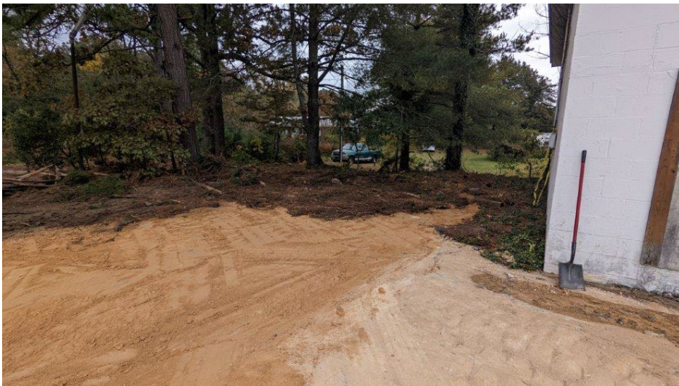
Photograph 8: Former UST area after backfilling excavation.
