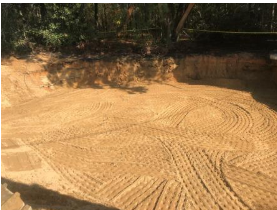
Photograph 10: Open excavation, awaiting compaction testing.
