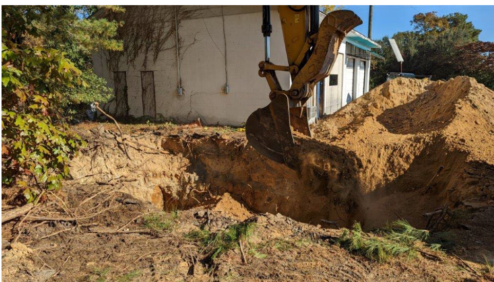
Photograph 6: Backfilling UST excavation.
