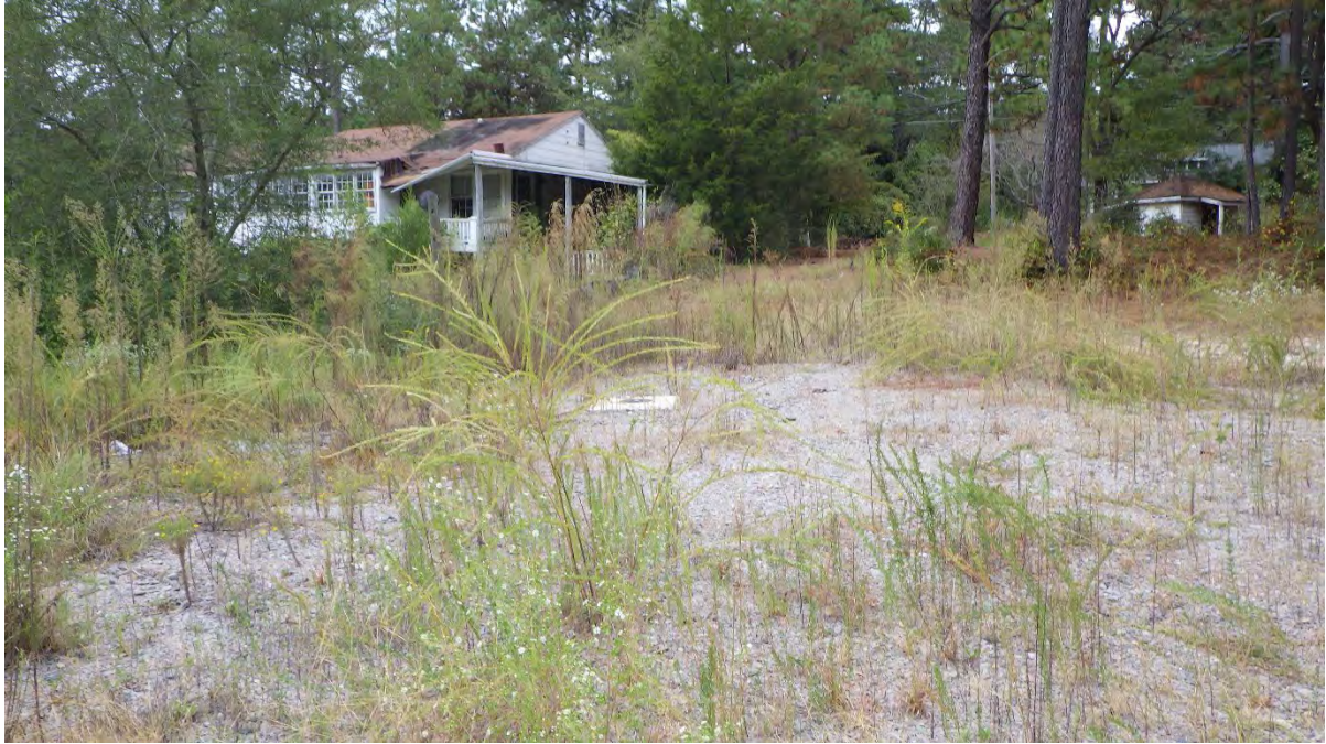
UST removal area.
