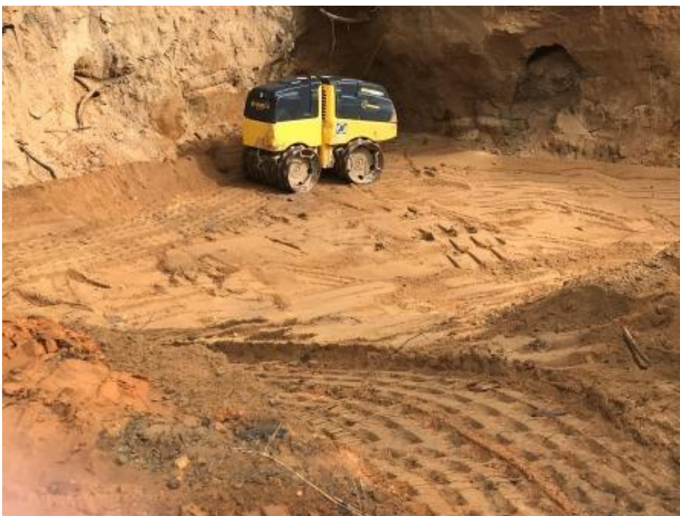
Photograph 9: EVO compacting excavation with remote compactor.
