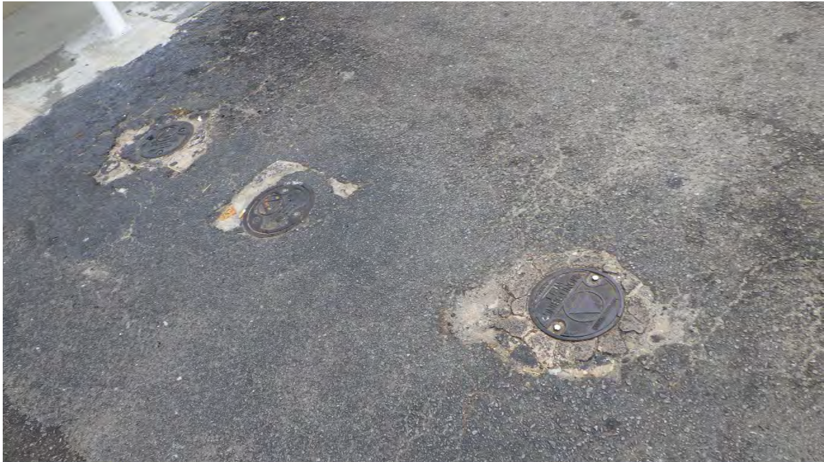
Multiple monitoring wells
