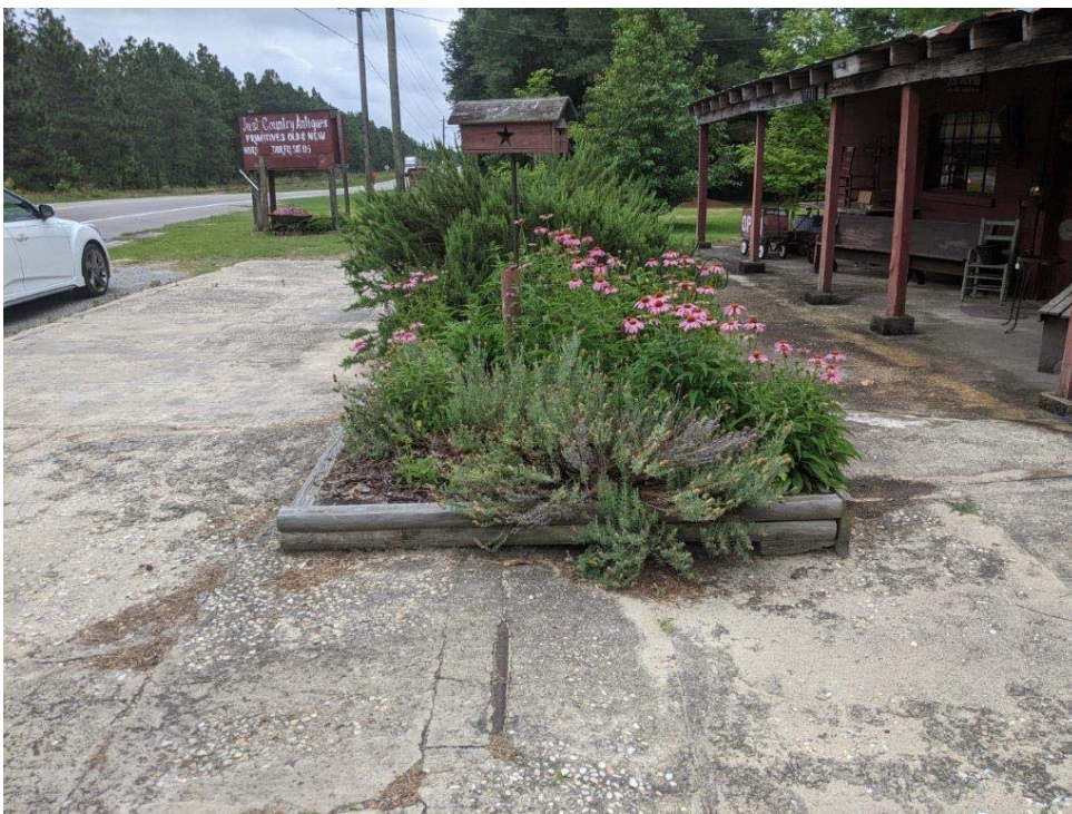
Photograph 2: View of suspected dispenser island (beneath flower beds) and possible product line (bottom of photo), facing southeast.
