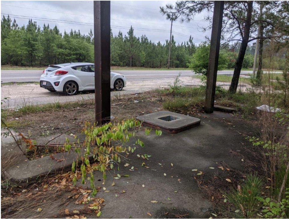
Photograph 3: Suspected dispenser islands at parcel 285, facing southeast.
