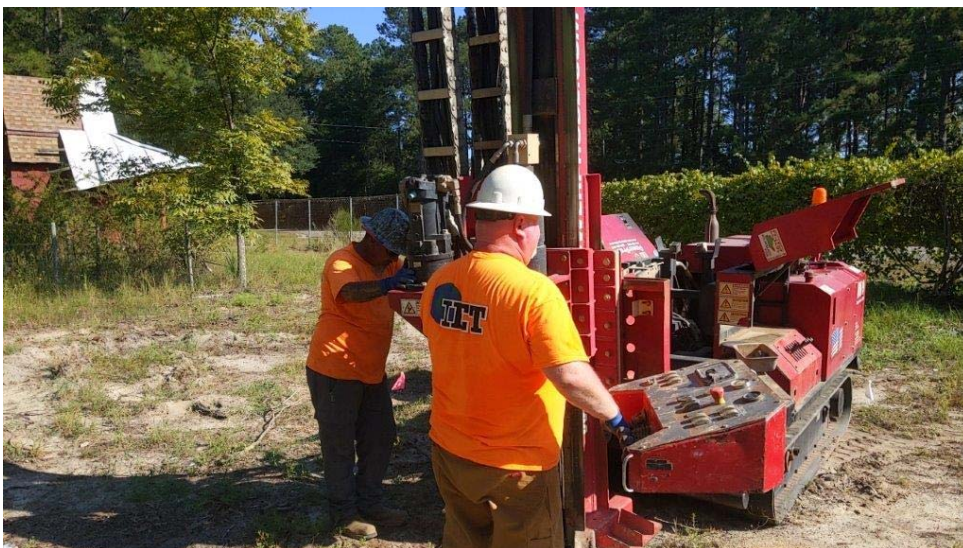
Photograph 6: View of IET advancing direct push soil sampler at parcel 335.
