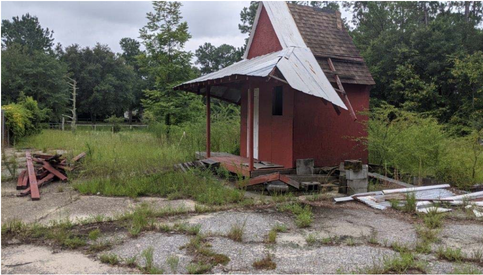
Photograph 1: Building located at parcel 335, facing southwest.
