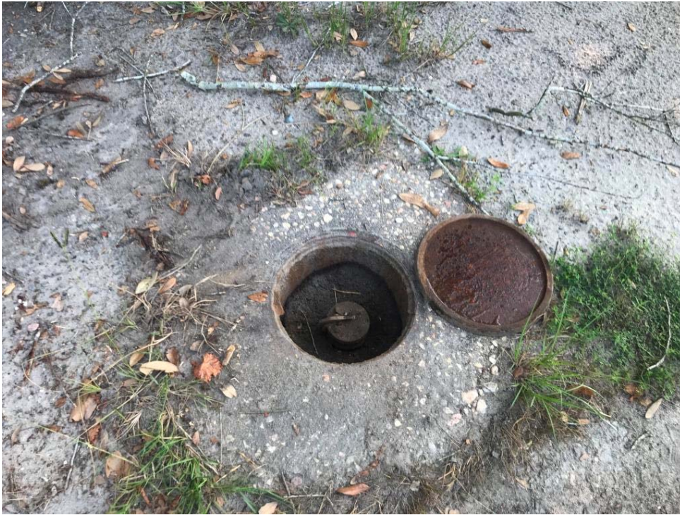
Photograph 3: Possible UST fill port located near the western building corner at parcel 368.
