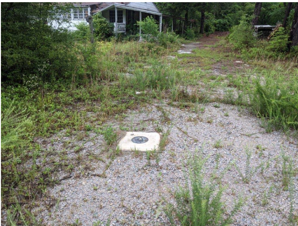
Photograph 6: MW-1 located in the southwestern portion of parcel 123, facing north.
