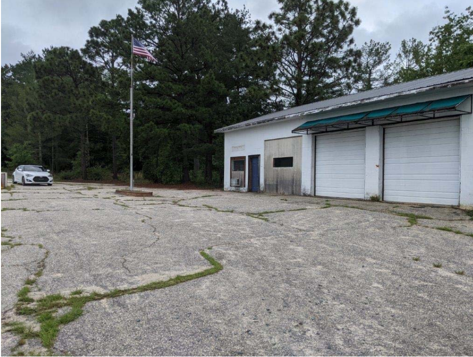
Photograph 1: View of building and suspected dispenser island at parcel 217, looking north.
