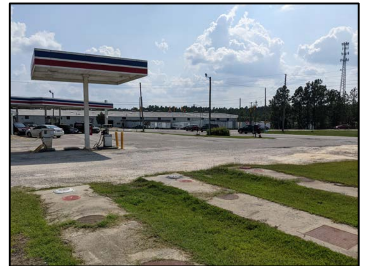
View of Survey Area (Facing Approximately South)
