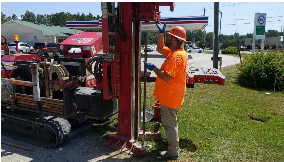
Photograph 6: View of IET advancing direct push soil sampler at parcel 229.
