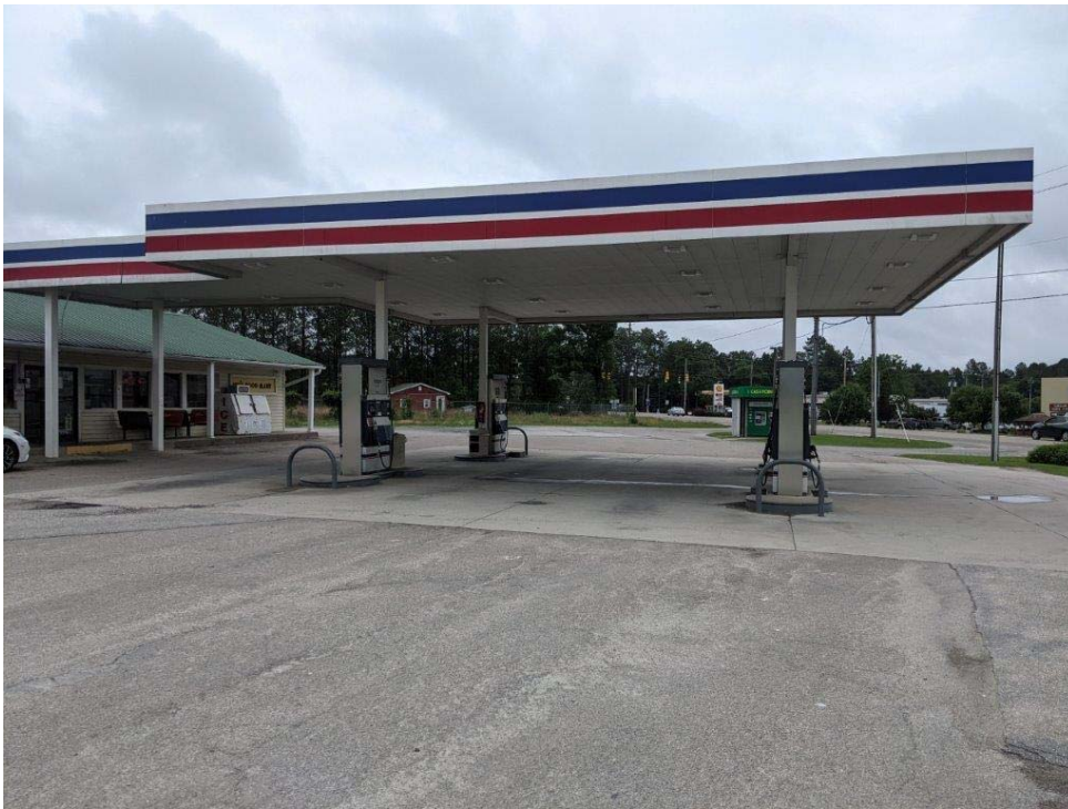
Photograph 2: View of four fuel dispenser islands located within the investigation area at parcel 229, facing southeast
