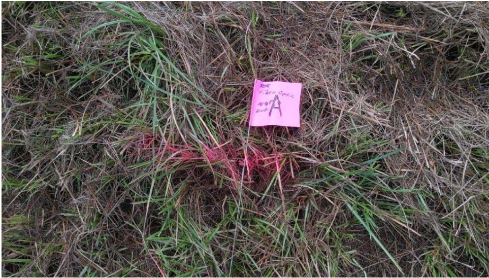
Photograph 7: Location of P218-A and paint marking indicating buried utility (fiber optic line) beneath flag location.
