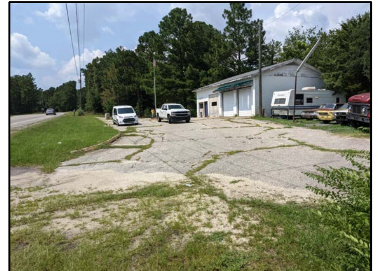
View of Survey Area (Facing Approximately Northwest)
