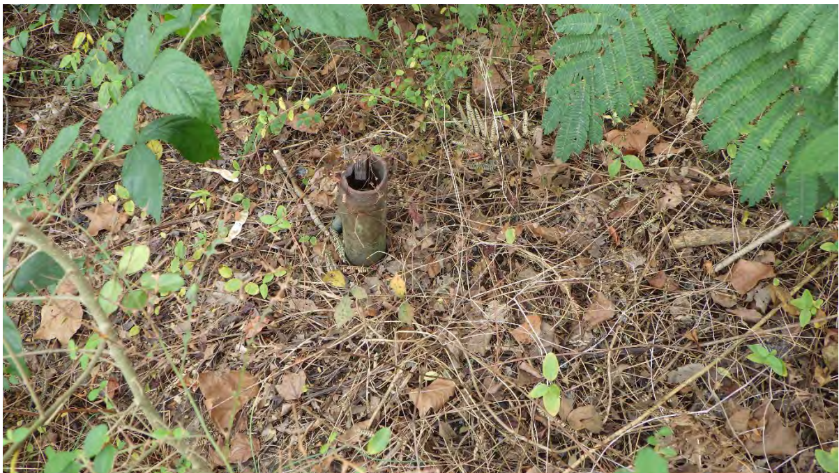
UST features in the dispenser island area-product line
