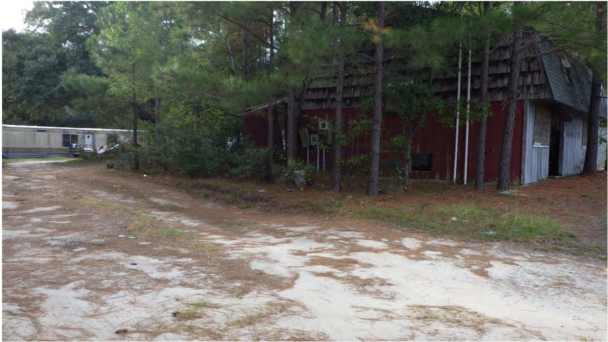
Side of the store building
