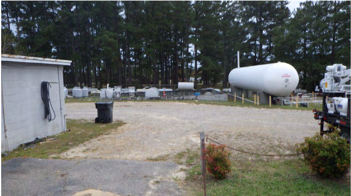
Facility yard in the back of the store building
