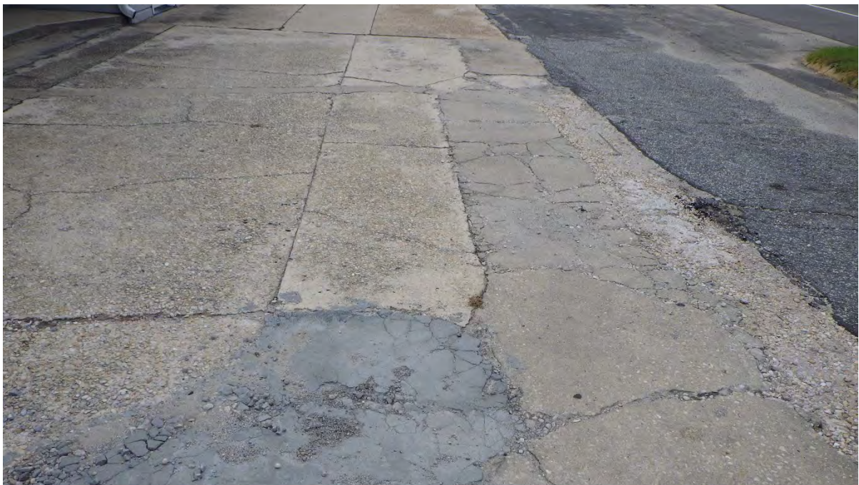
Possible former disperser island location in front of the store building
