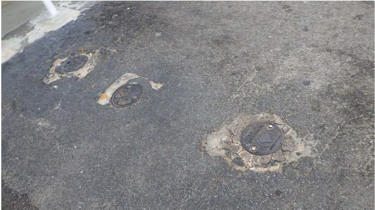
Multiple monitoring wells
