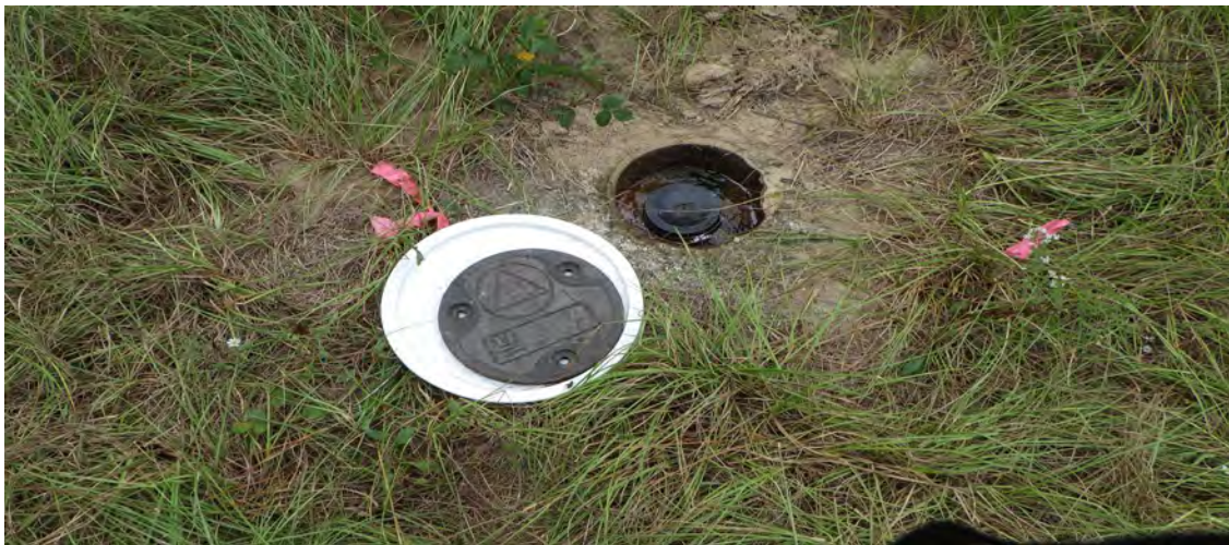
Recently accessed off site monitoring well
