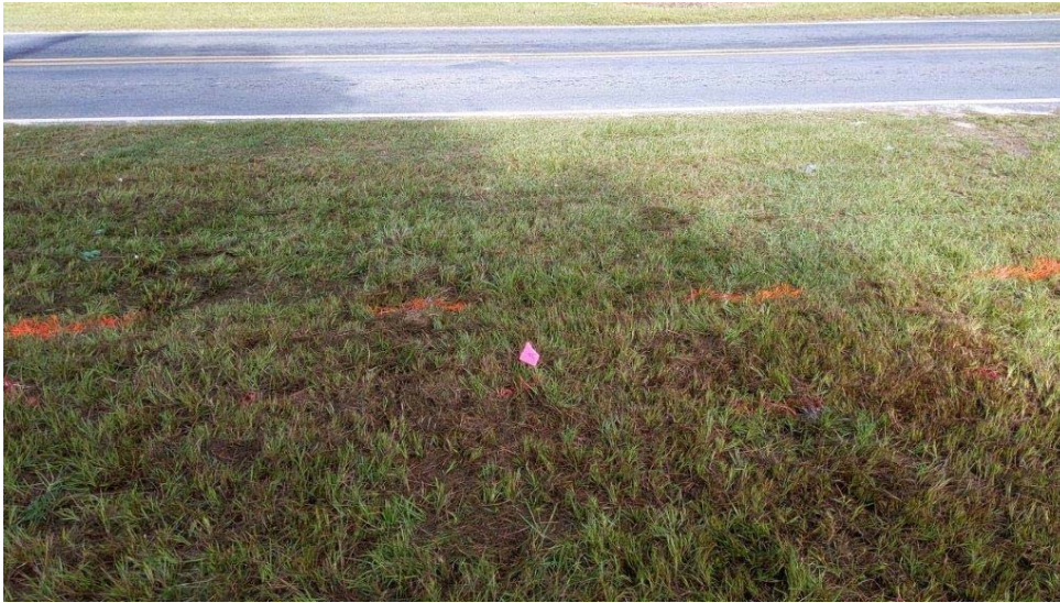
Photograph 5: Location of P218-A and paint markings indicating buried utilities (fiber optic lines), facing northwest.
