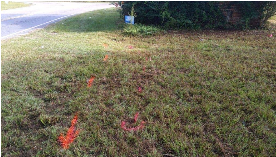
Photograph 6: Location of P218-A and paint markings indicating buried utilities (fiber optic lines), facing northeast.
