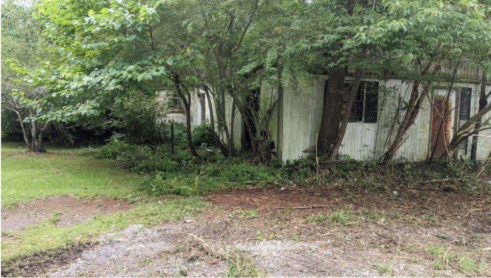
Photograph 3: Parcel 79 following the completion of vegetation clearing, facing south.
