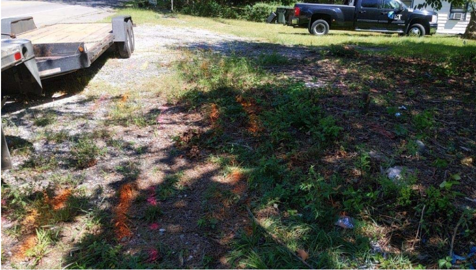
Photograph 5: View of numerous markings indicating underground utilities located between the suspected dispenser island (right side of photo) and NC 211 Hwy (left side of photo), facing east.
