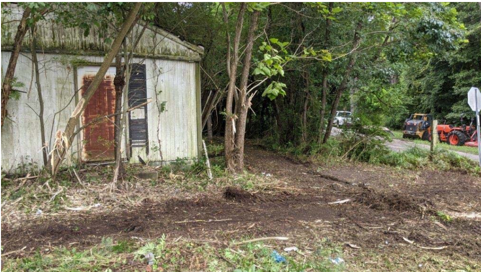
Photograph 4: Parcel 79 following the completion of vegetation clearing, facing south.
