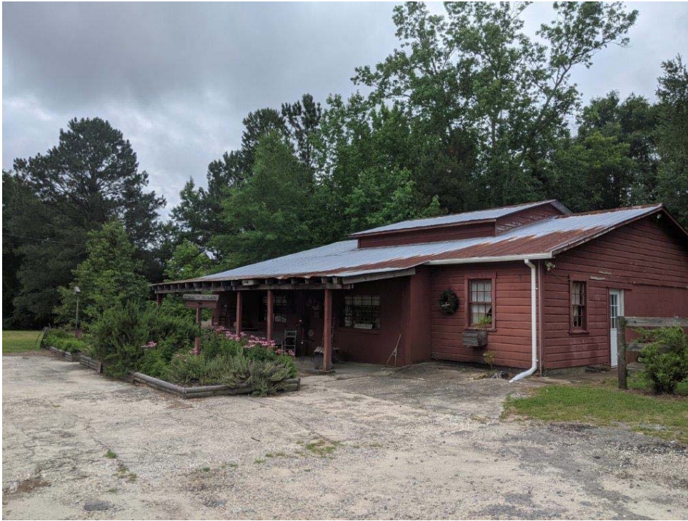
Photograph 1: View of antique store and suspected dispenser island (beneath flower beds), facing south.
