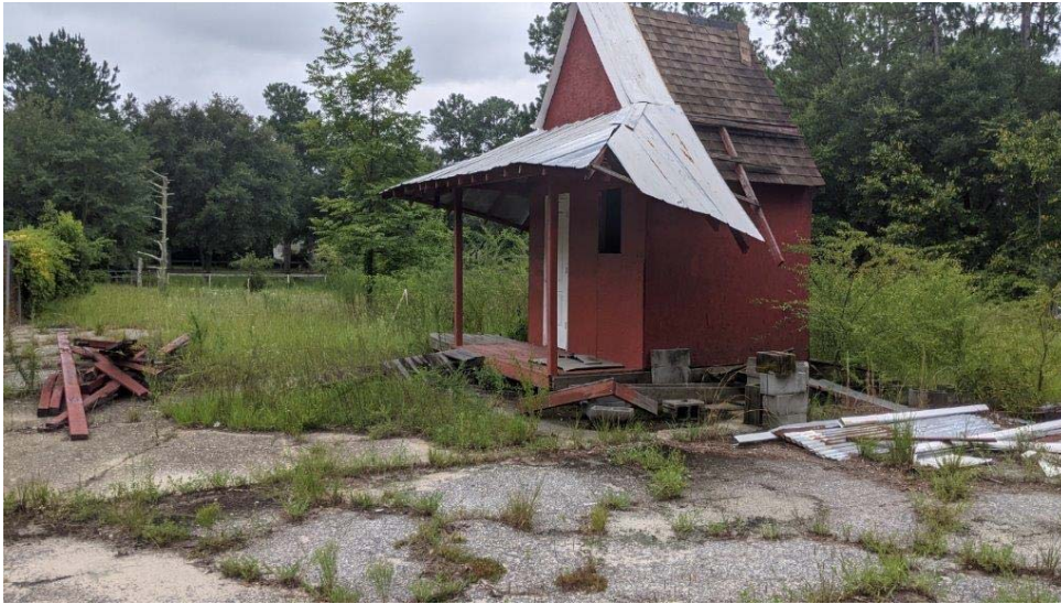
Photograph 1: Building located at parcel 335, facing southwest.
