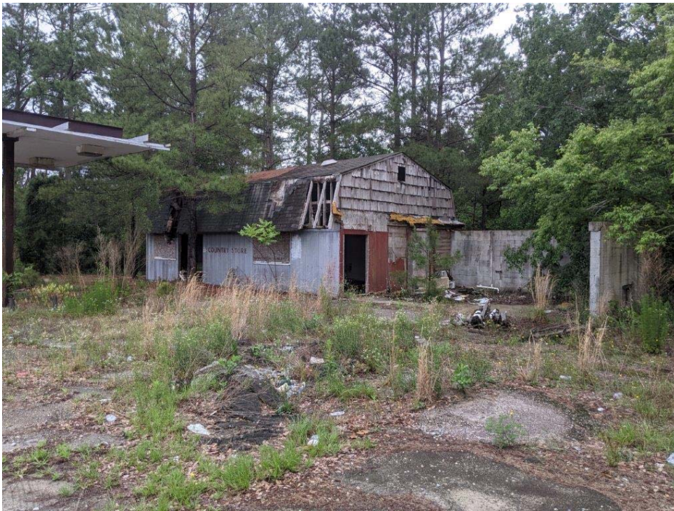
Photograph 2: Building and canopy at parcel 285, facing southwest.
