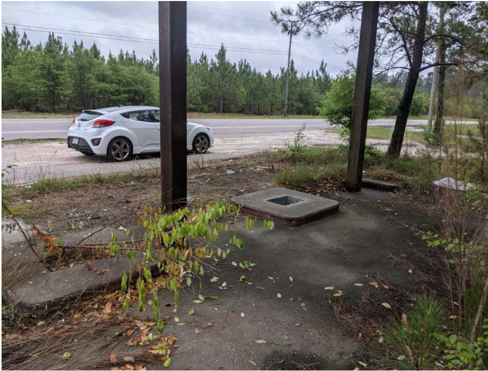
Photograph 3: Suspected dispenser islands at parcel 285, facing southeast.
