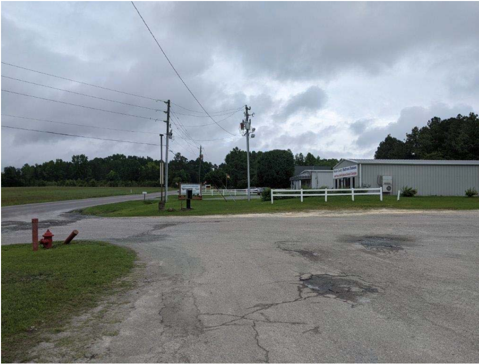
Photograph 3: Northern portion of investigation area at parcel 229, facing north.
