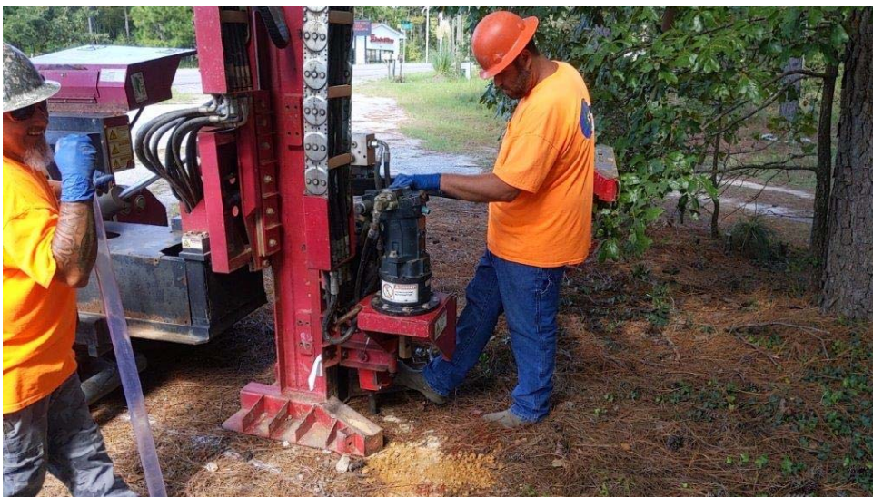
Photograph 4: View of IET advancing direct push soil sampler at parcel 217.
