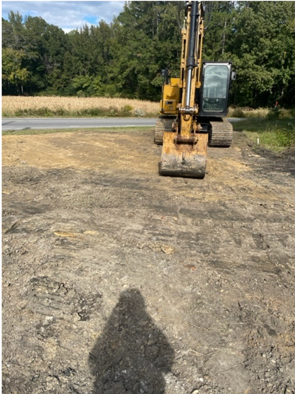
Photograph 14: Excavation filled, brought back to grade, and compacted with excavator.
