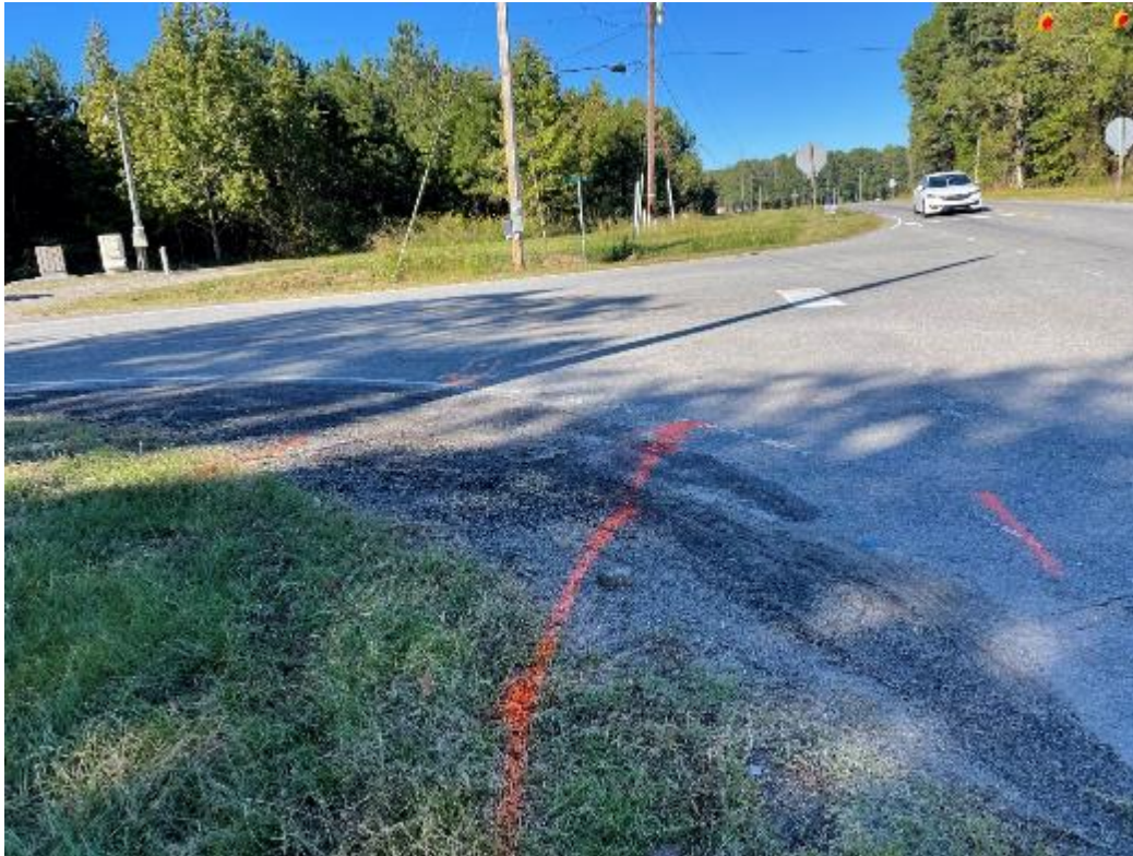
Photograph 5: Marked broadband utility services
