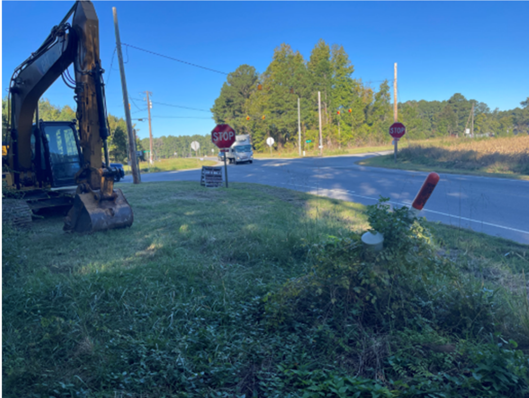
Photograph 1: View of site prior to closure activities.
