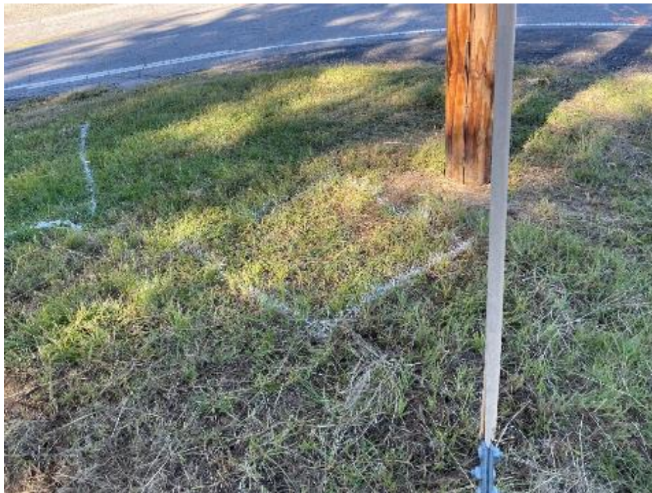
Photograph 4: Anomaly area identified with GPR adjacent to corner pole.
