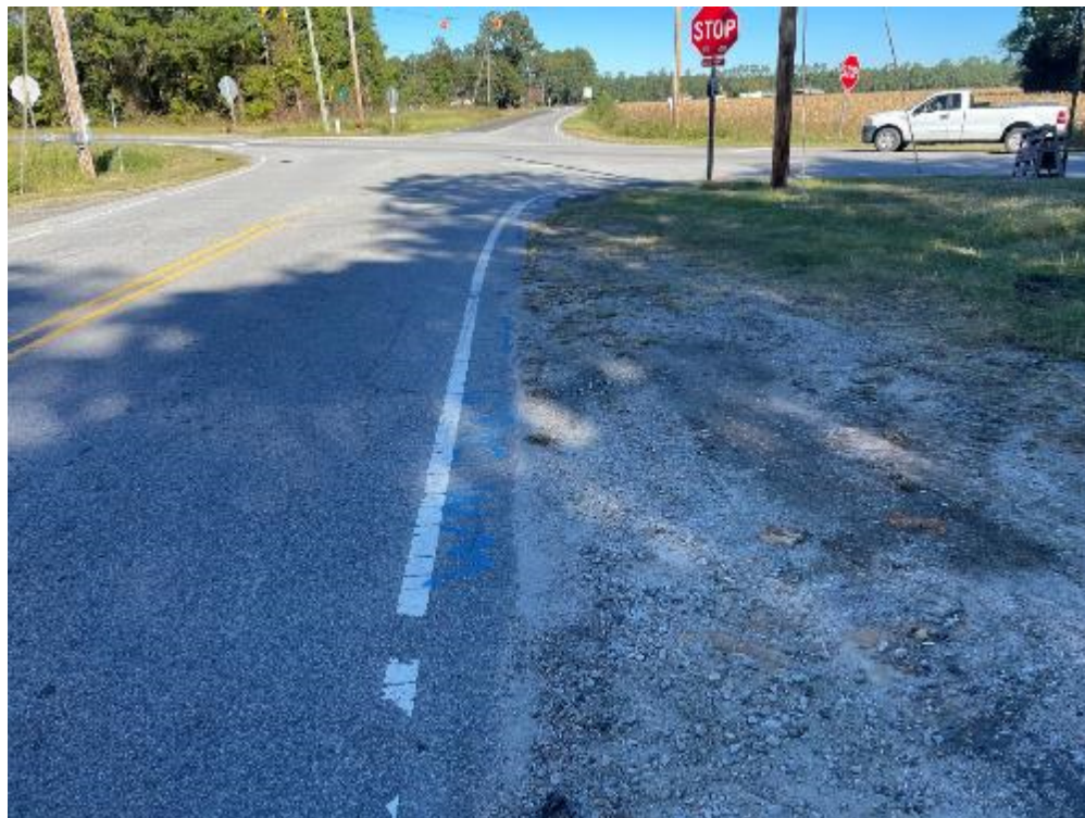
Photograph 6: Marked water services.
