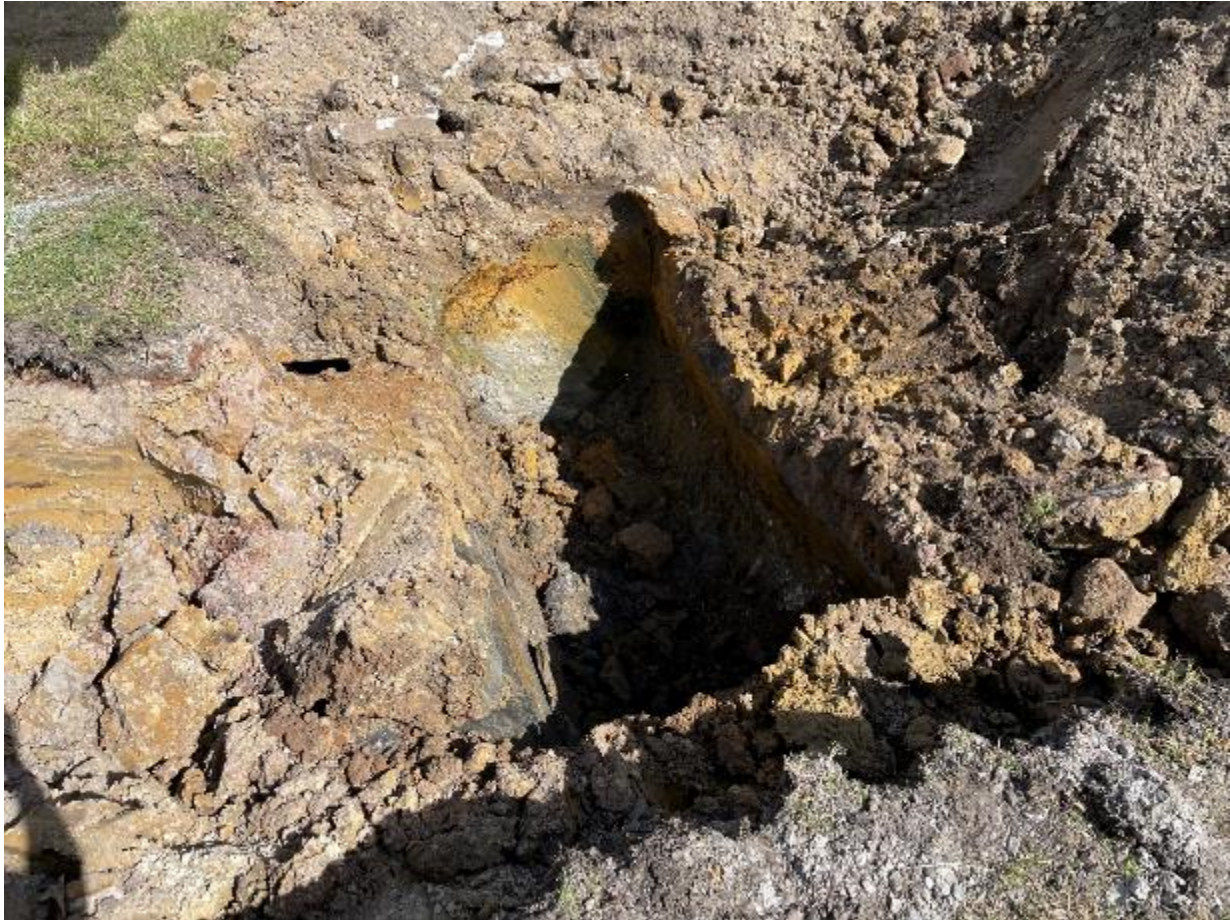
Photograph 9: Tank pit 1 post-tank excavation.
