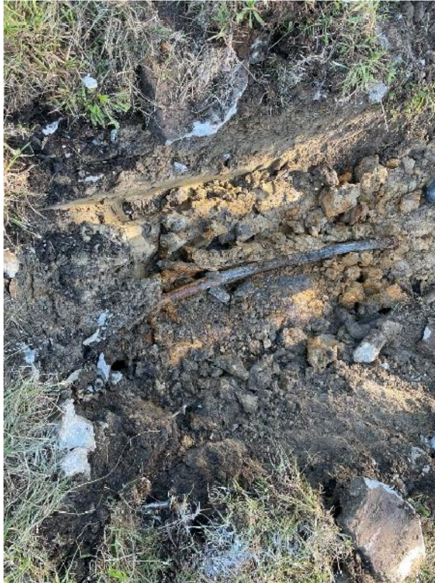
Photograph 7: Tank 1 excavation pit, showing single pipe from tank
