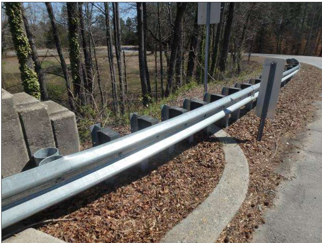
Northeast Corner Transition
