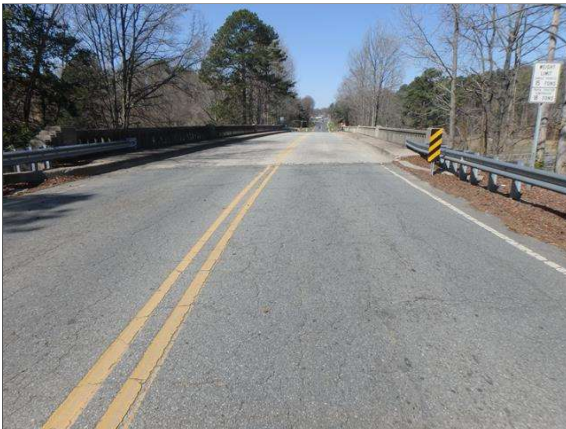
East Approach Looking West
