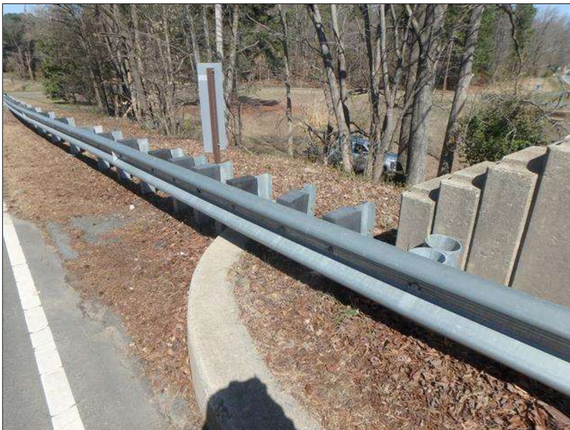
Northwest Corner Transition
