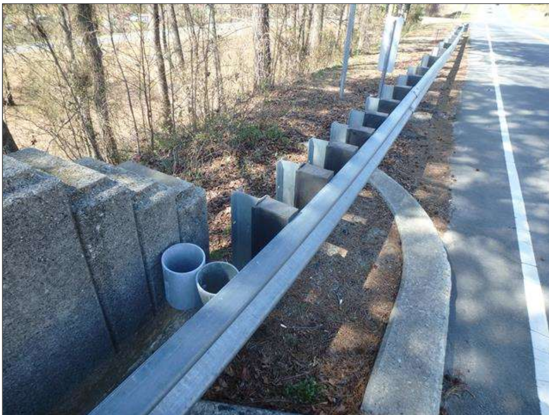
Southwest Corner Transition
