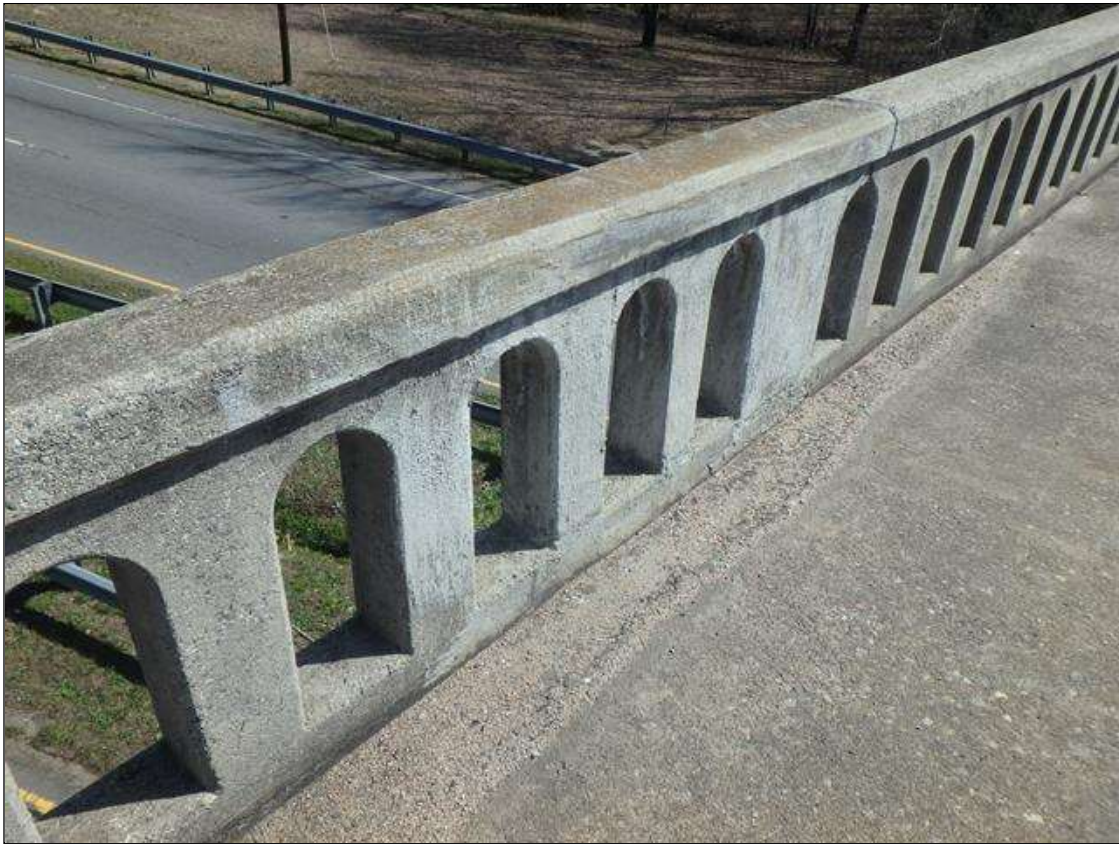
Span 2 left RC rail near mid-Span, sound repair.
