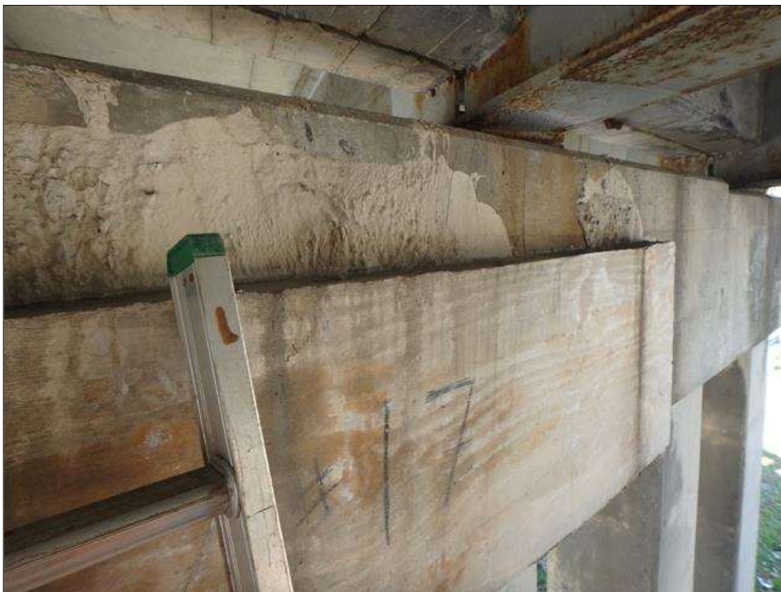
Bent 2 cap East side below bay 2, sound patch.
