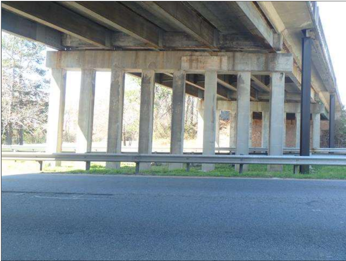
Bent 2 east side
