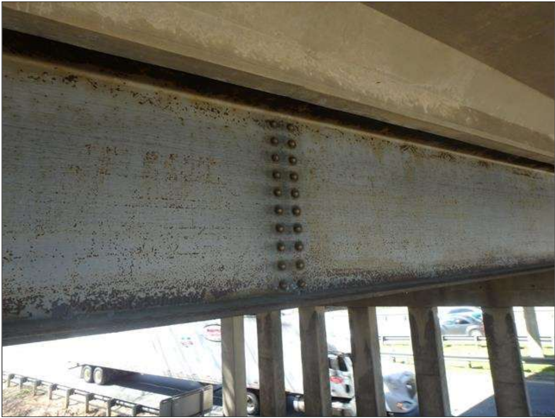
Span 4 Beam 1 left side, Interior Diaphragm riveted connection.
