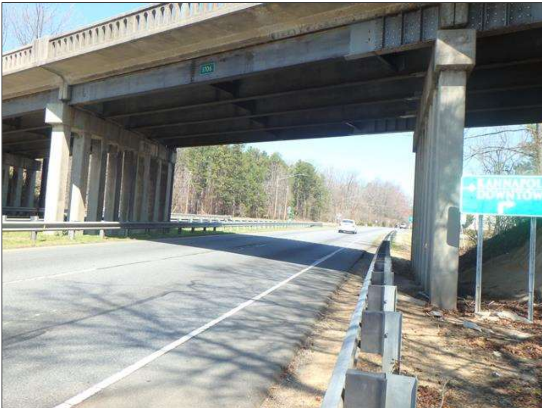
Looking North Span 3
