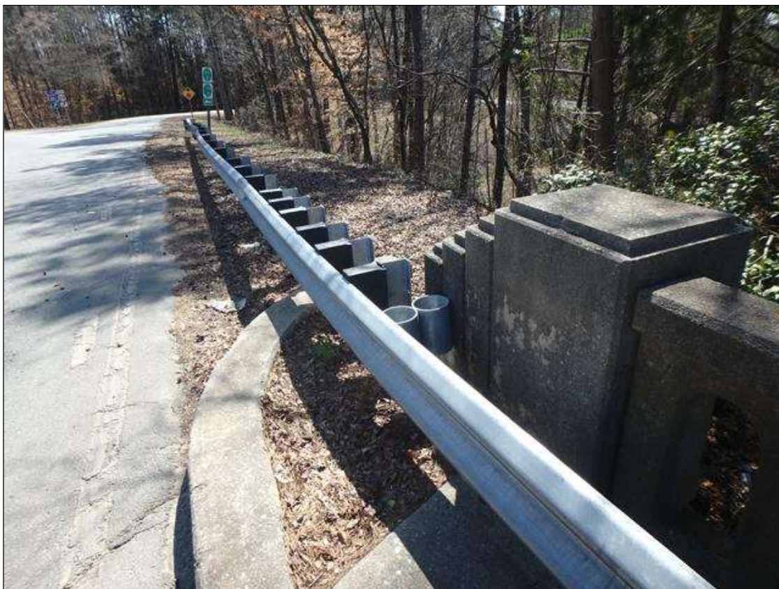
Southeast Corner Transition
