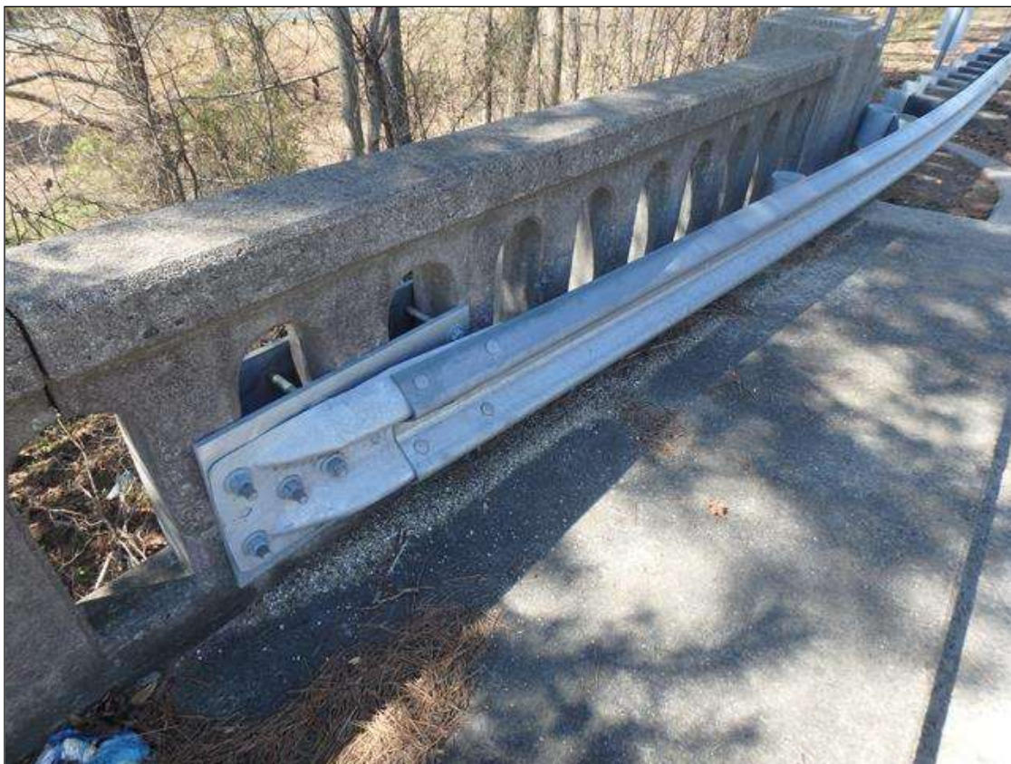
Guardrail connection at Southwest Corner
