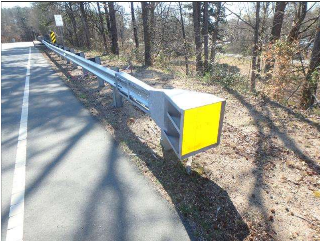
Guardrail end Southwest Corner
