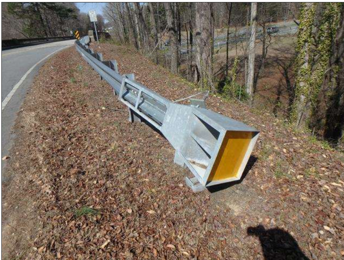
PRIORITY MAINTENANCE: Guardrail end treatment at Northeast Corner has impact damage: cable disconnected, end treatment pushed and leaning over 1'.
