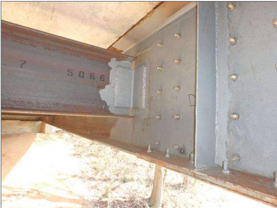
Span 4 intermediate diaphragm in bay 4 near Bent 3, welded connection to beam 5.
