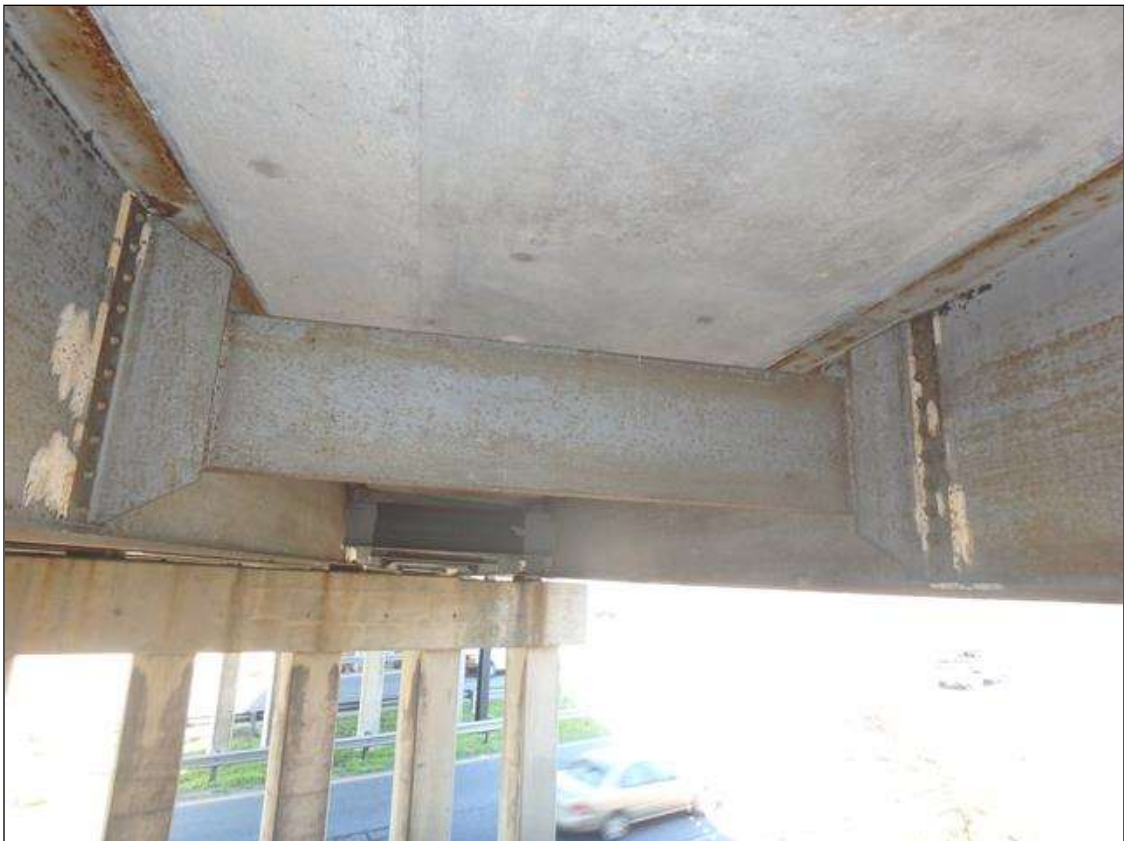
Span 4 intermediate diaphragm in bay 1
