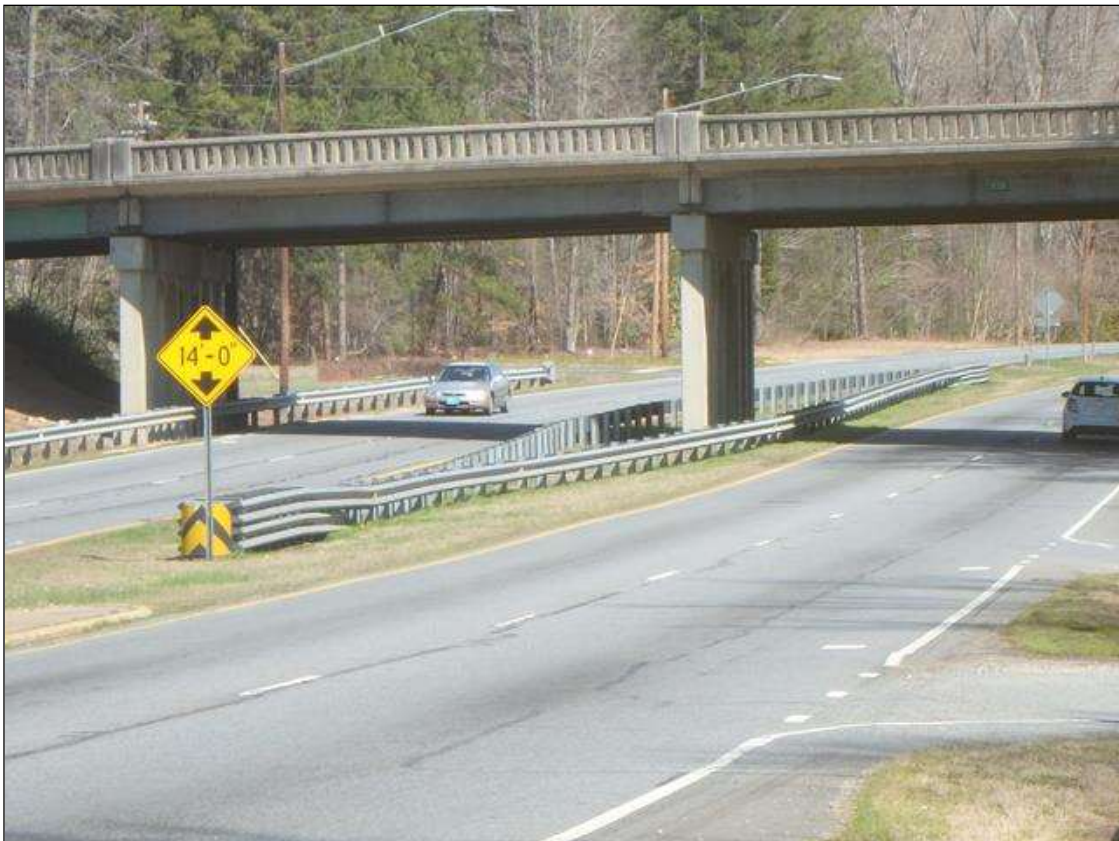
North bound US 29 vertical clearance sign at 200' south of structure
