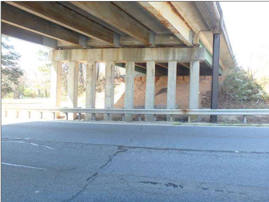
Bent 1 east side
