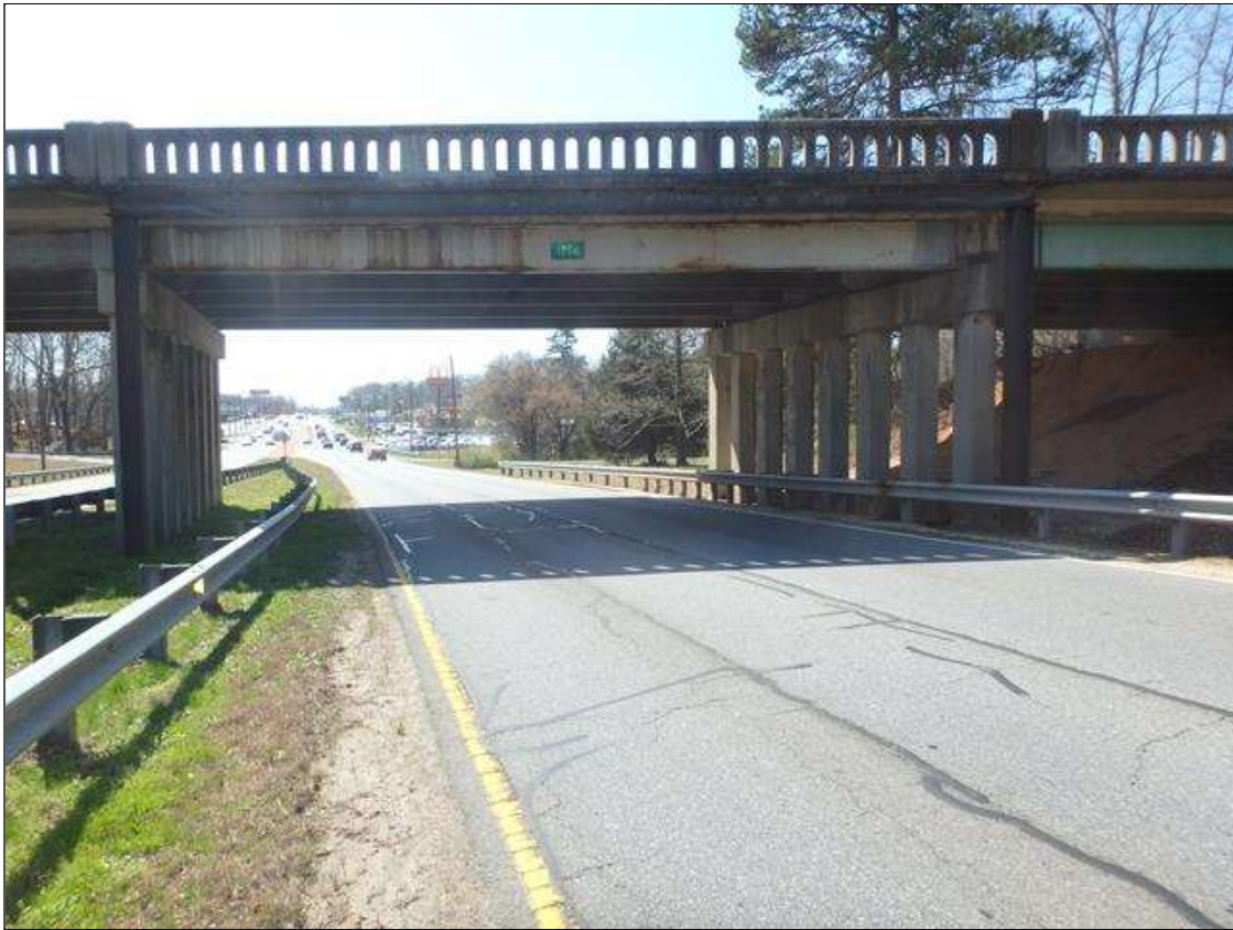
Looking South Span 2
