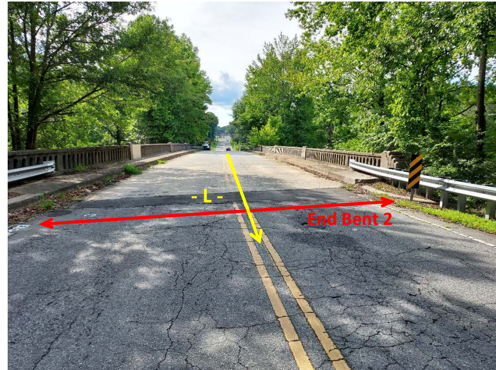
Photograph No. 3: View looking west at End Bent 2
