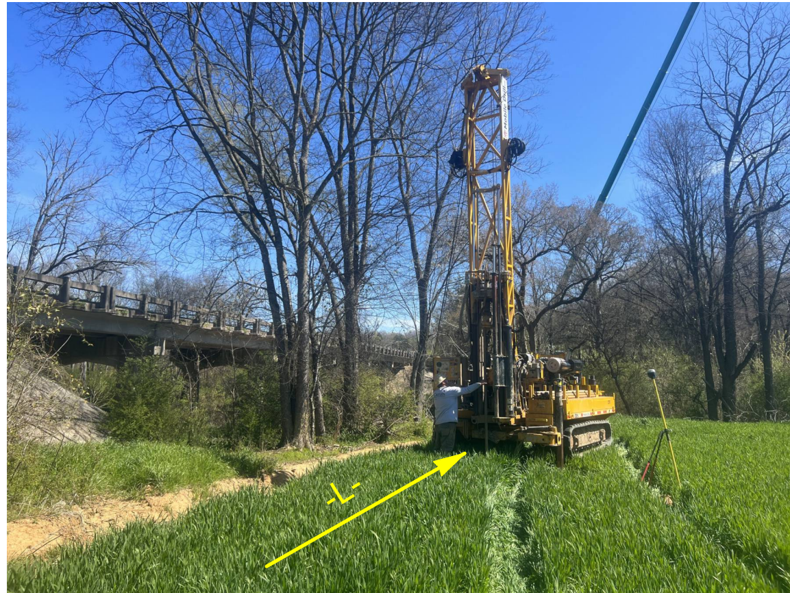
RIG ON EB1-C FACING UP STATION
