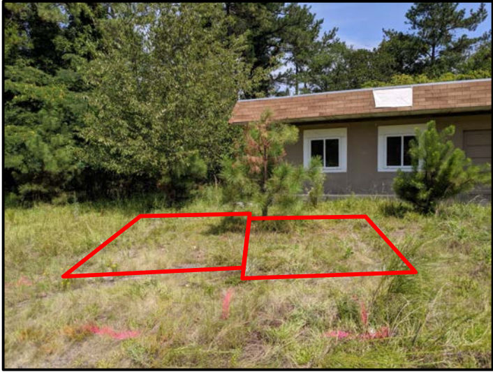
View of Two Probable USTs Facing Approximately North
